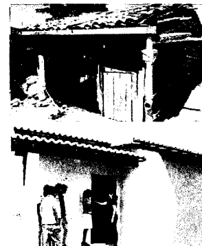
Before and after the house
