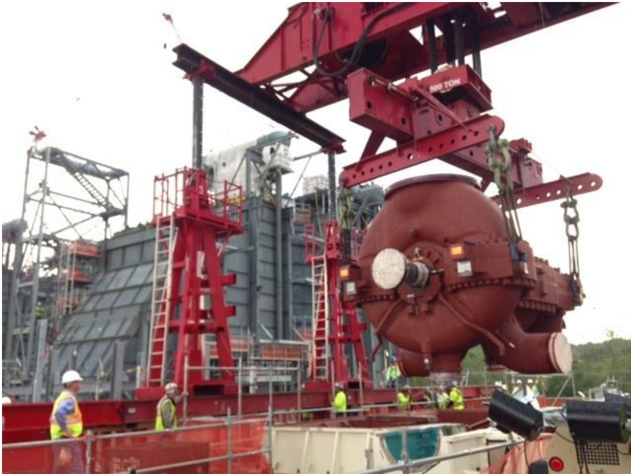
Setting High Pressure/Intermediate Pressure Turbine
