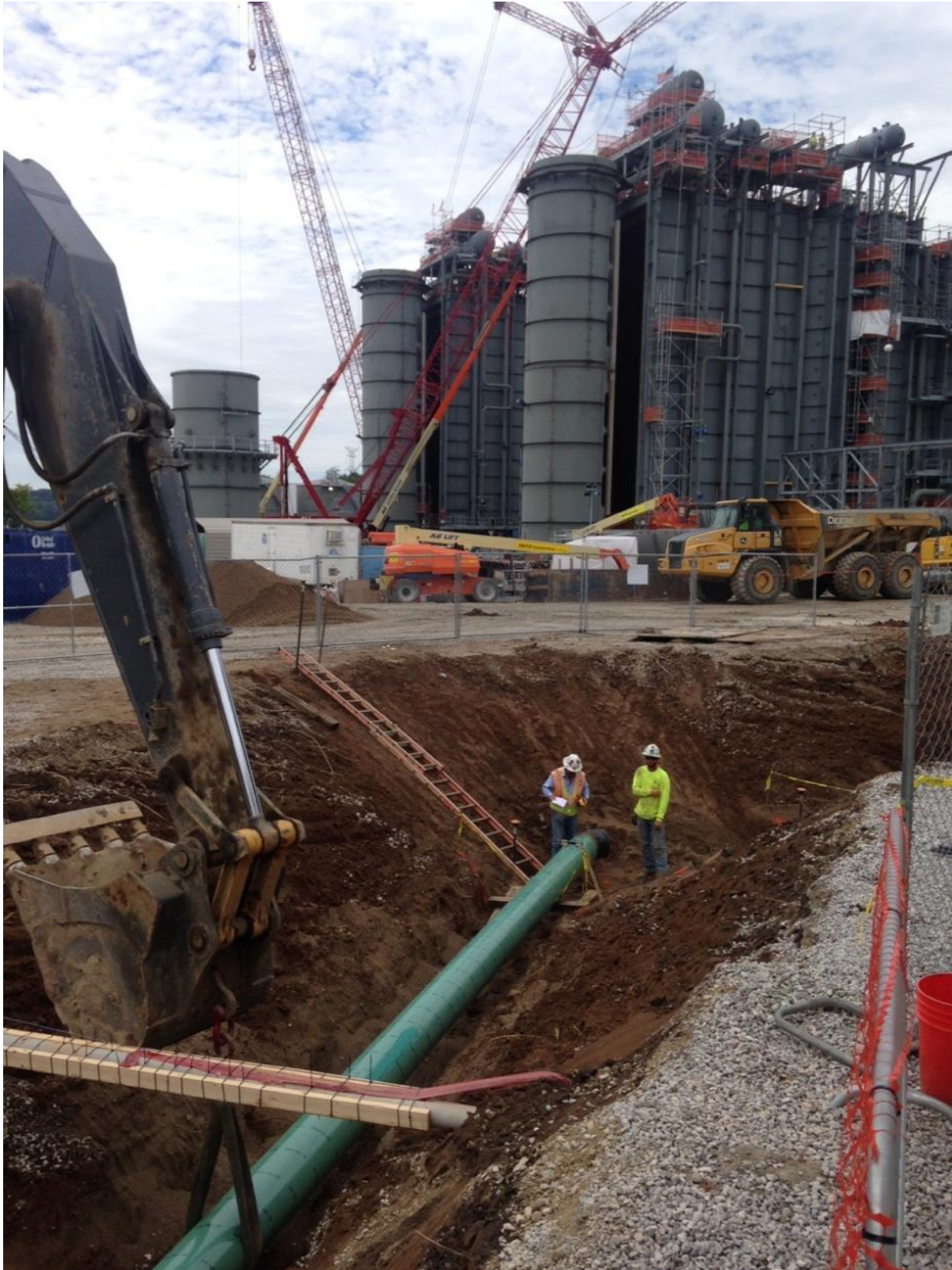
Gas Pipeline Installation on Site
