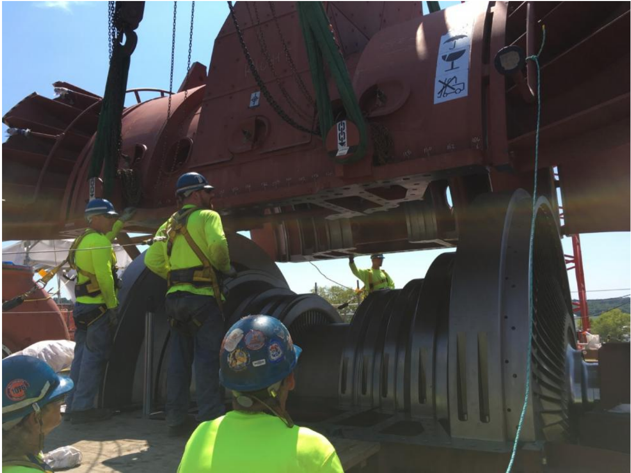
STG Inner Upper Install
