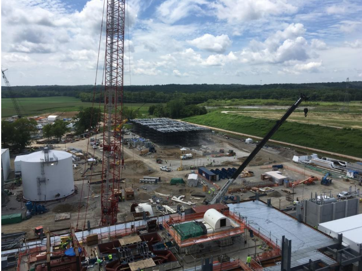
Cooling Tower Erection
