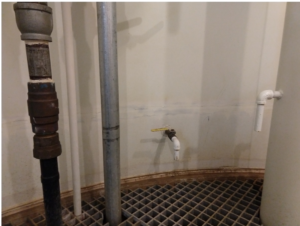
Close-up shot of Aeralater repair
