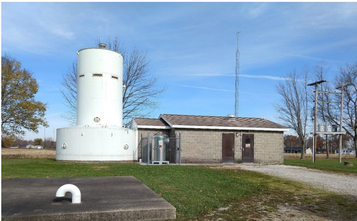
Treatment plant exterior, Aerator on left
