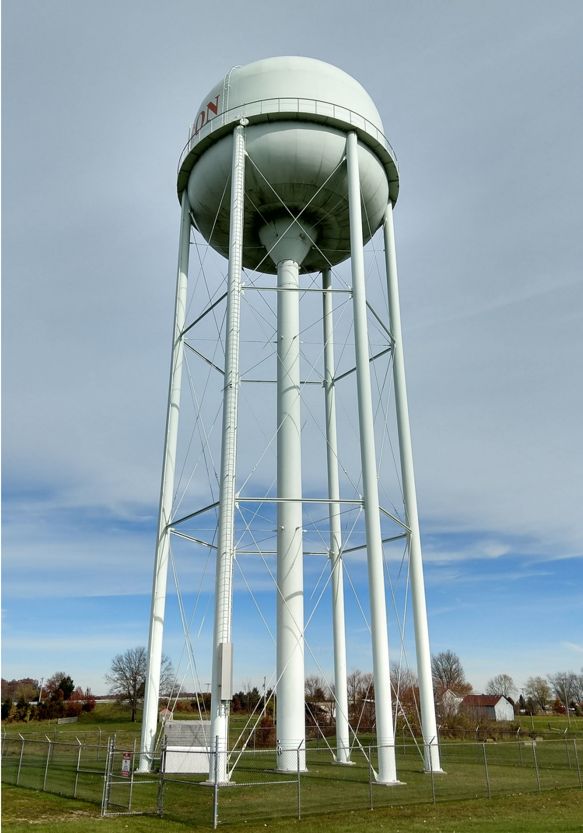
St. Leon 500,000-gallon tank
