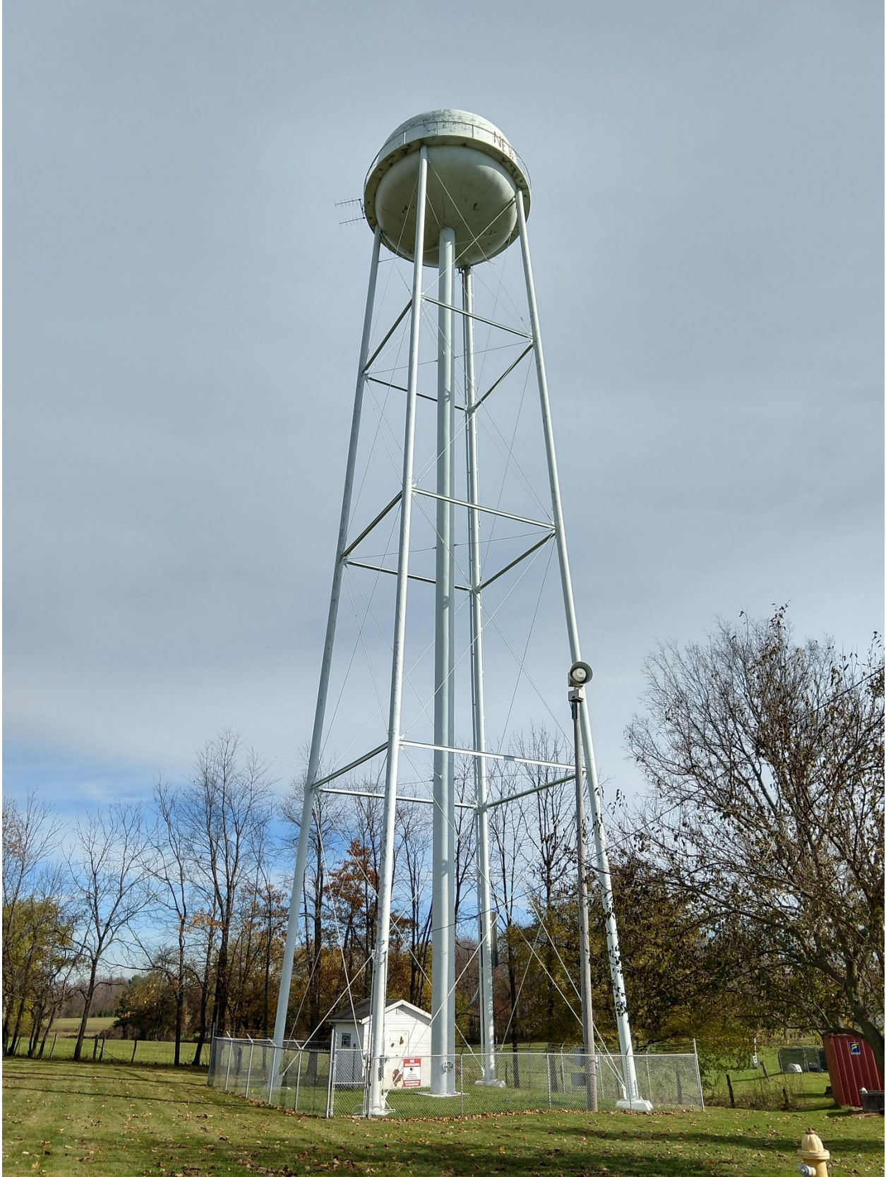
Old New Alsace 75,000-gallon tank
