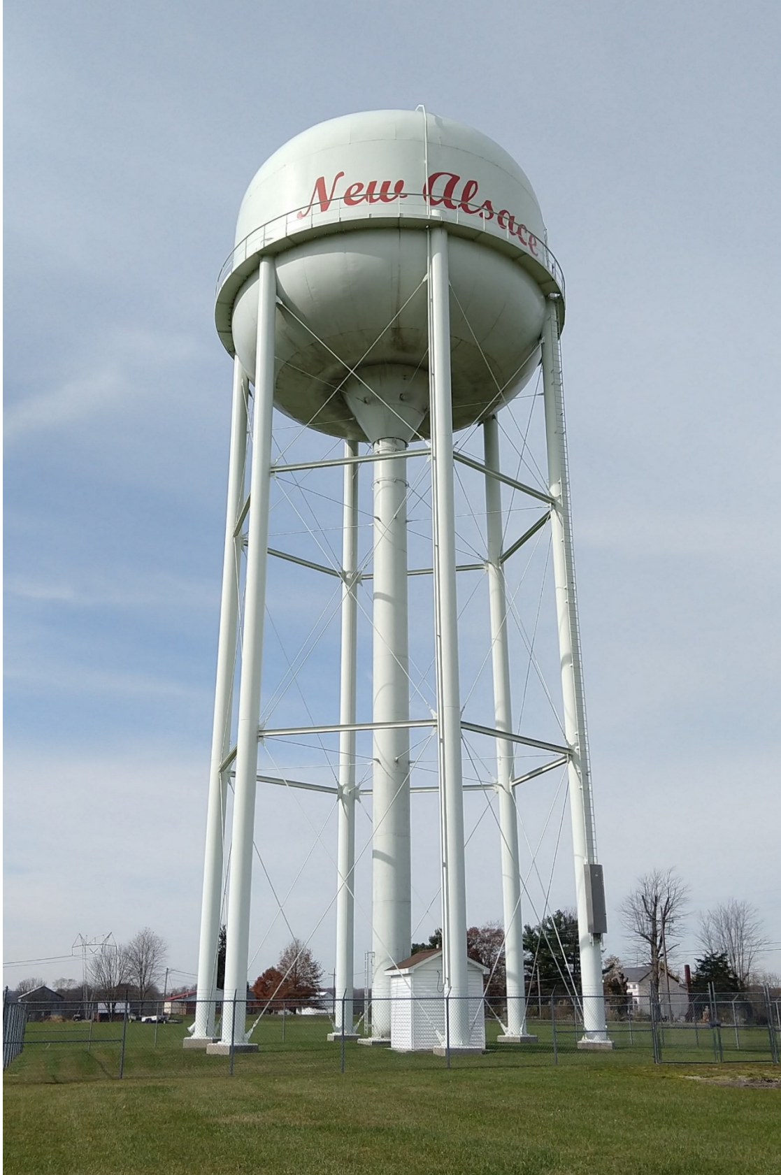
New New Alsace 500,000-gallon Tank
