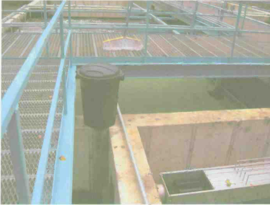
North Clarifier (note duckweed on surface)
