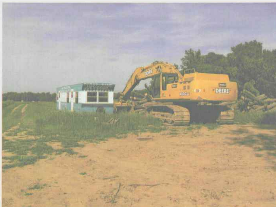
On site equipment and trailer
