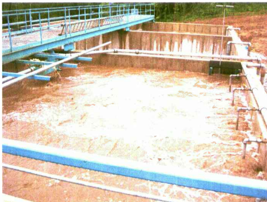
South aeration basin
