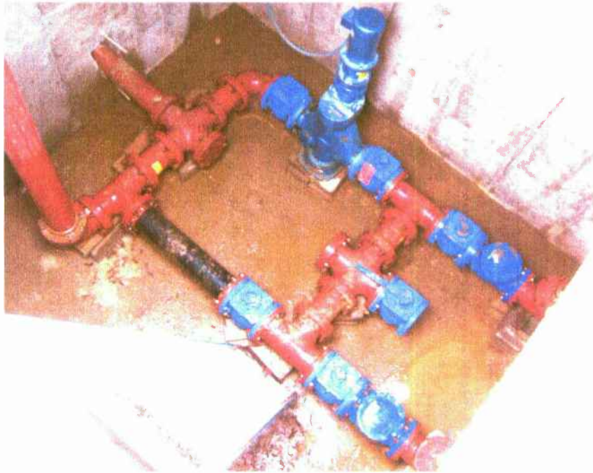
Influent dry well 04
