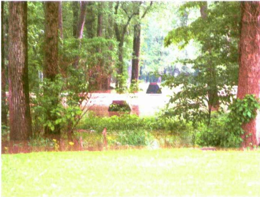
Bypass manhole. No bypassing at inspection 11
