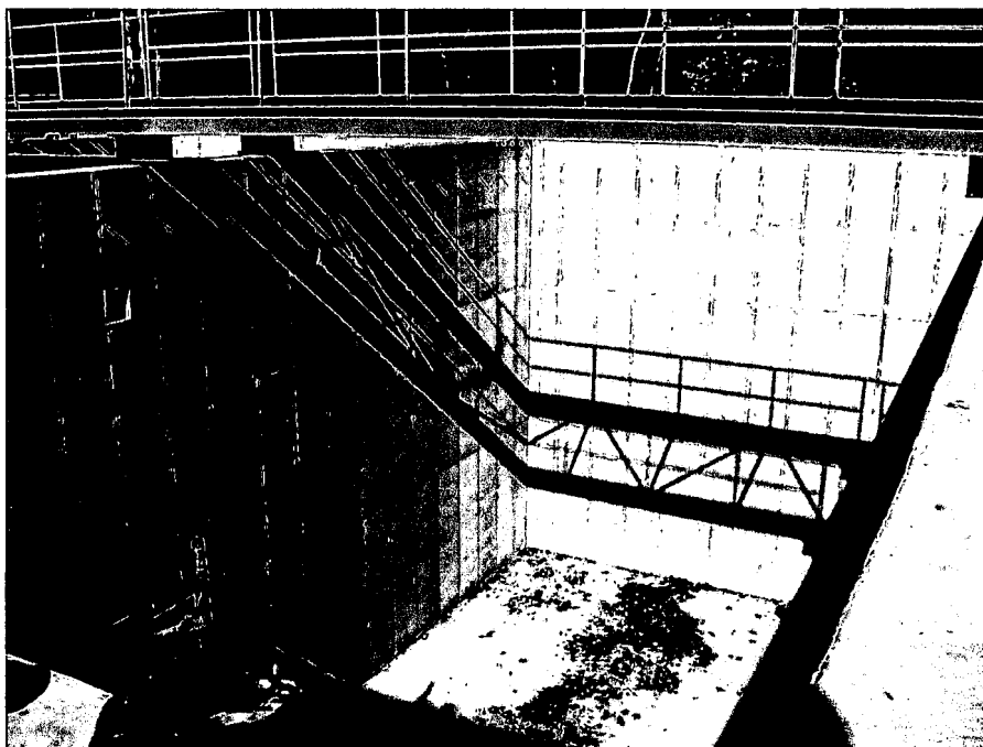
Aeration tank - 24 foot deep
