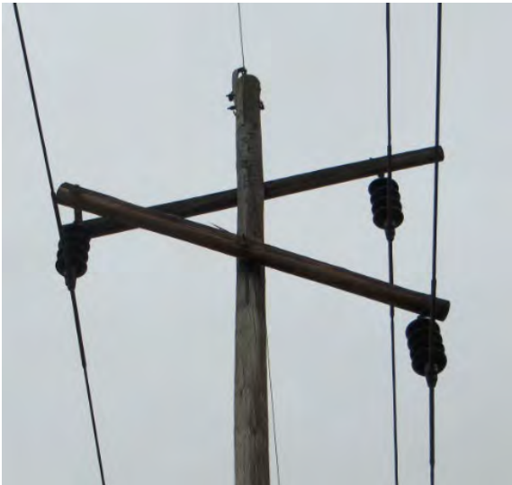
Wishbone Construction
