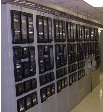
Typical Electromechanical Relays
