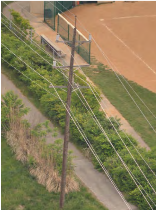
69 kV Wood Pole Construction
