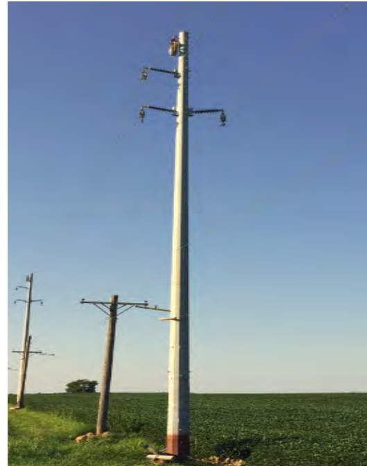
New 69 kV Steel Pole Construction
