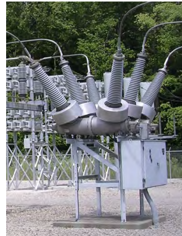
Typical Transmission Gas Circuit Breaker
