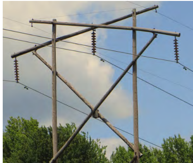
Gulf Port Construction
