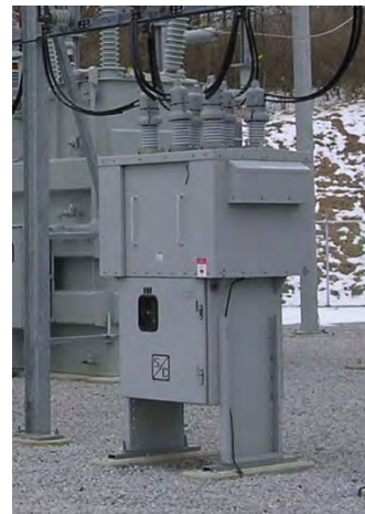
Typical Distribution Vacuum Circuit Breaker
