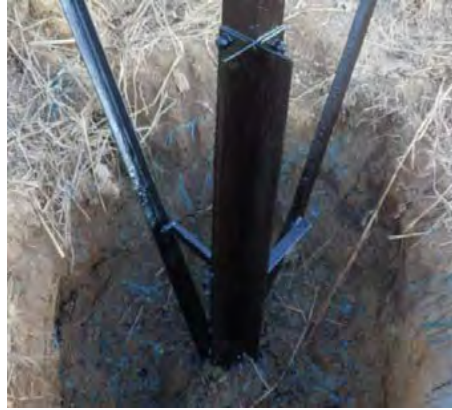
Tower Leg Repair
