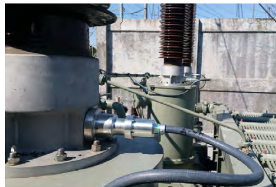
Typical Transformer Bushing Monitor Sensors
