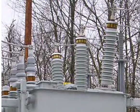
Transformer Bushings
