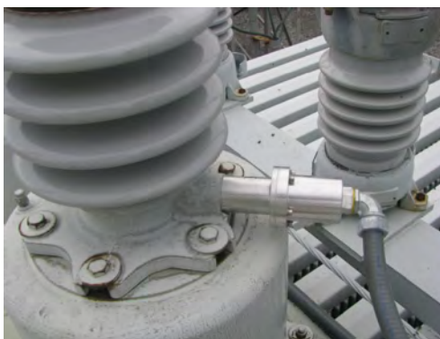
Typical Transformer Bushing Monitor Sensors
