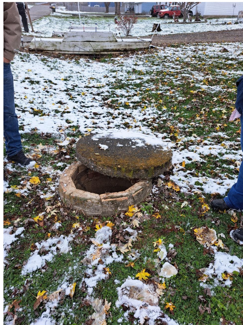
Fig. 20 – 2024 Photo - View of shallow manhole in ditch line.
