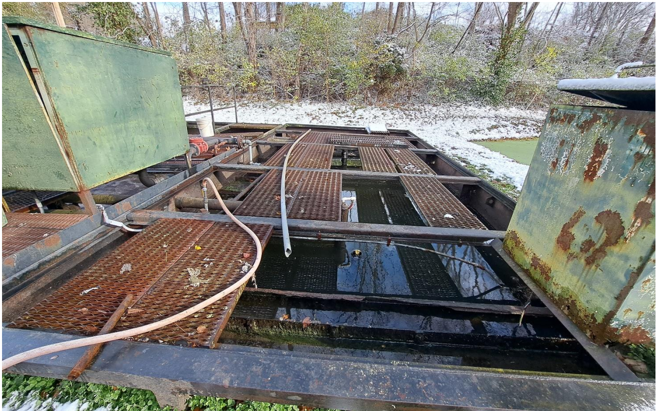
Fig. 14 – 2024 Photo – View NE of clarifiers with blowers at left.
