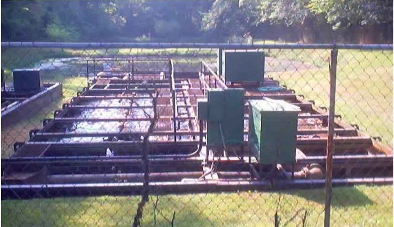
Fig. 1 – 2002 Photo. View SE of the 60,000 gpd steel package plant installed in 1974. The original 16,700 gpd. package plant is at left center. Polishing ponds are beyond.
