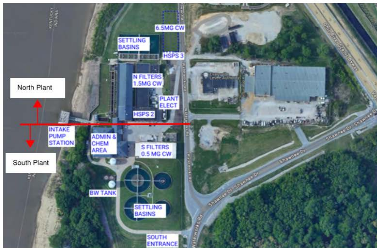
Figure 3-1: Aerial View of WTP Delineating North and South Plants
