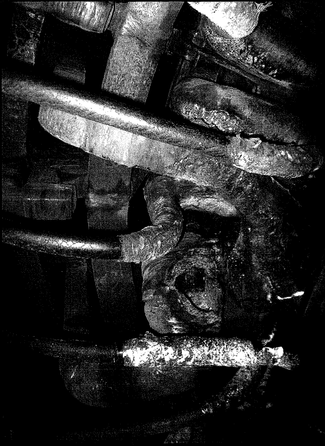
Area of Gibson failure at connections-as found condition
