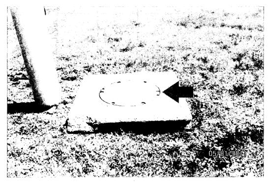
Photo shows the tank midway access manway. Manway is a street manway with direct access to the water storage area and is allowing the ingress of waterborne contaminants into the watet sysyem. AWWA regulations require a 4" minimum curb and a 2" overlap cover above the roof. We recommend installing a 4" curb with a 2" overlap cover on the street ring.
