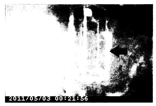
Tank end manway interior shell ladder in above photo is not equipped with non-skid rungs and is seriously deteriorated. We recommend installing an OSHA approved interior shell ladder complete with standoffs every 10' on centers and a cable type ladder safety device.
