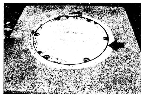
Photo shows the tank end access manway. Manway is a street manway with direct access to the water storage area and is allowing the ingress of waterborne contaminants into the watet sysyem. AWWA regulations require a 4" minimum curb and a 2" overlap cover above the roof. We recommend installing a 4" curb with a 2" overlap cover on the street ring.
