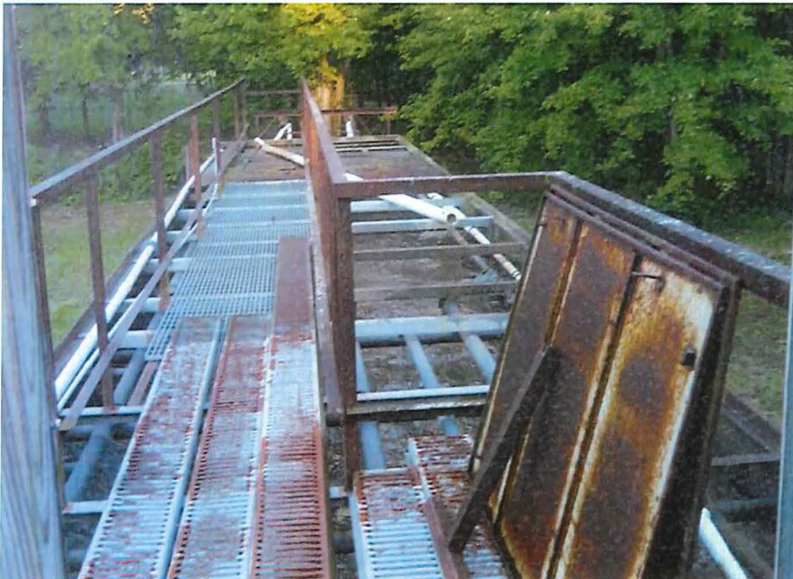
Fig. 3 View west of top of the aeration tank and sludge digester.
