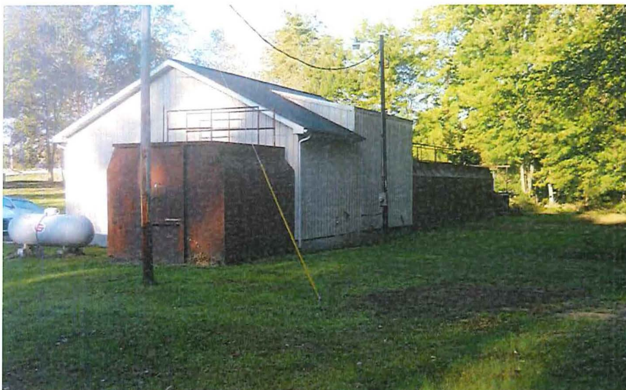
Fig. 7 View of out of service filter tank (brown), Control Building, and Aeration Tank (in background).
