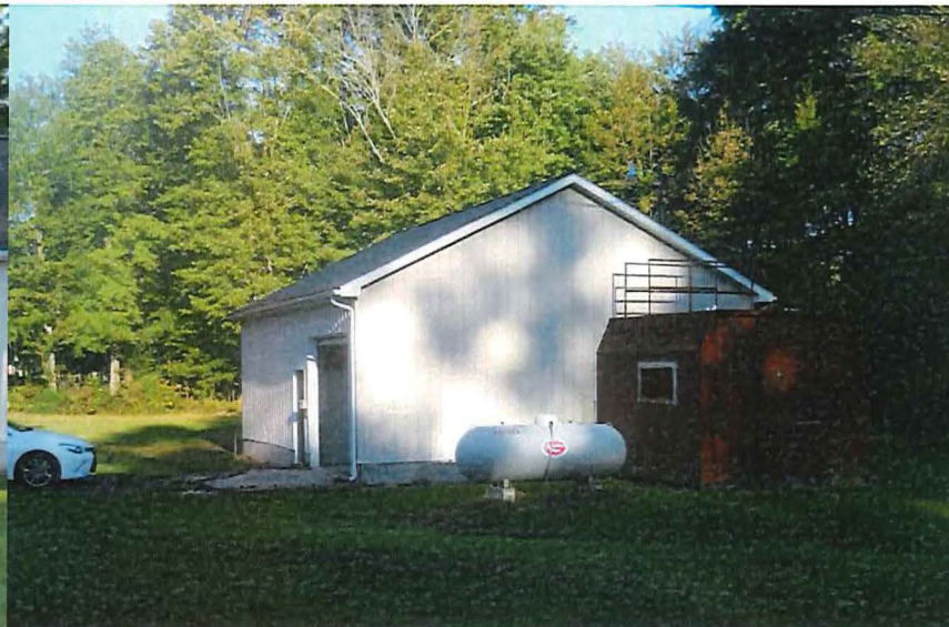
Fig. 6 View west of Control Building and out of service filter tank.
