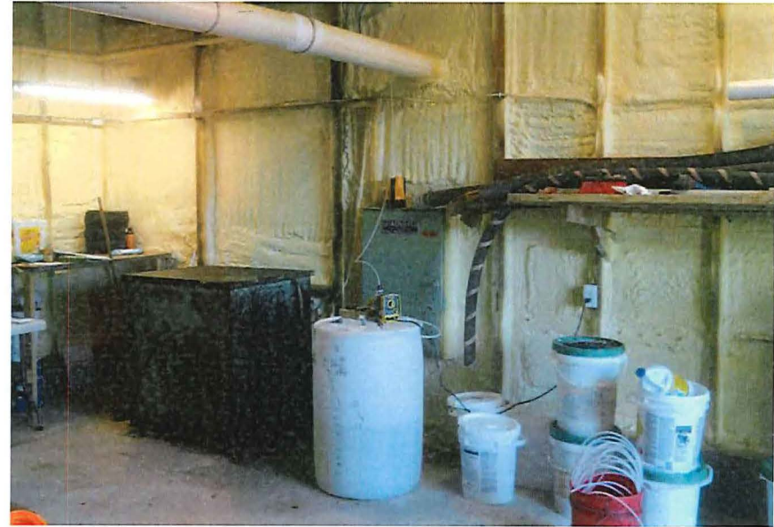
Fig. 10 Chemical feed system for effluent disinfection.
