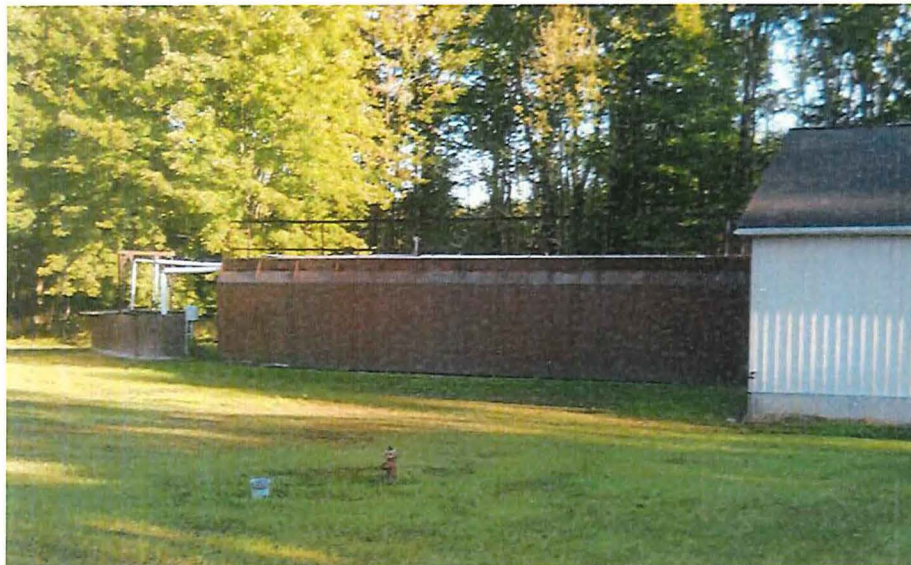
Fig. 5 View of Hillview Estates steel package treatment plant.
