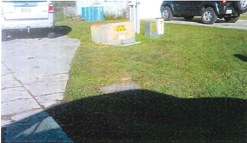
Fig. 1 Manhole on South Hillview Drive.
