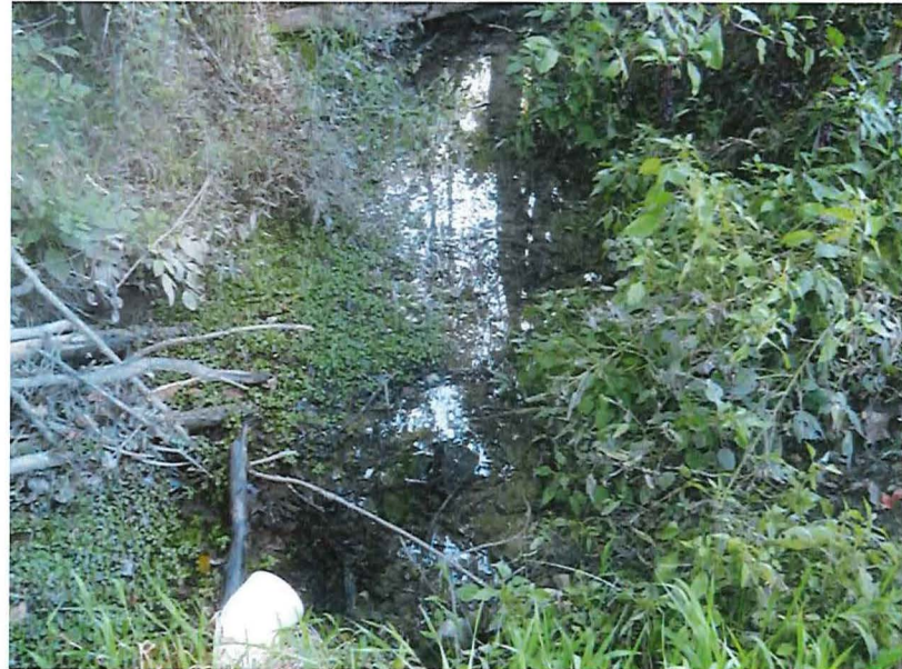
Fig. 16 View of Outfall 001 discharging to unnamed tributary.
