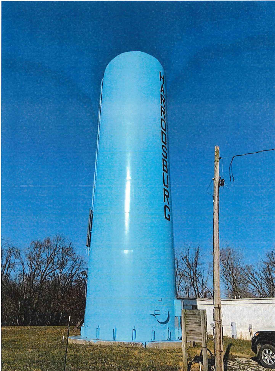
Harrodsburg tank – 100,000 gallons
