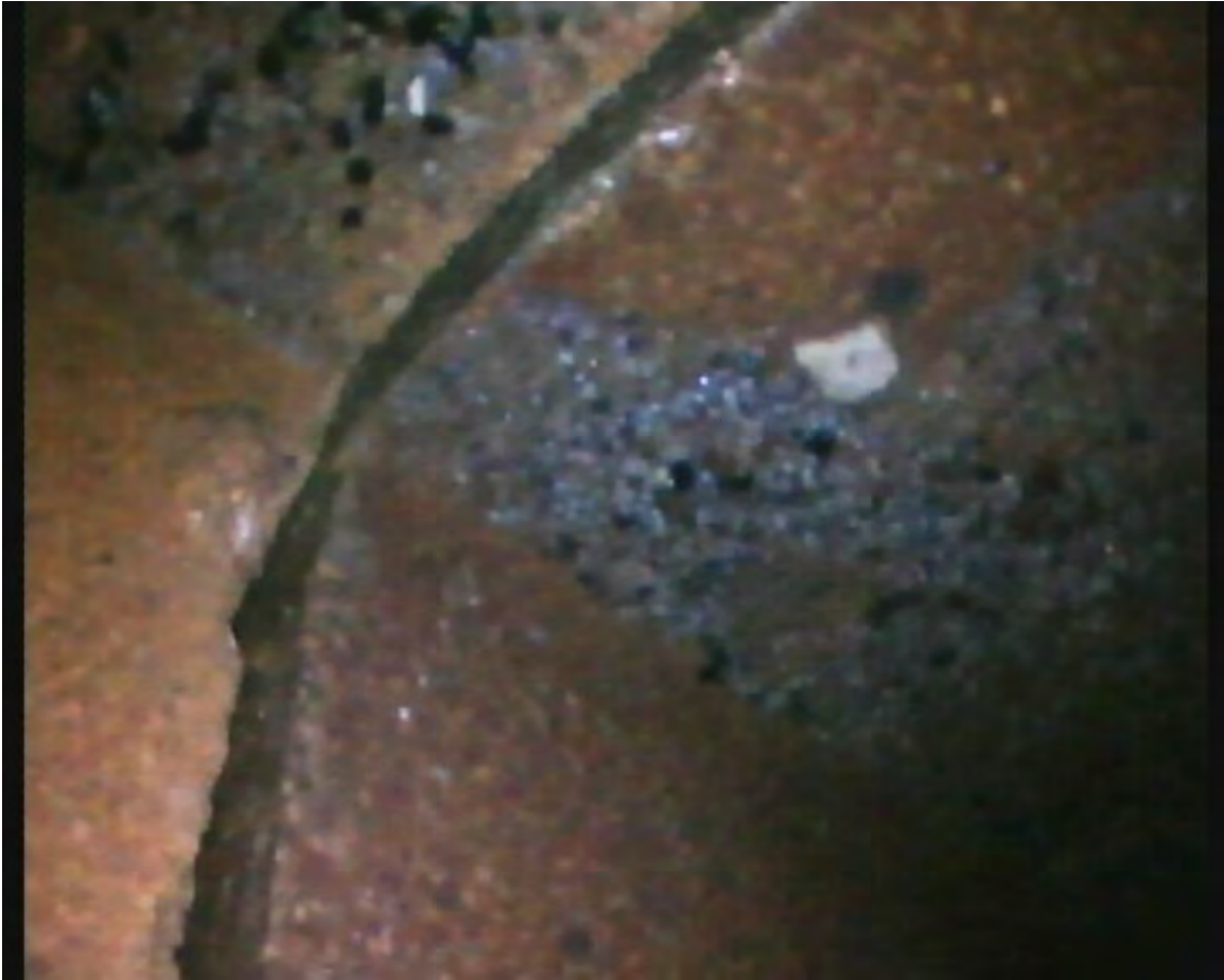
Filter 21 grout missing sides and bottom typical.
