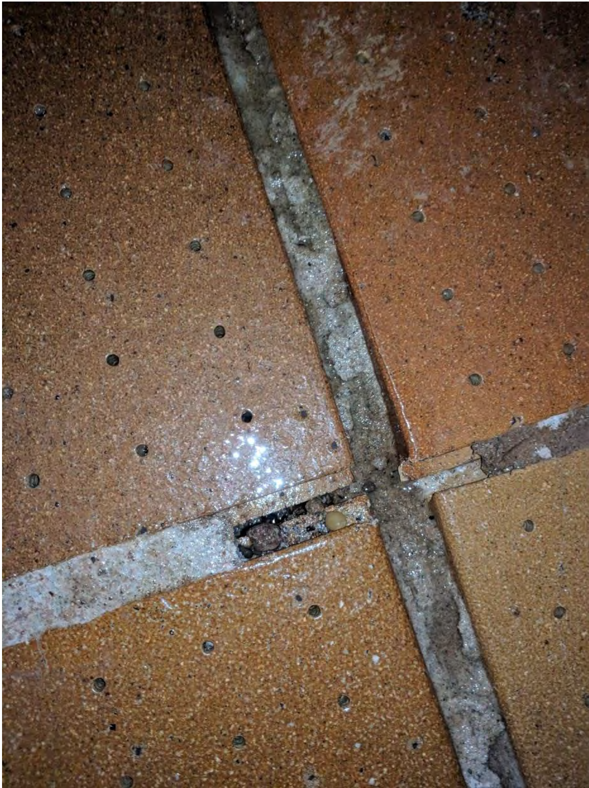
Typical filter 21 grout missing and separation from block.
