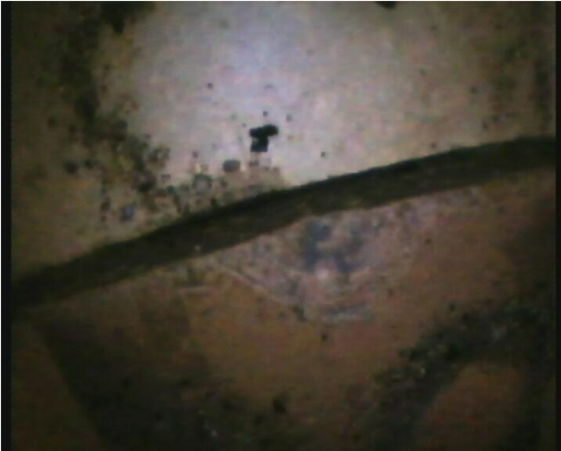
Filter 29 missing grout at the bottom head joint.
