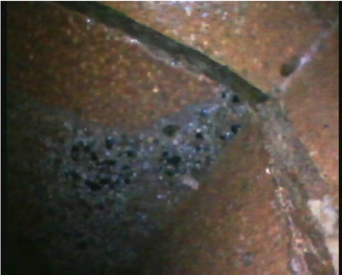
Internal Filter 21 missing grout on bottom. Grout is still in head joint.
