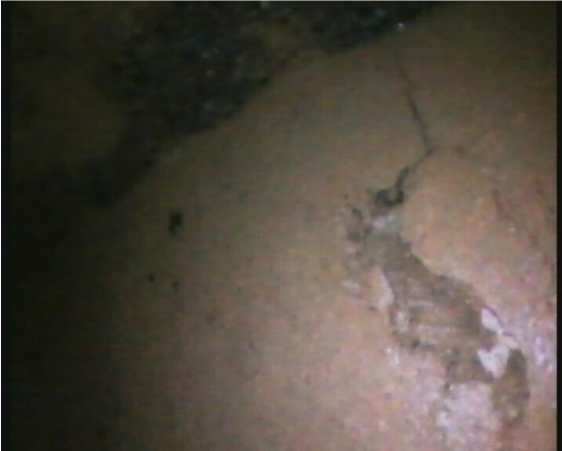
Filter 29, actual block breakage and cracks.
