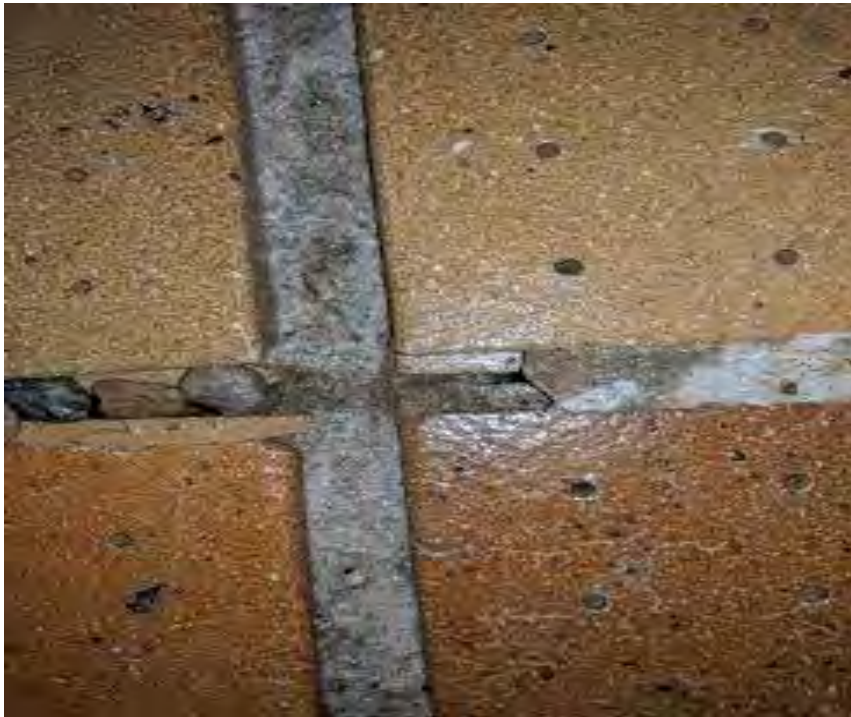
Typical grout missing and surface stress cracks
