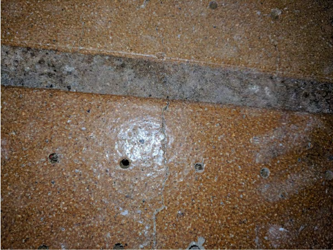
Typical surface cracks found throughout filter 21.
