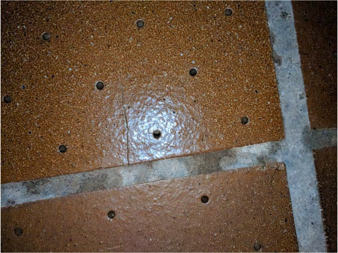
Filter 29 surface crack
