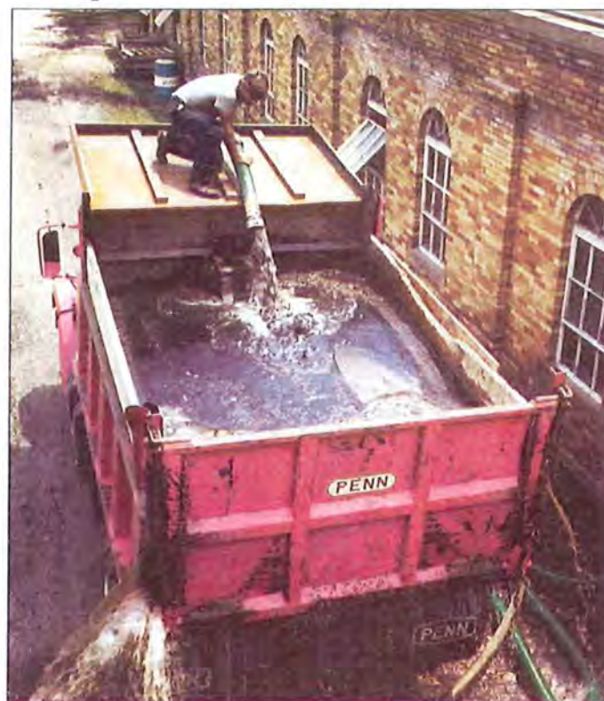
For years, utilities have replaced fouled filter media, but media can be washed and saved if sizes remain within acceptable ranges.
