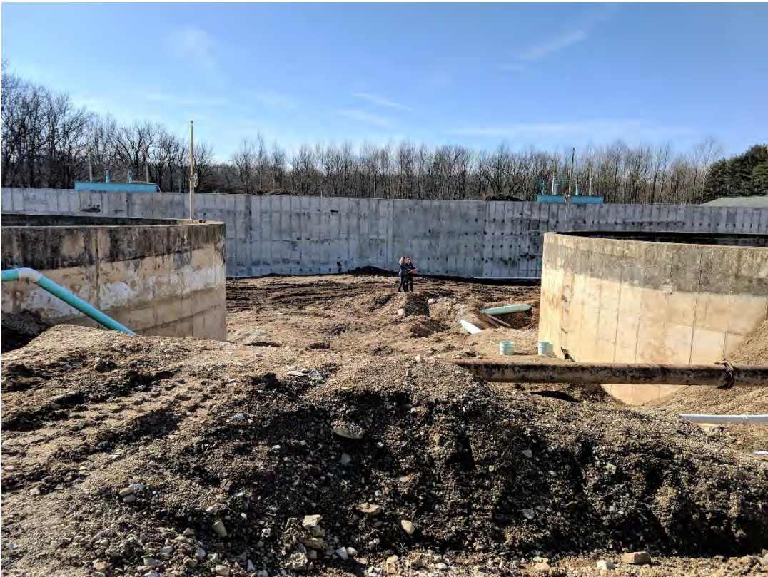
03/05/2020 Backfilling and site grading (Status: Not Complete)
