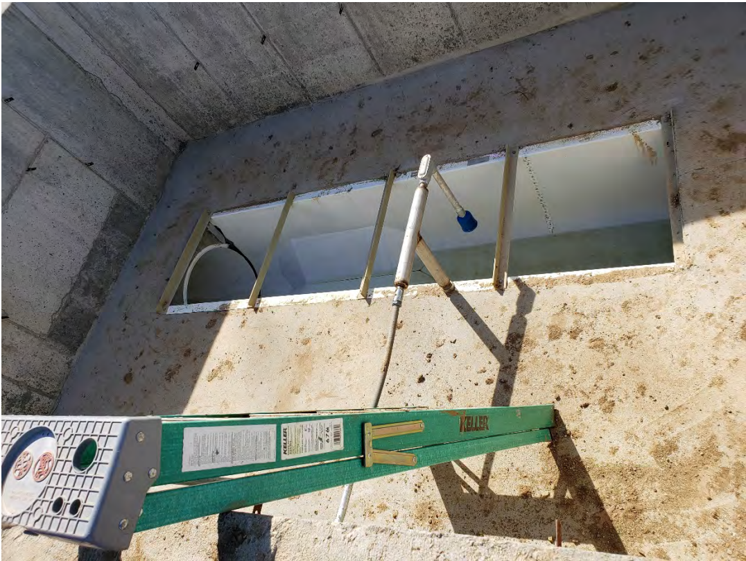
03/05/2020: Effluent Flow Meter – Access stairs not complete
