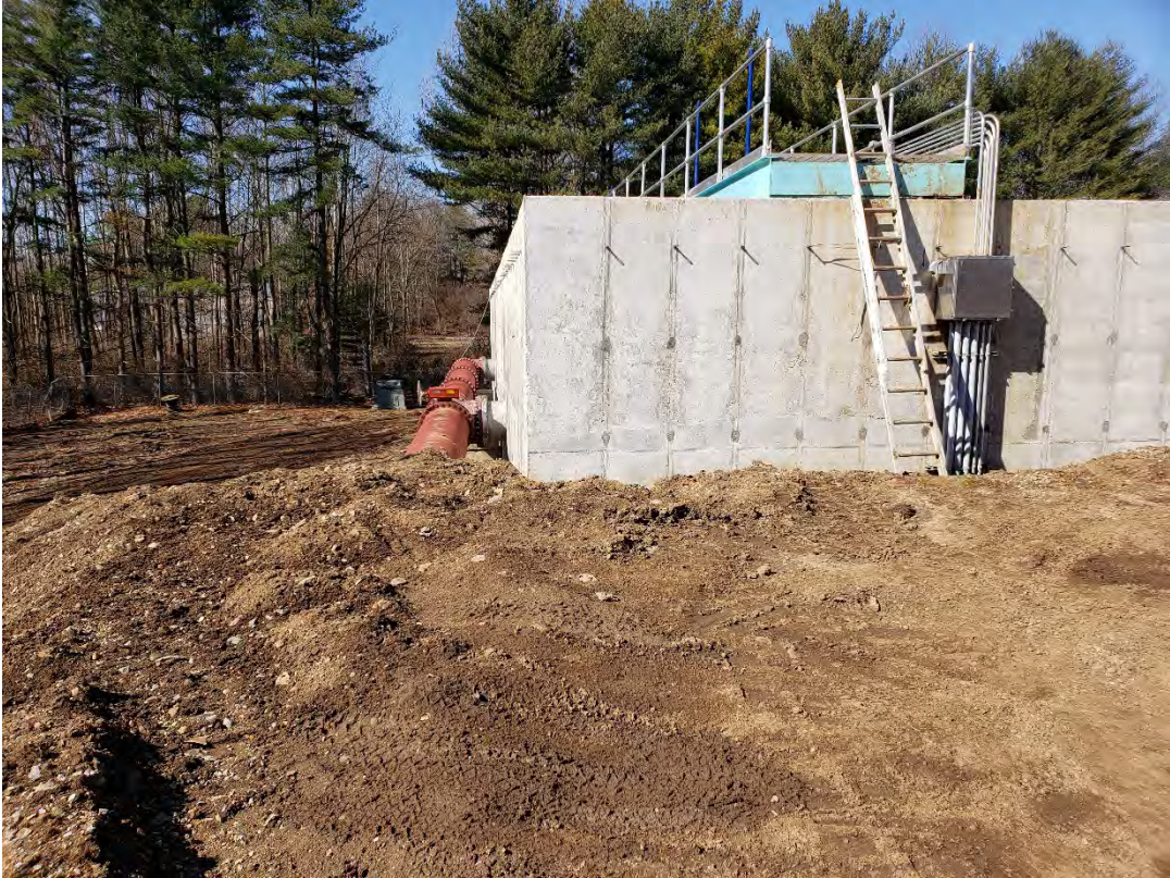
03/05/2020: Access stairs to new CSBR tanks not complete
