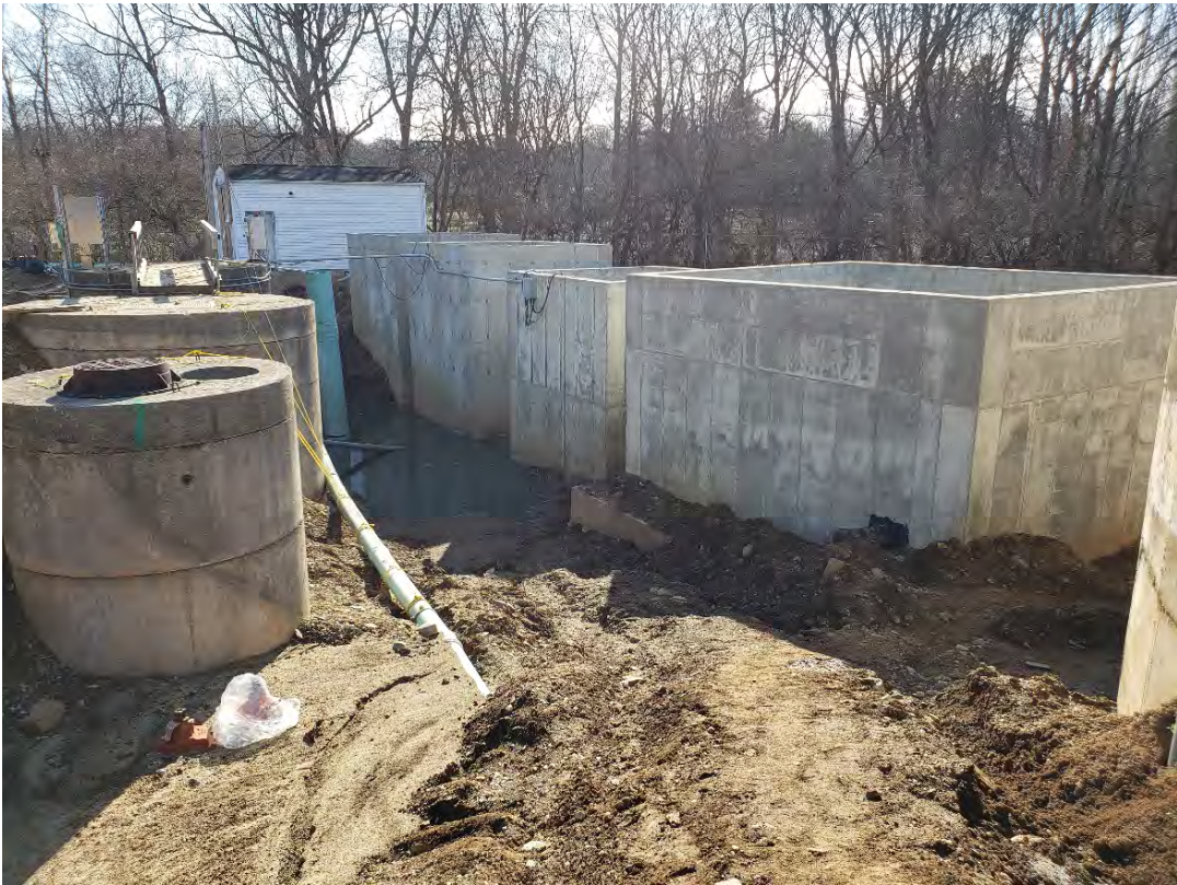
03/05/2020 – Backfilling headworks influent structures (Status: Not Complete)
