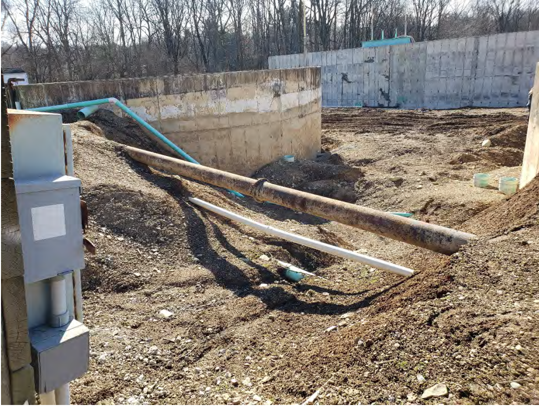
03/05/2020: Backfilling and rough grading not complete
