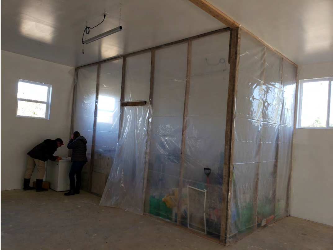
03/05/2020: Laboratory in Chemical Phosphorus Removal Building (Status: Not Complete)
