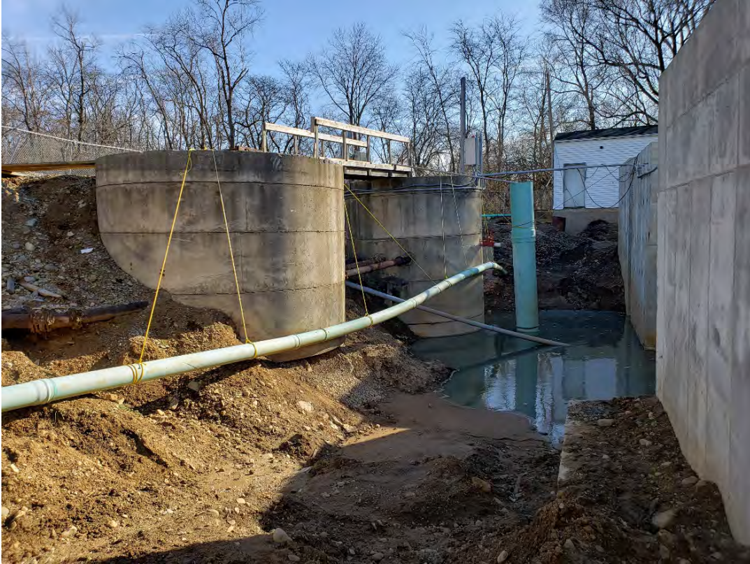
03/05/20 Backfilling headworks influent structures (Status: Not Complete)
