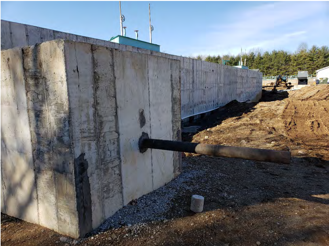
03/05/2020: Facilities under construction
