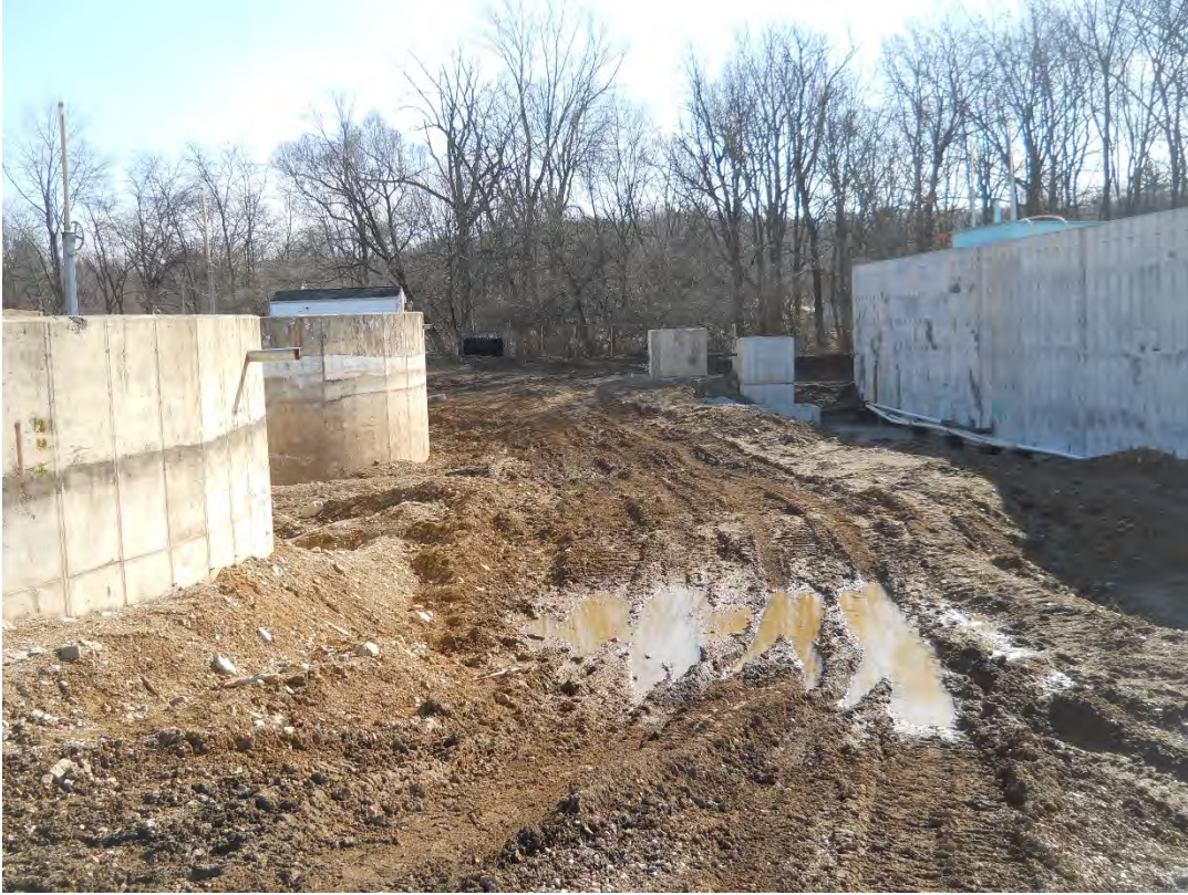
03/05/2020 Backfilling and site grading (Status: Not Complete)
