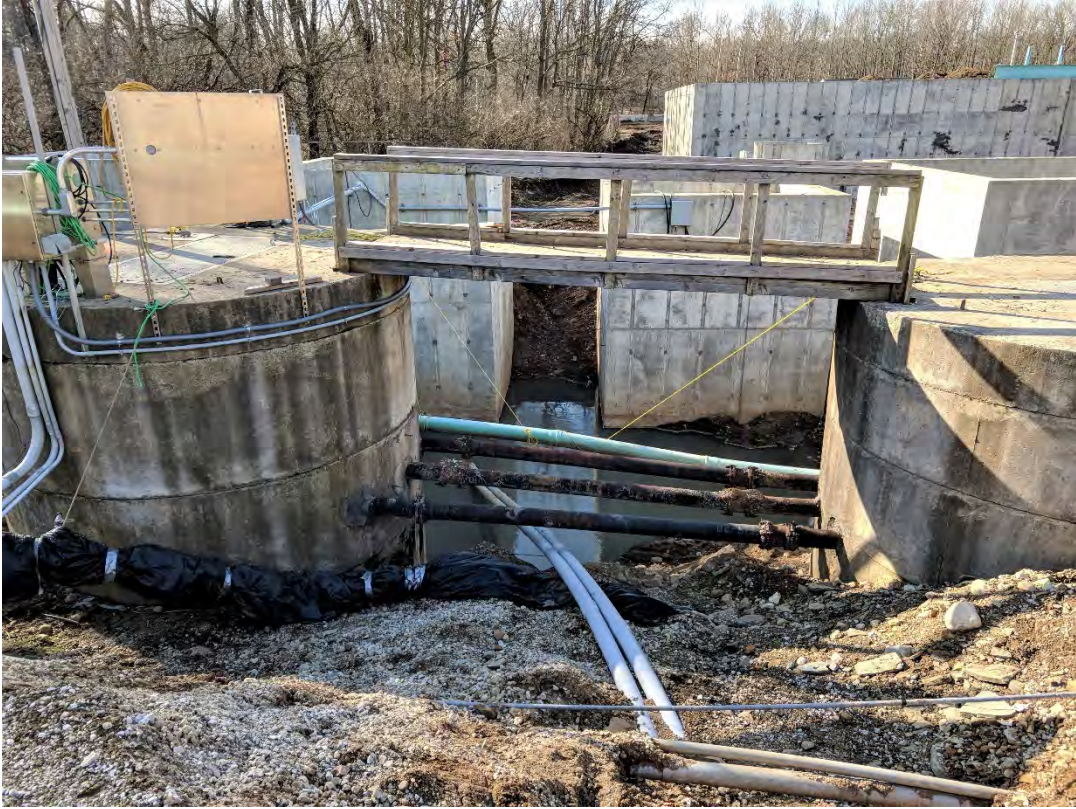
03/05/2020 – Backfilling headworks influent structures (Status: Not Complete)
