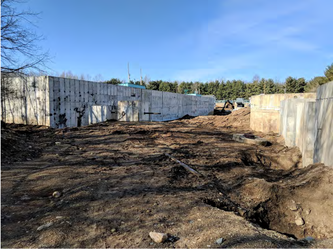
03/05/2020: Rough Site Grading (Status: Not Complete)
