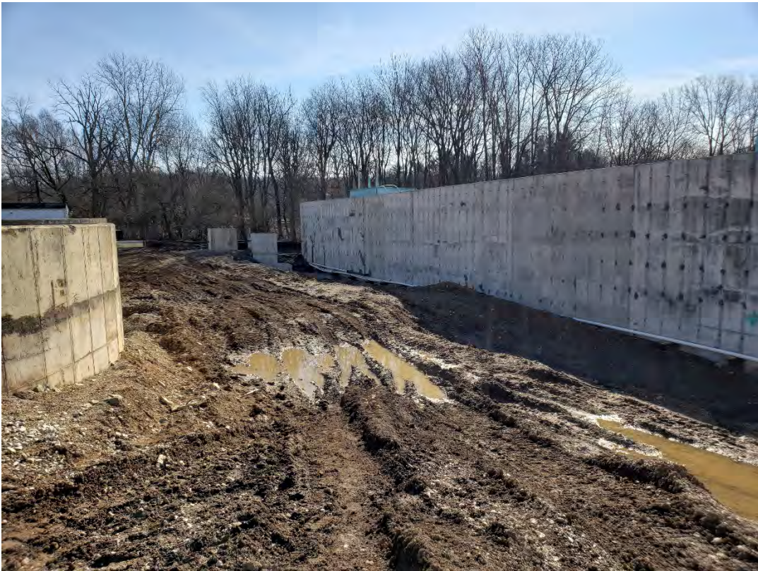
03/05/2020: backfilling, rough grading, access stairs and walkway for digester not complete
