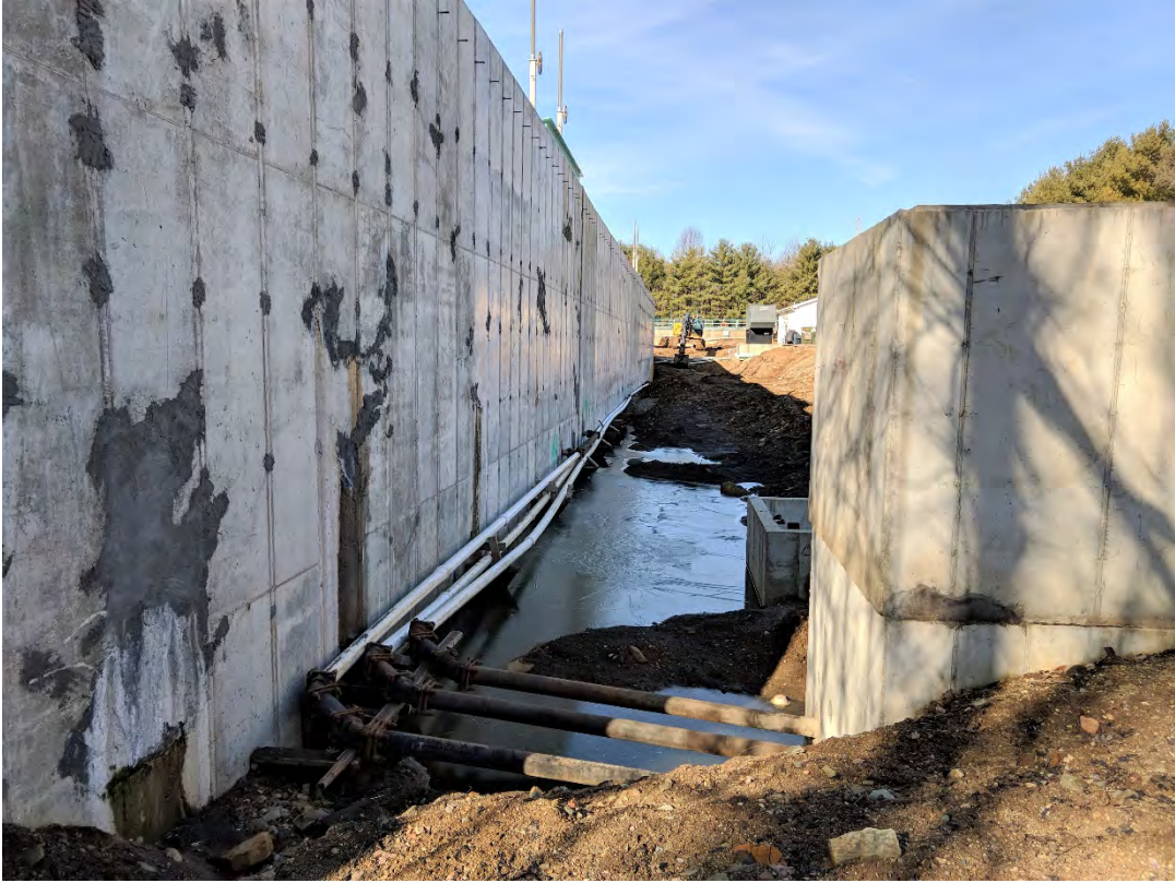
03/05/2020: Backfilling Digesters (Status: Not Complete)
