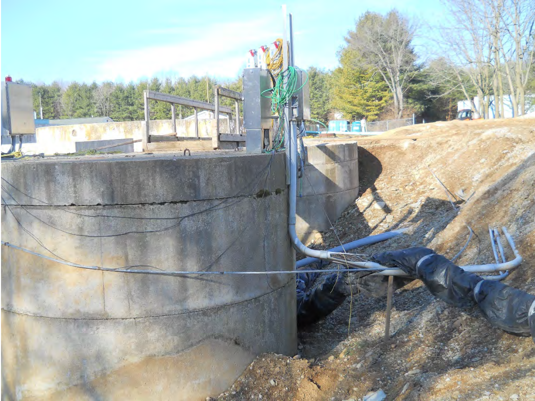
03/05/2020 Electrical work (Status: Not Complete)
