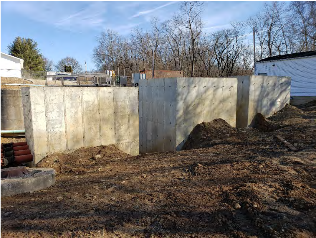
03/05/2020 Backfilling headworks influent structures (Status: Not Complete)
