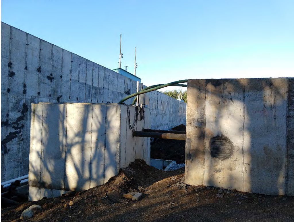
12/04/2019: Facilities still under construction
