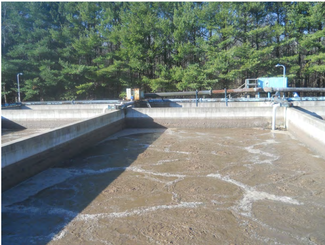
12/04/2019: CSBR Rehabilitation (Status: Not Completed)
