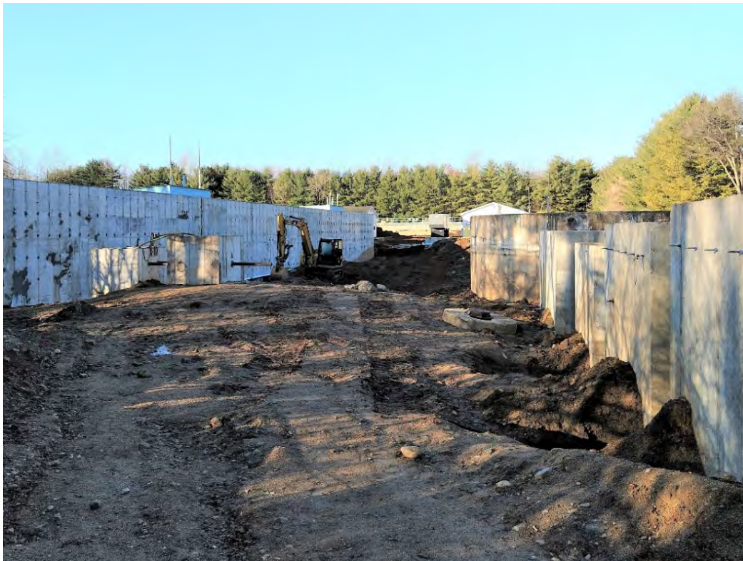
12/04/2019: Backfilling, site grading, digester stairs and walkway (Status: Not Complete)
