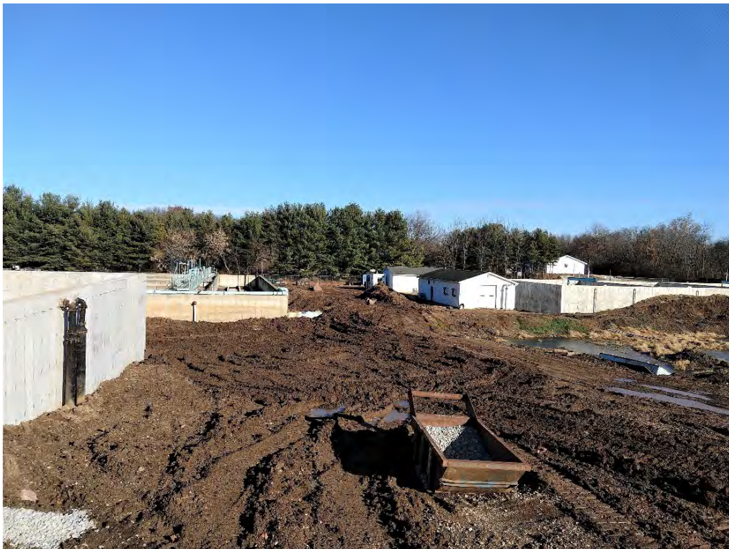
12/04/2019: Backfilling, site grading, pavement, sidewalks (Status: Not Complete)
