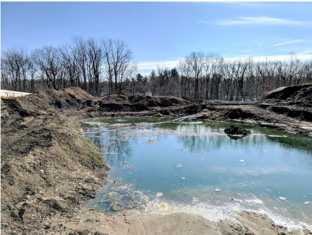
March 5, 2020, Sludge Lagoon removal and site grading (Status: Not complete)
