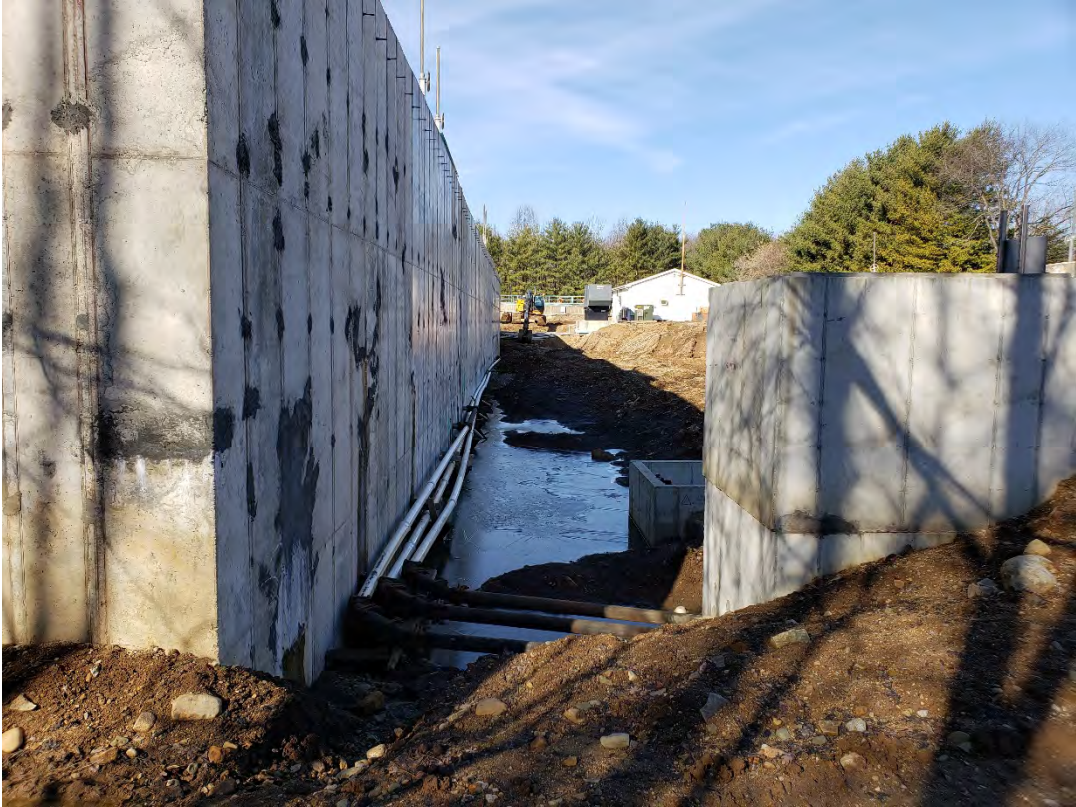
03/05/2020: Ongoing construction. Stairs and walkway for digesters not complete.
