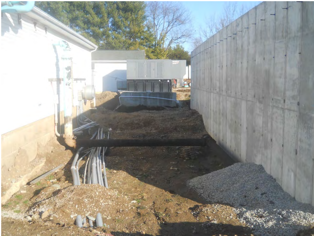
12/04/2019: Backfilling, site grading, exposed electrical conduit (Status: Not Complete)
