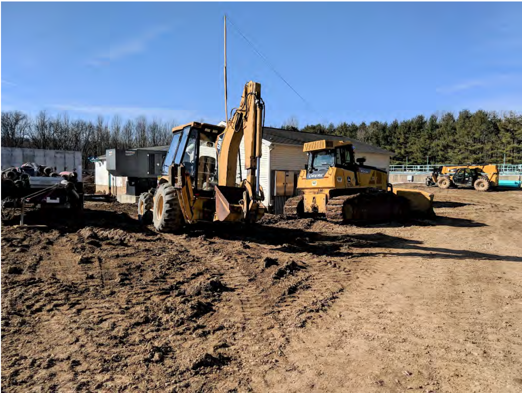
03/05/2020 Rough site grading, final grading, final pavement, sidewalks (Status: Not Complete)
