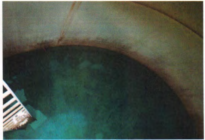
Interior Sidewall Coating
