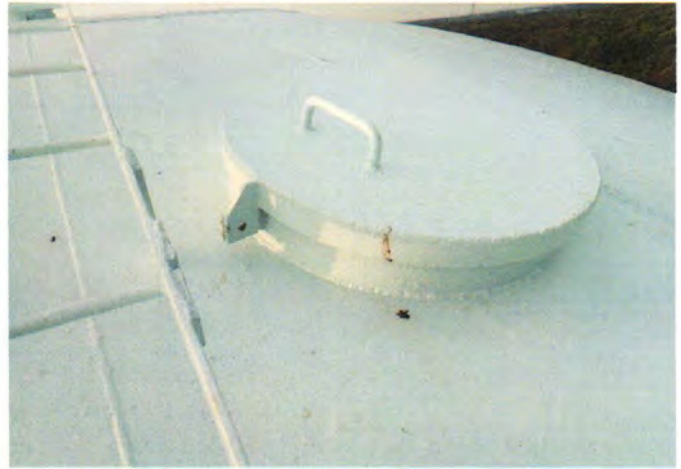
Wet Interior Access Hatch
