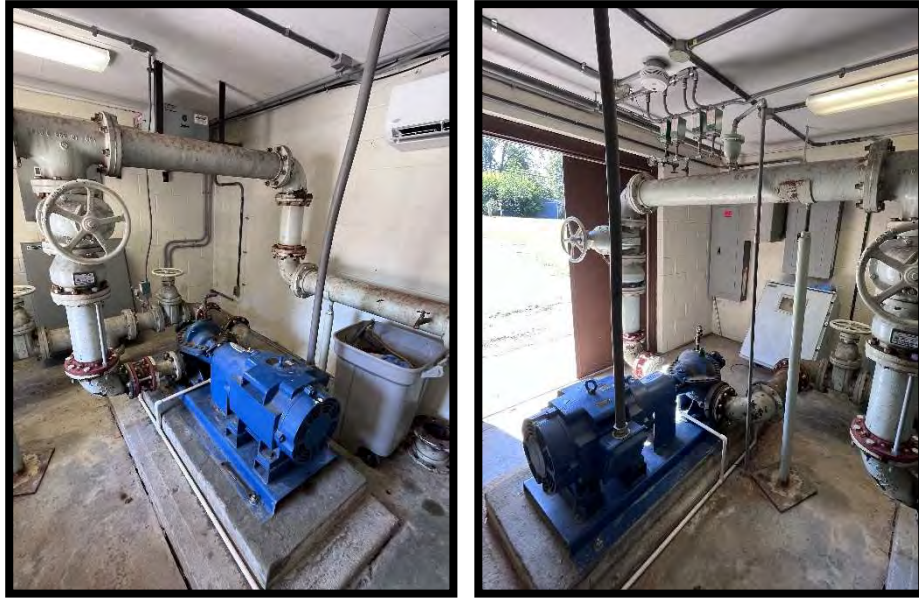
Booster Pumps and Process Piping
