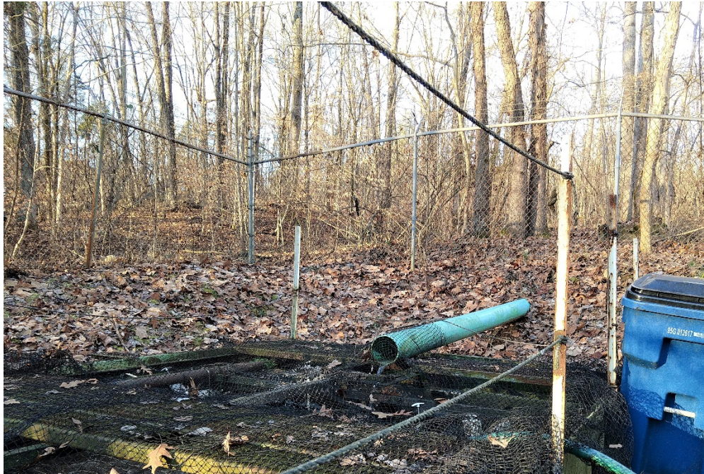
Existing corroded steel influent pipe was replaced with PVC
