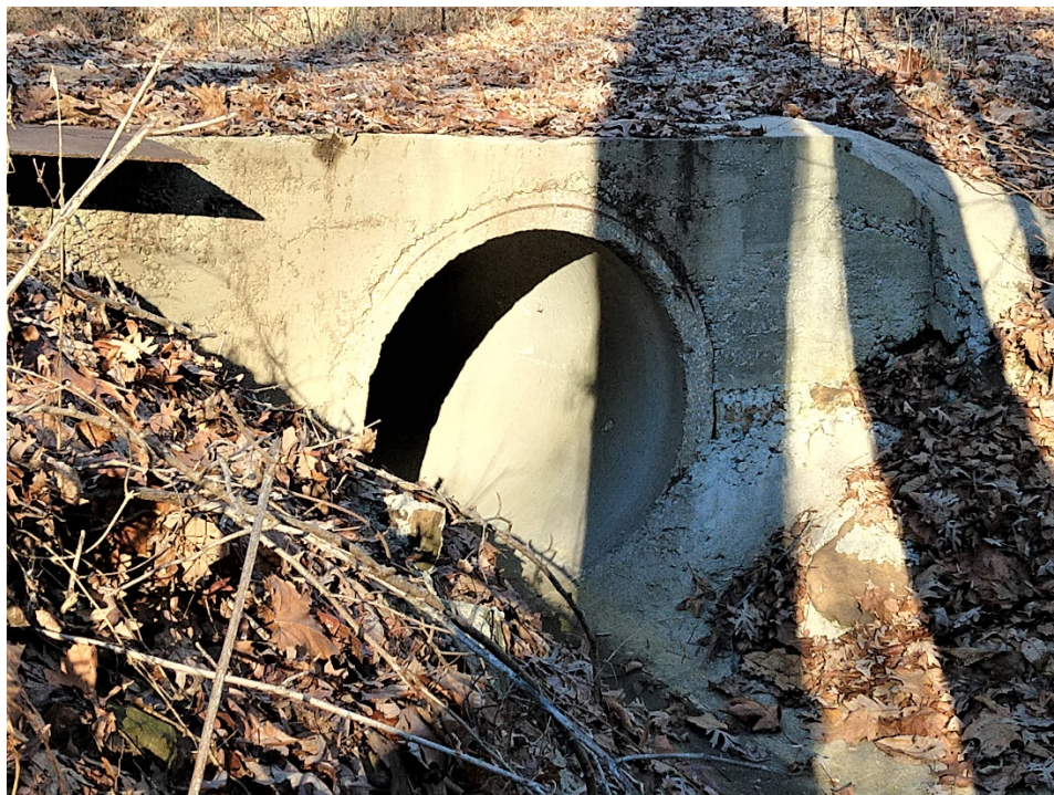
New concrete culvert installed to replace failing corrugated steel culvert
