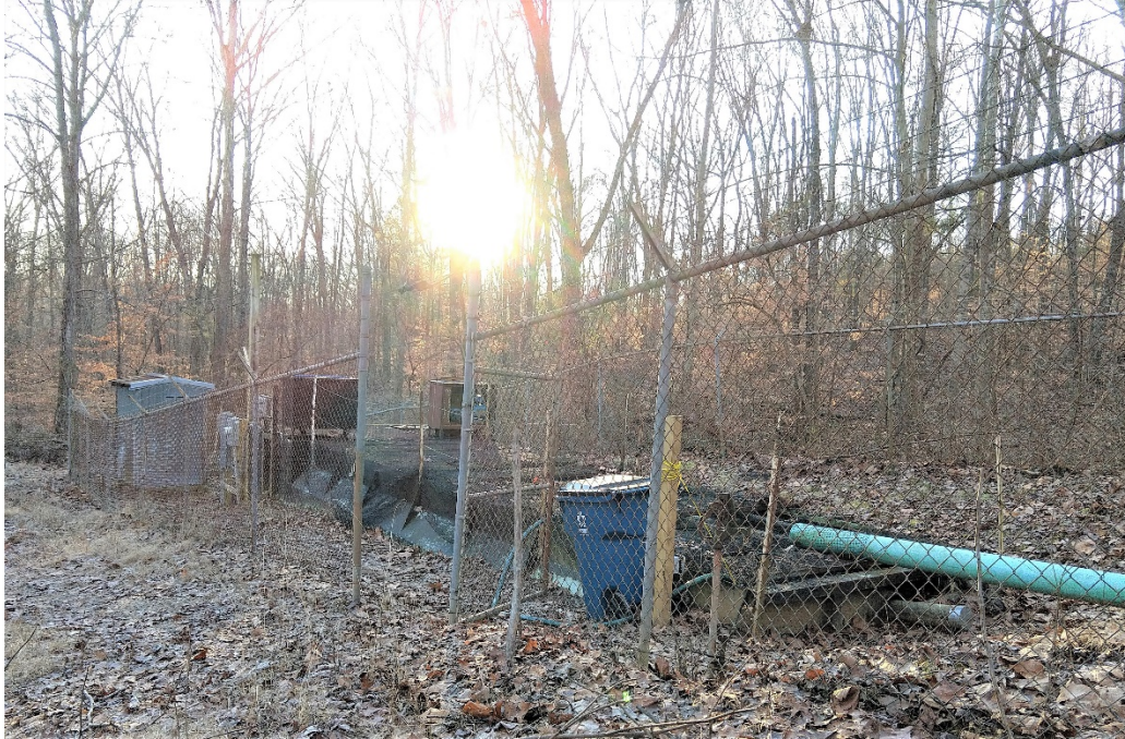
View of plant showing new PVC influent pipe (R), blower motor housings above tank (C) and existing outbuilding
