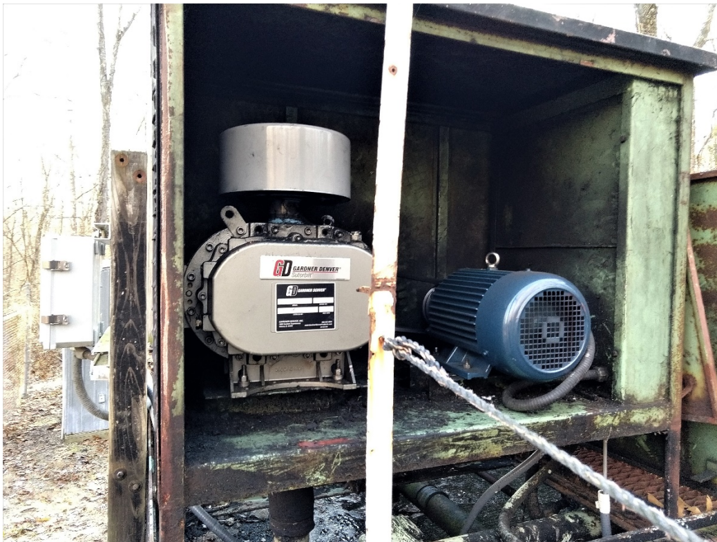
New north blower motor – Aqua intends to move this and south blower from top of structure at later date
