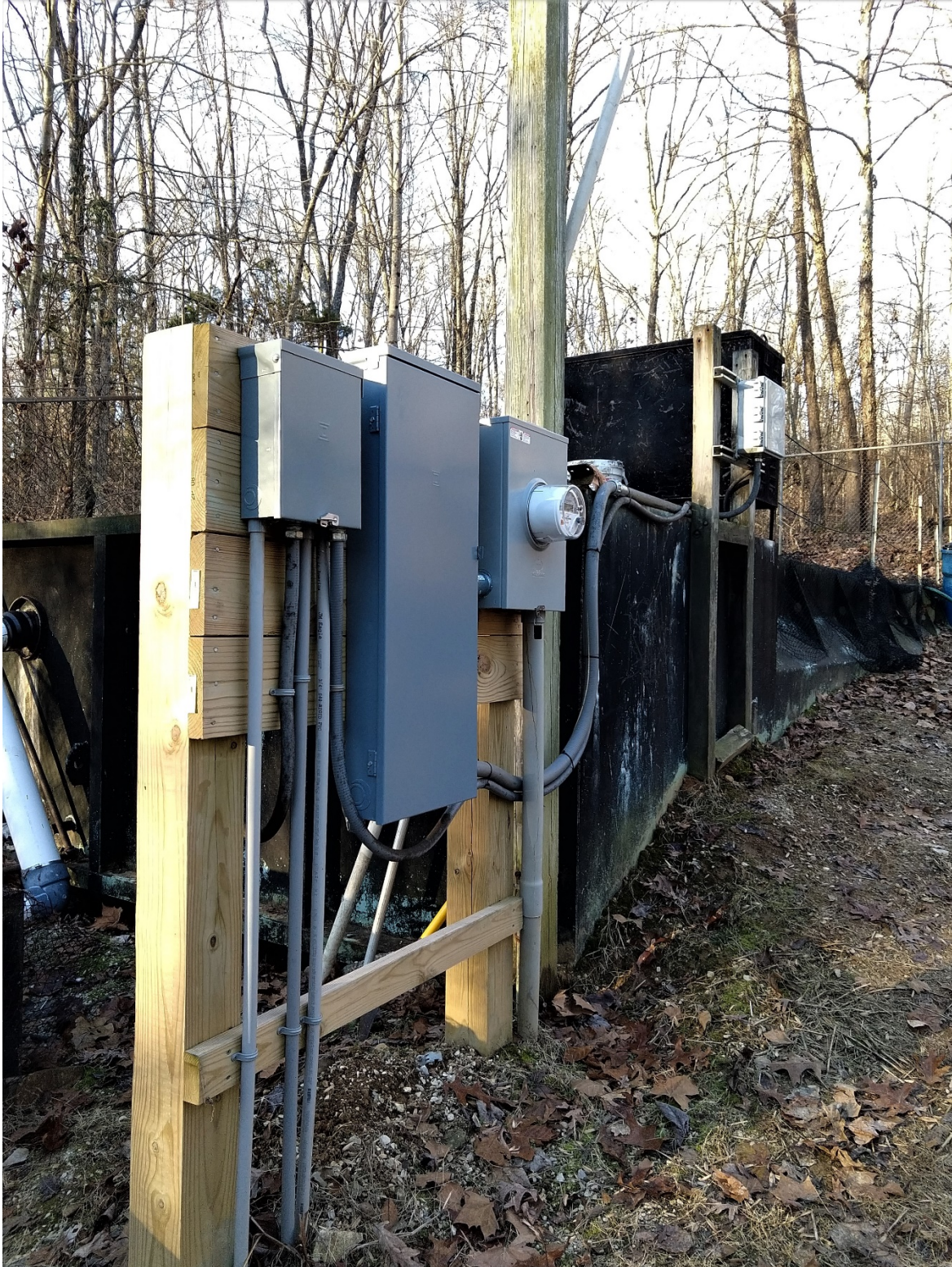
View of new board, electrical control panel, electrical service now buried. New dialer at far right
