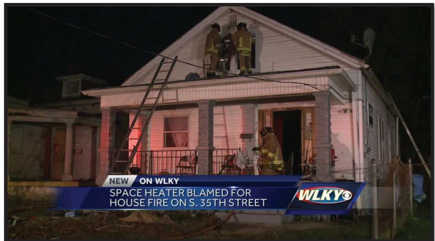
Louisville, KY November 15, 2016: House Fire caused using space heater Source: WLKY, Kentucky
