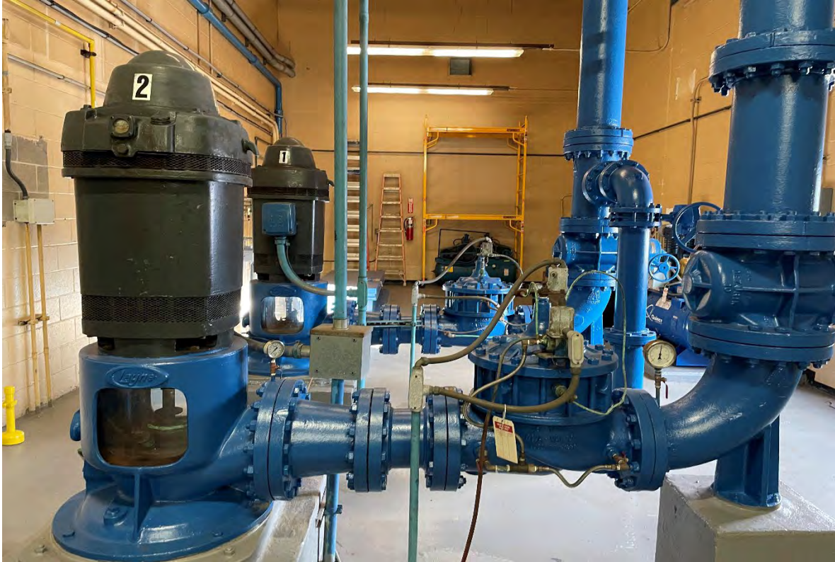
Austin Water Treatment Plant High Service Pumps
