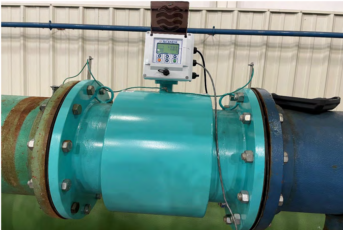
Marble Hill Water Treatment Plant Flow Monitor
