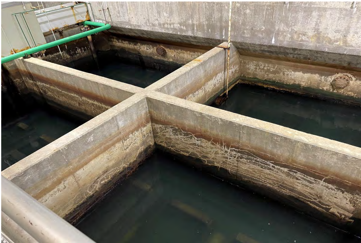
Austin Water Treatment Plant Filtration Tanks
