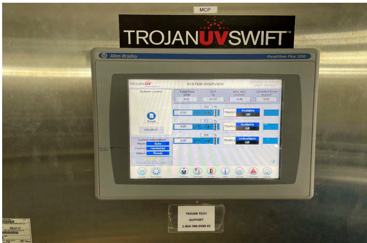
Austin Water Treatment UV System Control Panel
