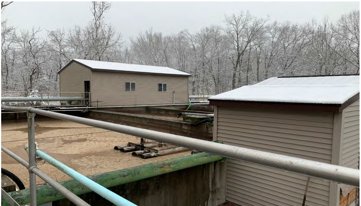
Sequence Batch Reactor Tanks Photo 2
