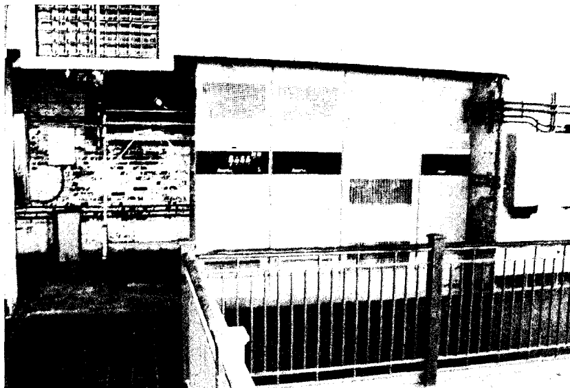
FIGURE 2-14 VFD for HSP No. 5
