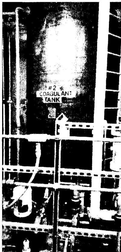
FIGURE 2-18 Coagulant Day Tank
