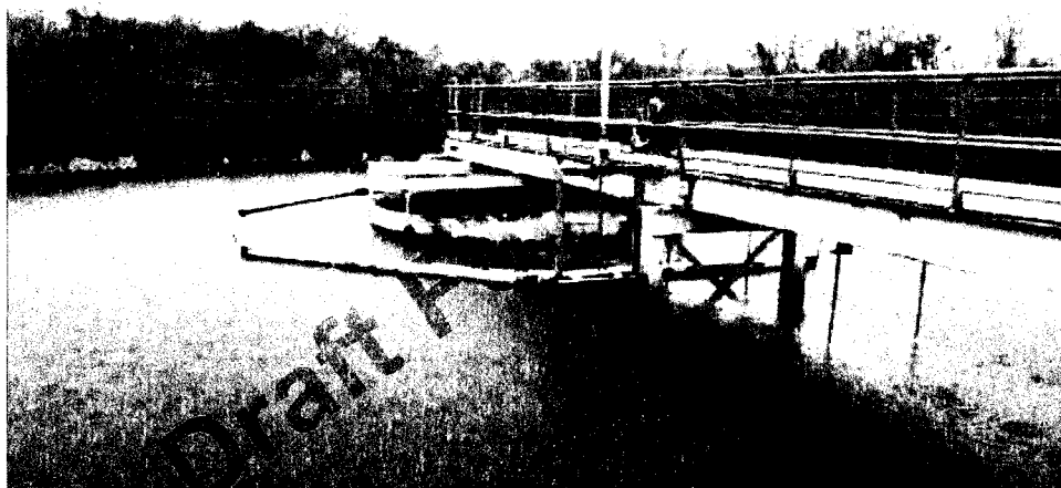
FIGURE 2-12 South Plant Secondary Clarifier
