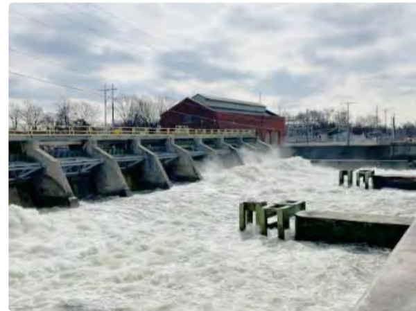
Elkhart Hydroelectric Plant
