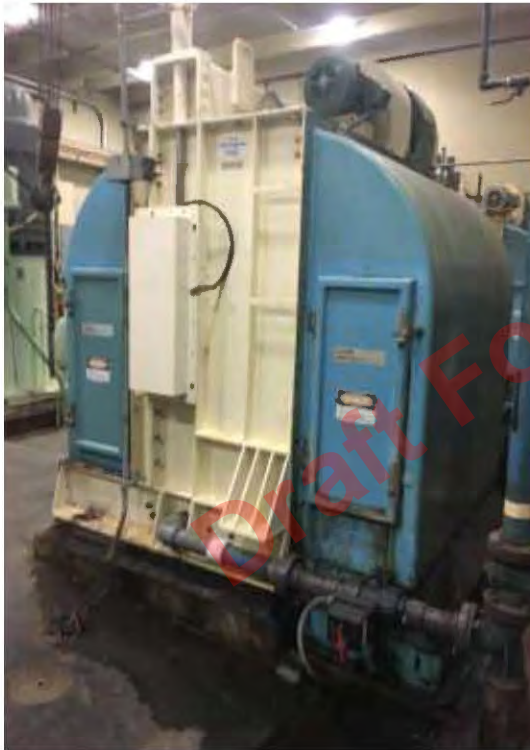
FIGURE 2-1 Traveling Screen
