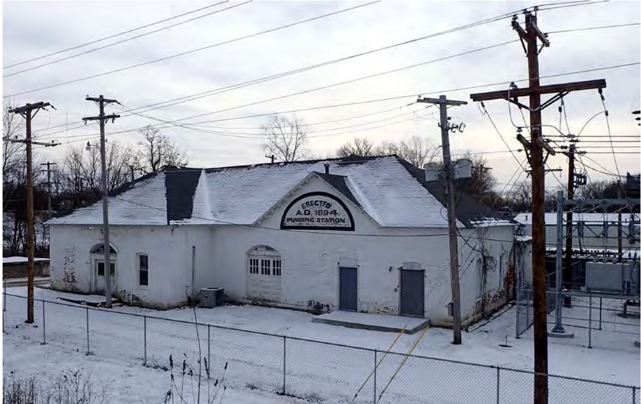
Front, exterior view of plant from US 40, showing adjacent substation
