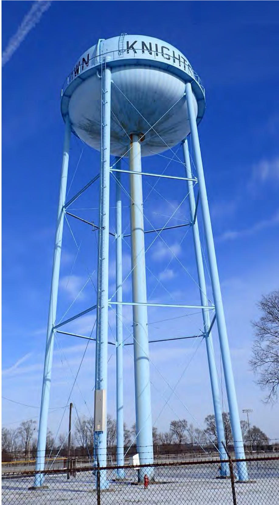
250,000 gallon elevated storage tank
