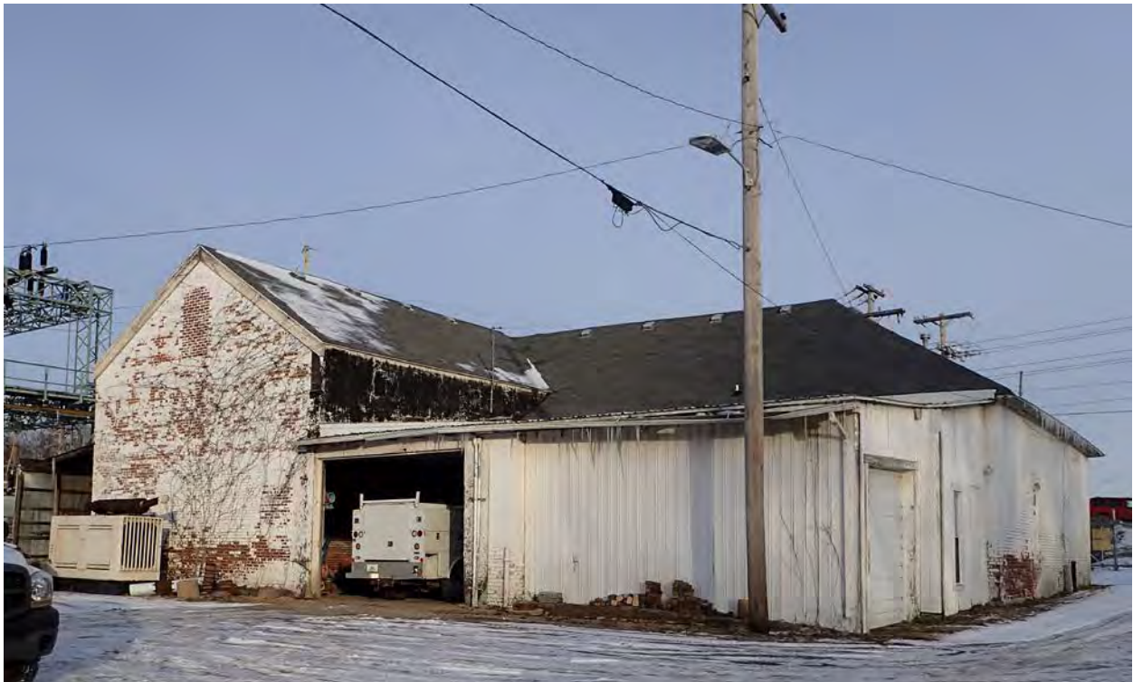
Rear, exterior view of plant
