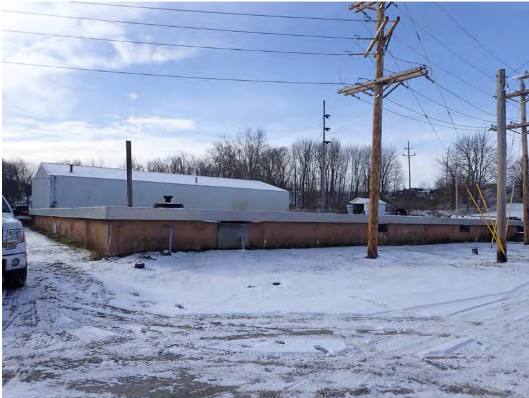
210,000 gallon clearwell behind plant
