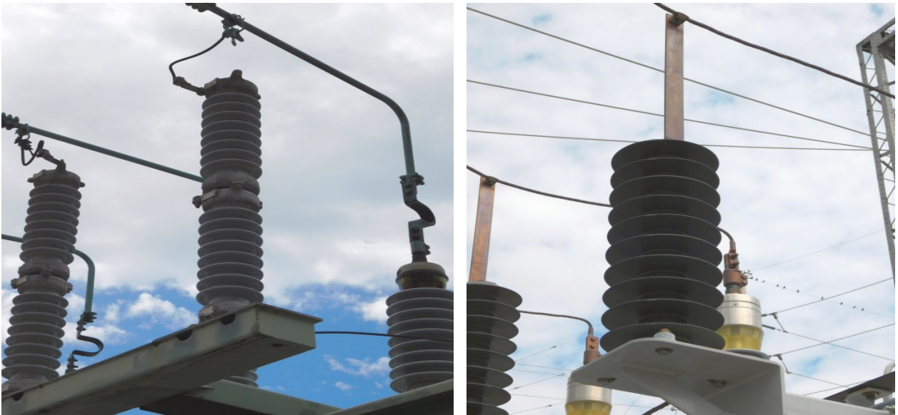
Figure 2. Example of aged porcelain arrester (left) and modern polymer arrester (right)
