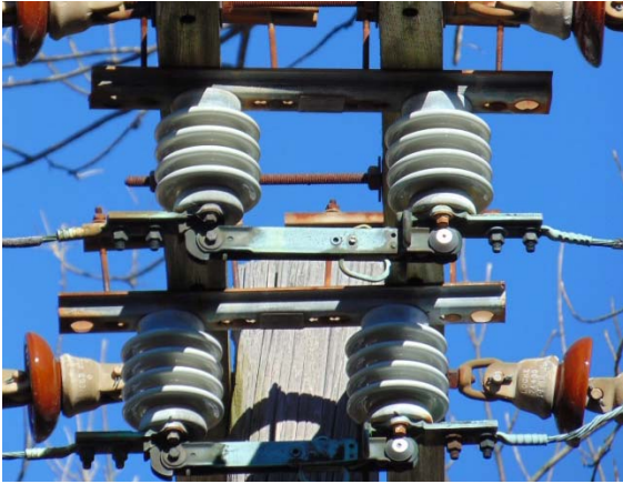
Figure 2. Example of closed underslung switch (left) and example of open underslung switch (right). Since switches are not gang operated, they must be opened or closed one at a time.
