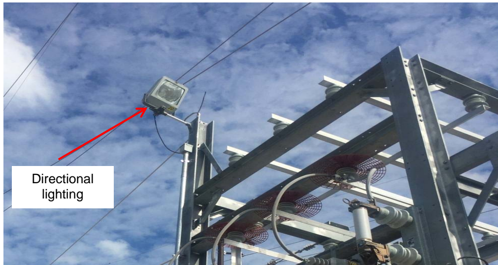
Figure 1. Additional lighting added to structures
