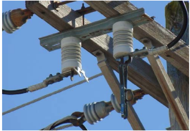
Figure 2. Example of closed underslung switch (left) and example of open underslung switch (right). Since switches are not gang operated, they must be opened or closed one at a time.
