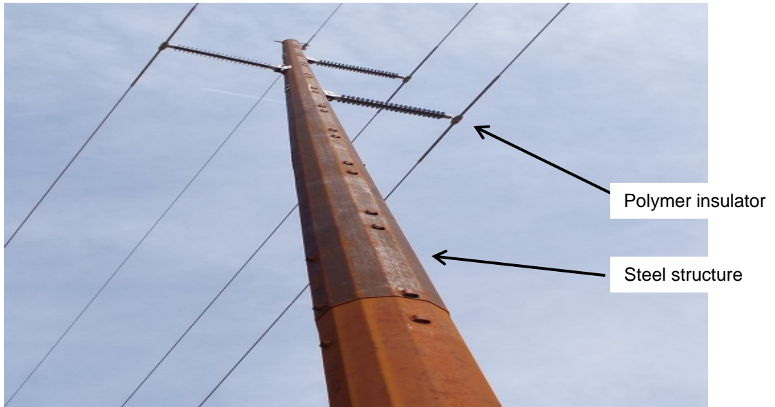
Figure 1. New construction of a transmission line using a steel pole
