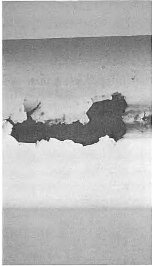
Frank Ott Tank — 100,000 gallon Elevated
