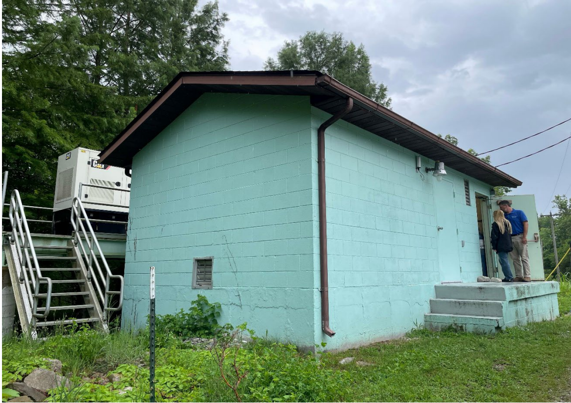
White River Wellfield Water Treatment Plant Exterior
