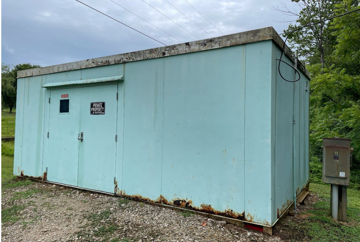
Doans Booster Station Exterior
