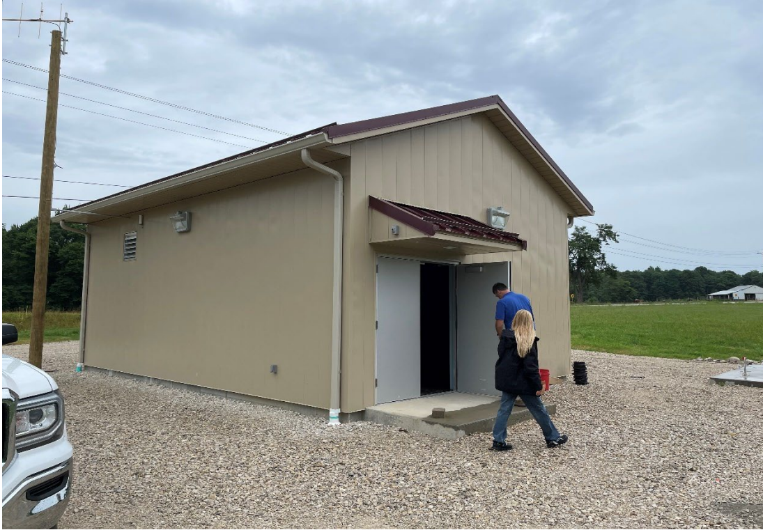
New Booster Station #2 Exterior
