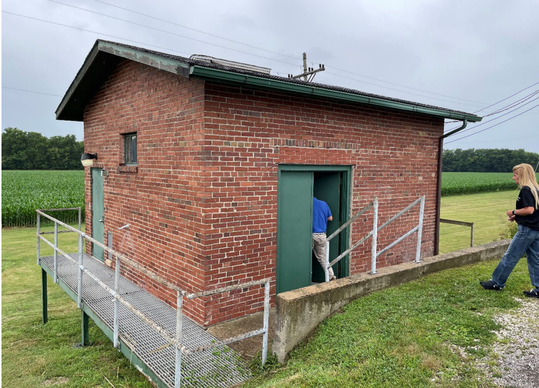
Bloomfield Wellfield Water Treatment Plant Exterior
