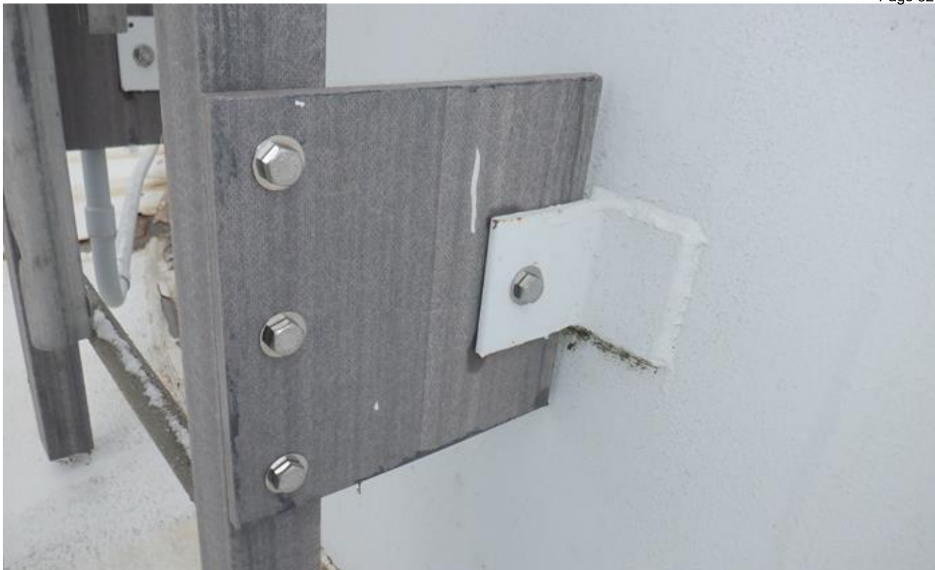
27. Middle tank section ladder bracket.
