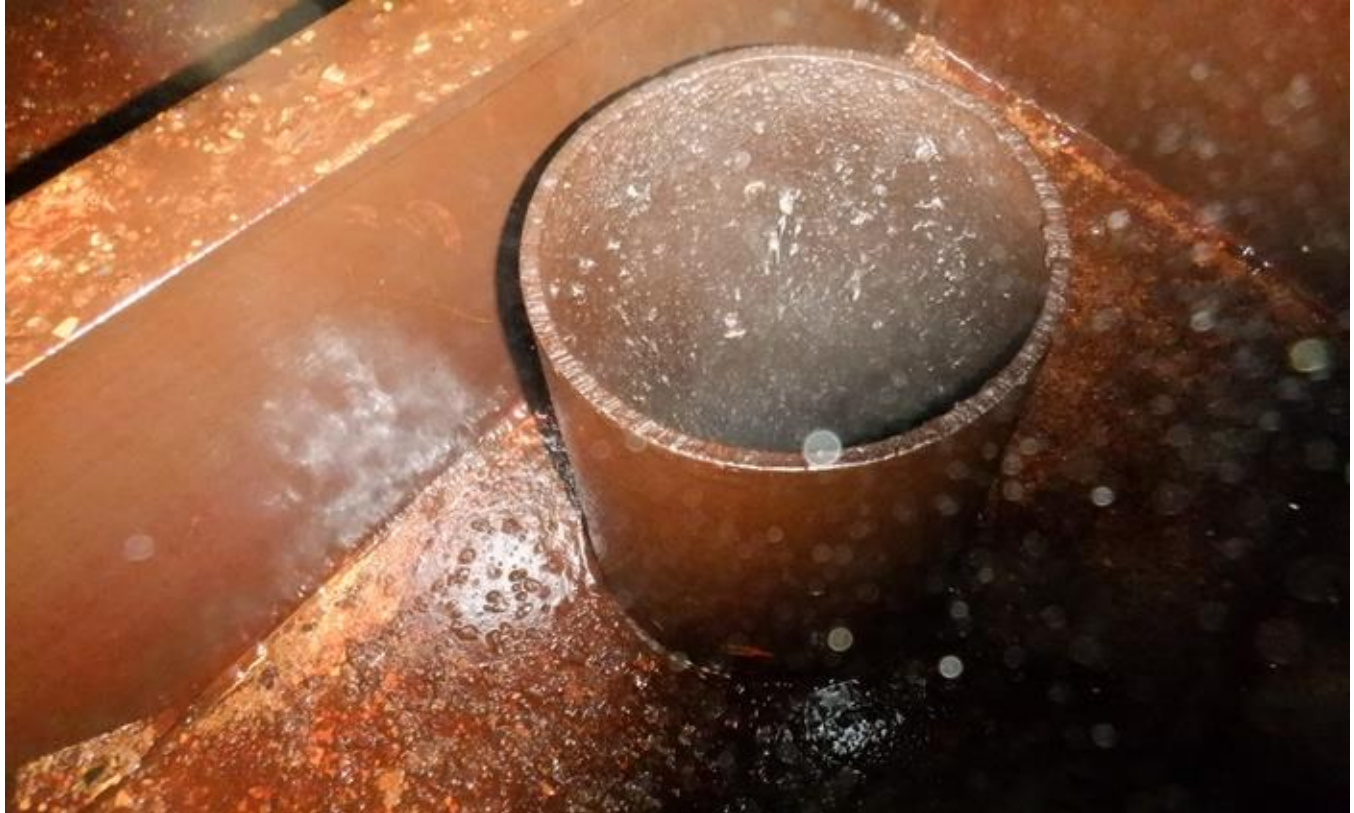
66. Pipe and stiffener at bottom of middle tank section.
