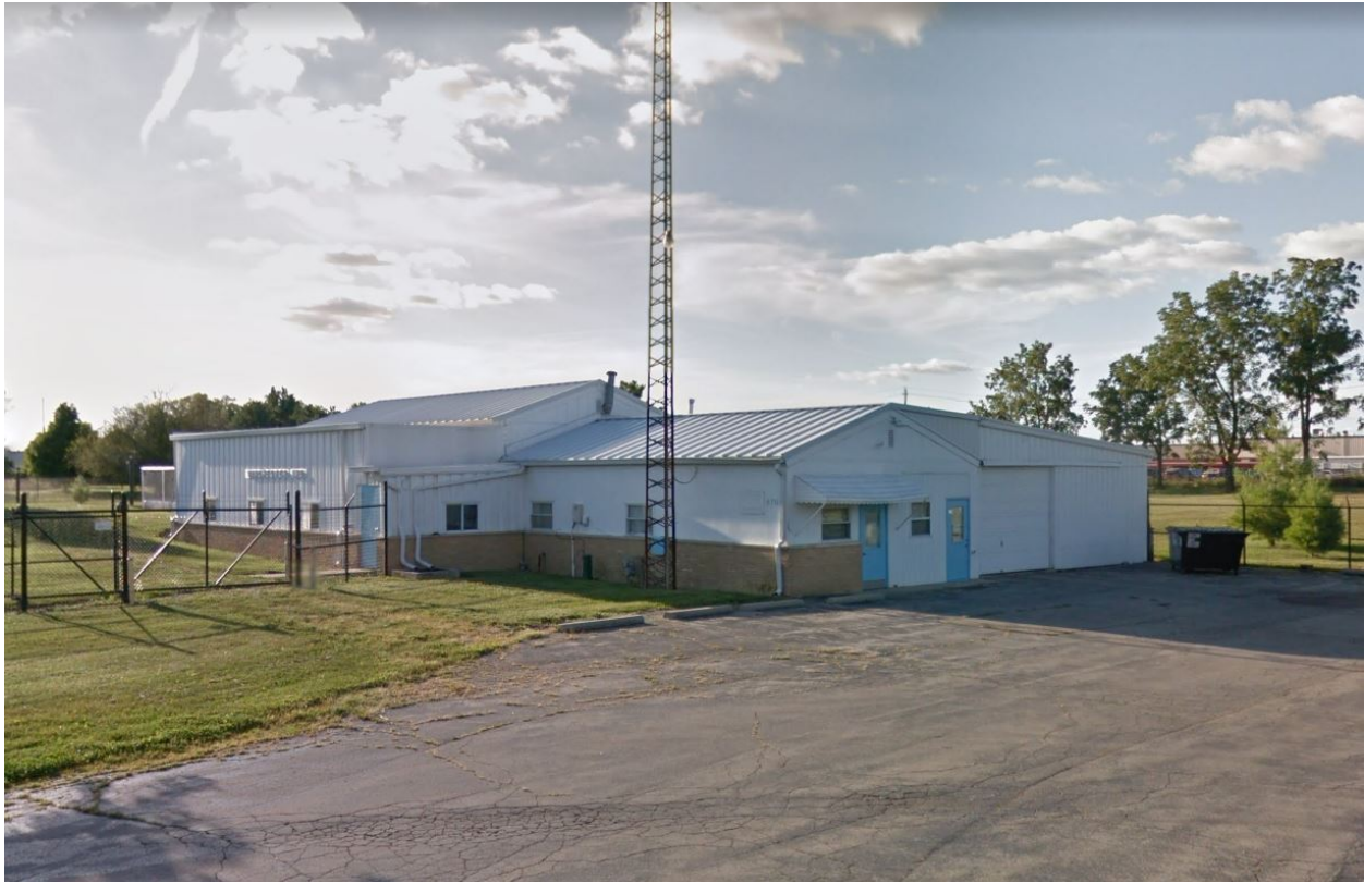
Exhibit 1-1: Winchester WTP chemical building exterior (looking at south wing)
