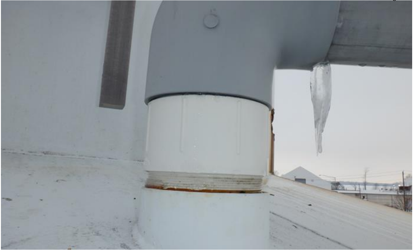
35. Overflow pipe projection and icicle.
