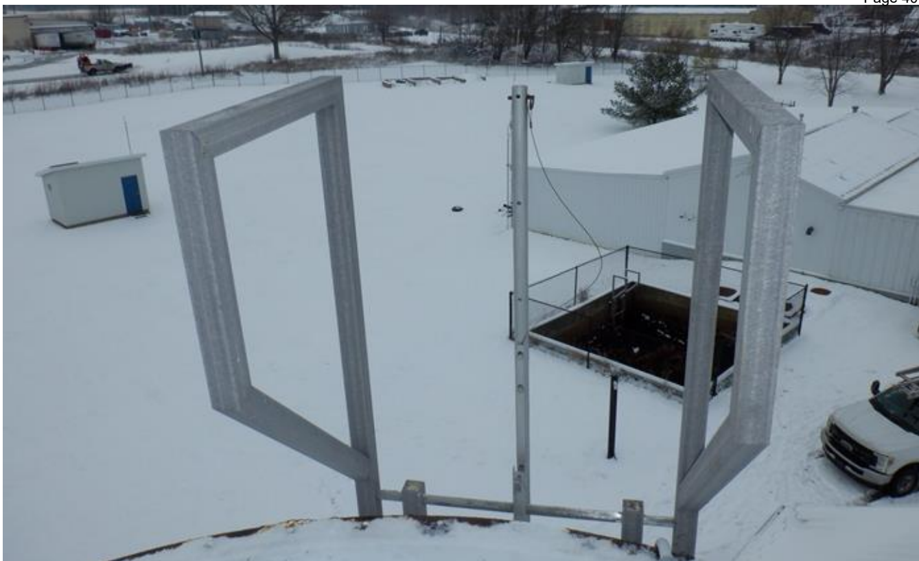
43. Top tank section roof access.
