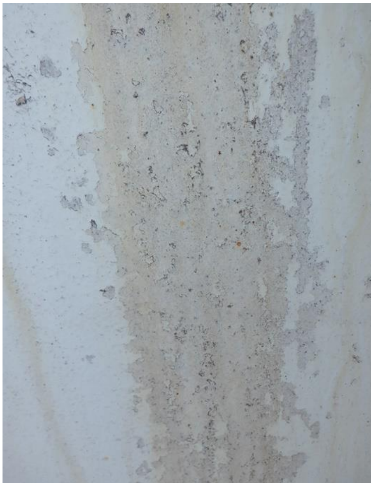
11. Coating failure and corrosion on shell coating.
