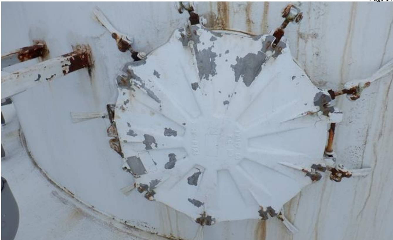
25. Shell manhole in middle section.
