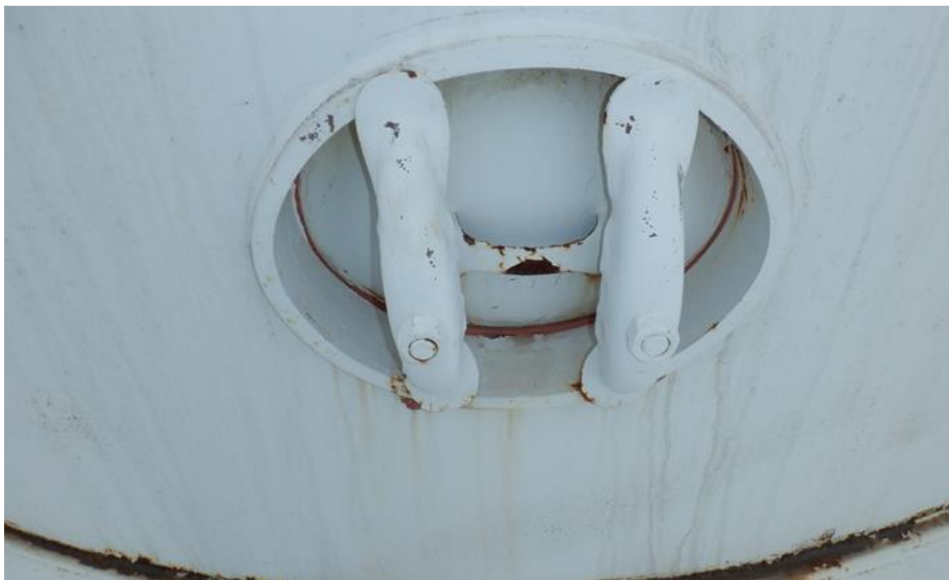
24. Shell manhole in middle section.
