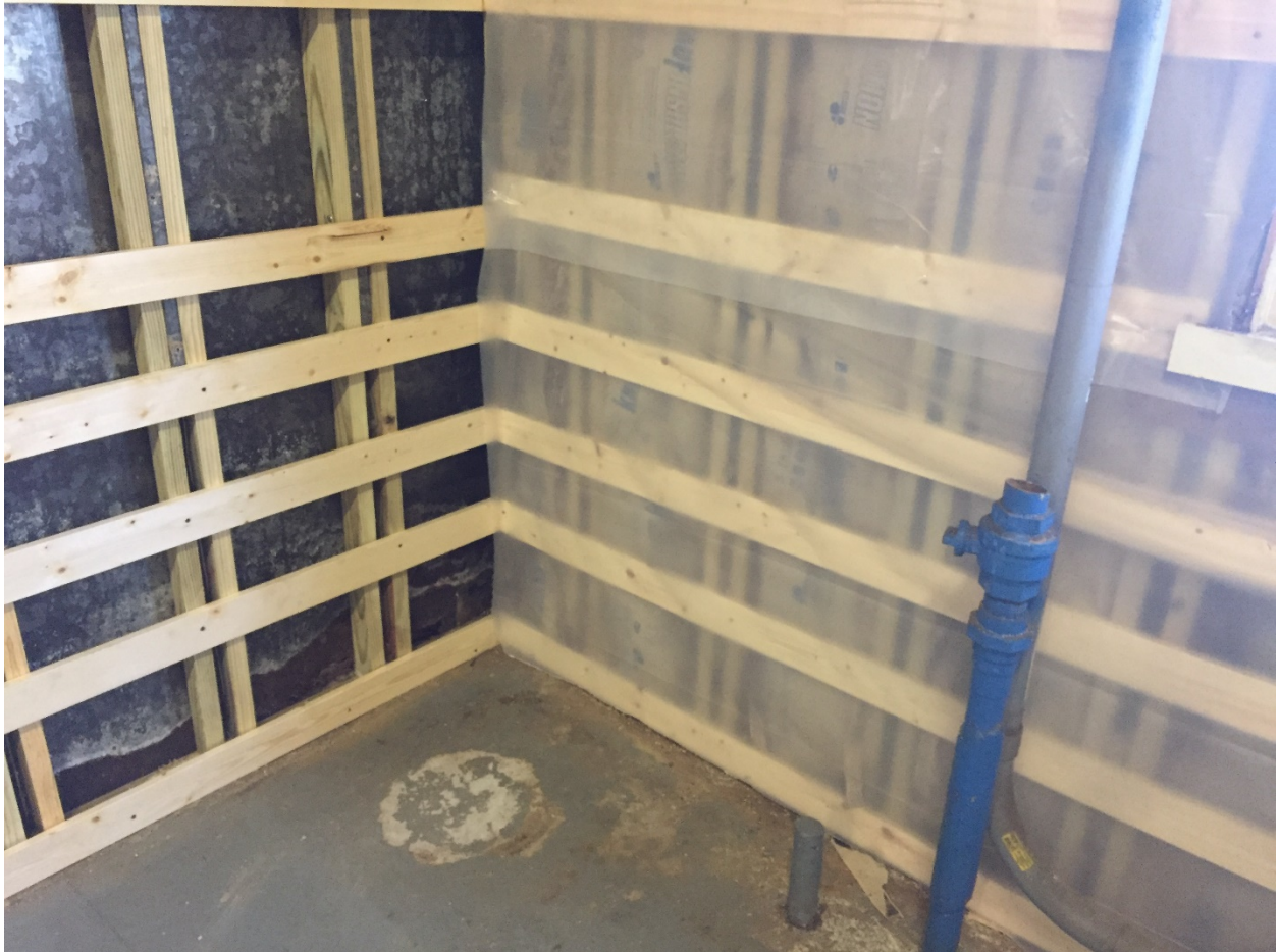
Exhibit 1-7: Photo of interior western wall reinforcement/repair
