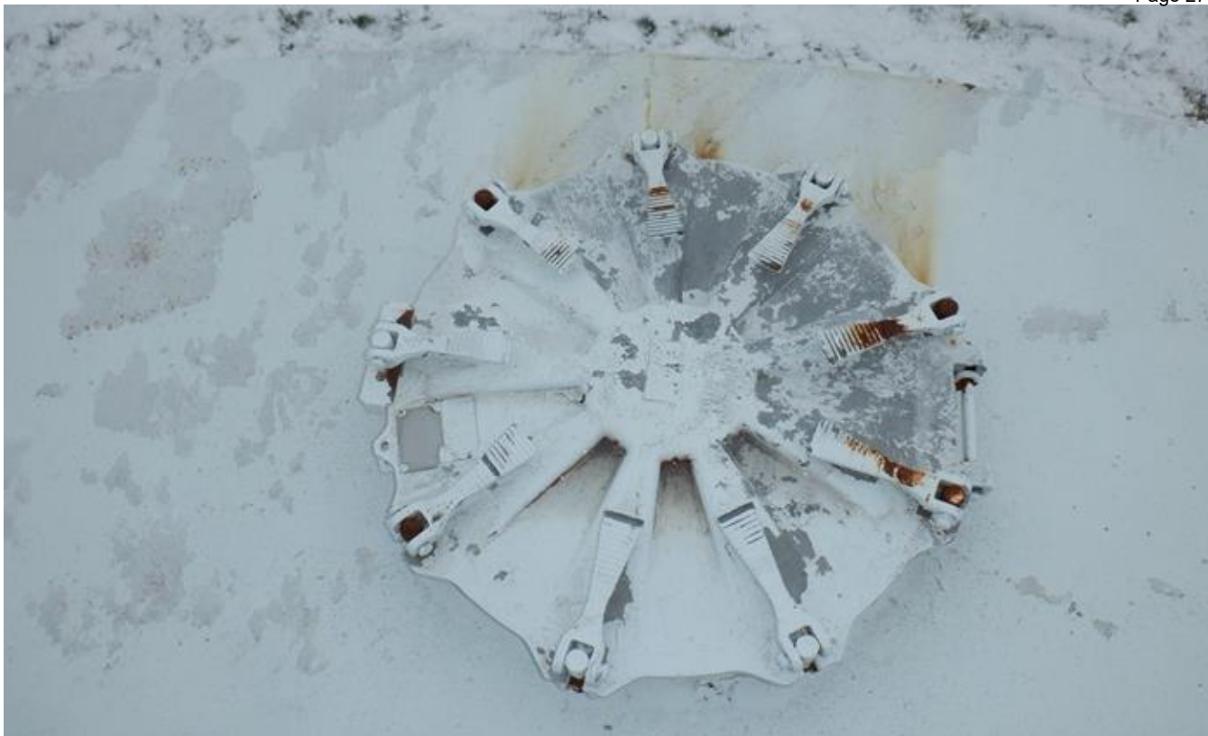
17. Roof manhole on bottom tank section roof.
