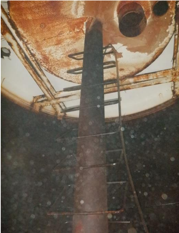
57. Inlet pipe, aerator effluent pipe, and interior roof of middle section.
