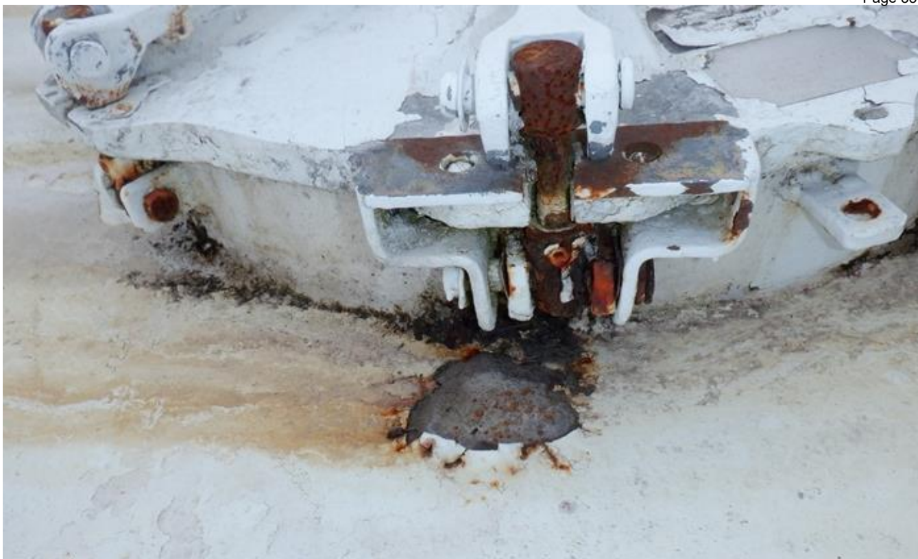
29. Corrosion on middle section roof manhole cover latch.
