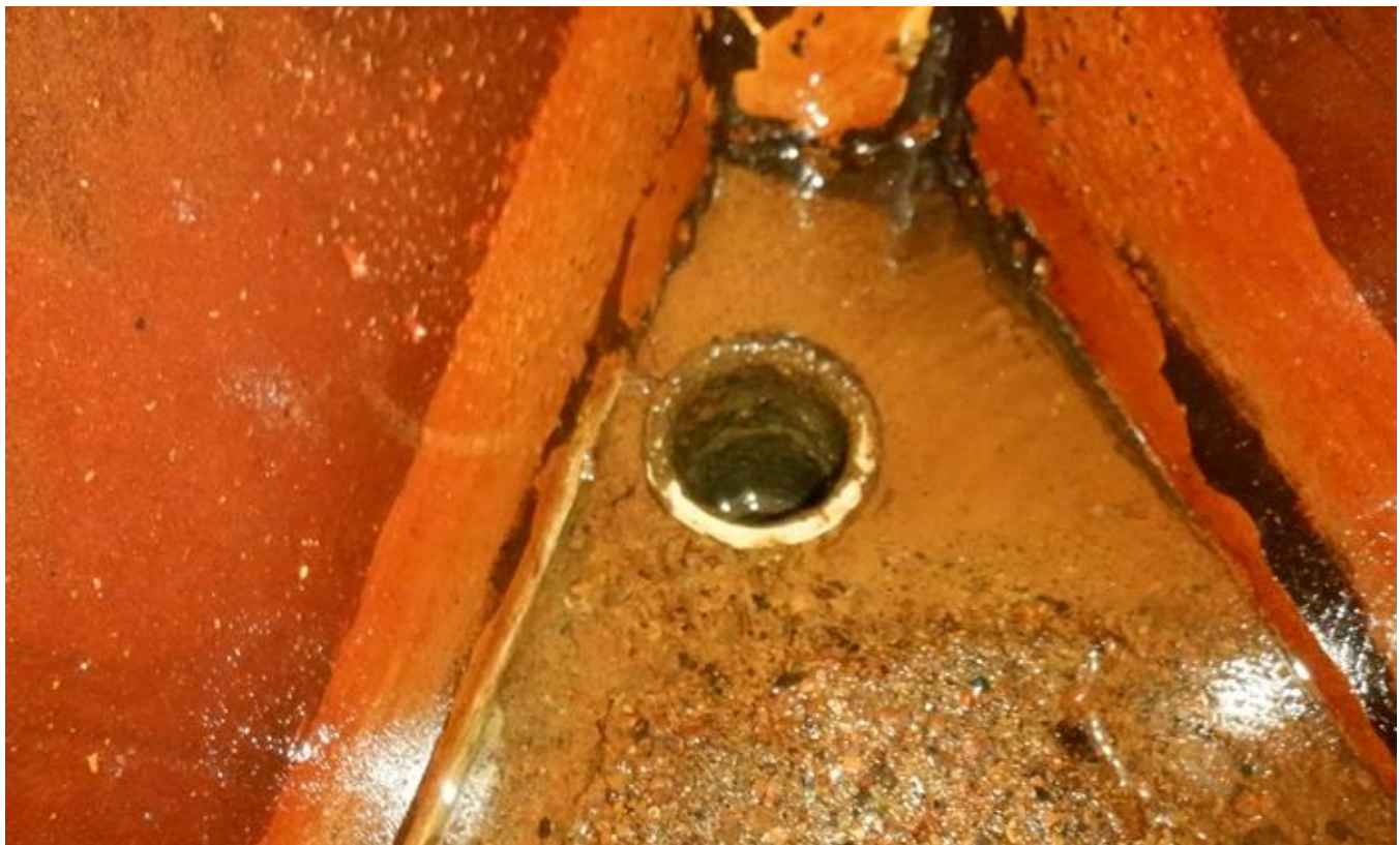
64. Pipe opening in middle tank section floor.
