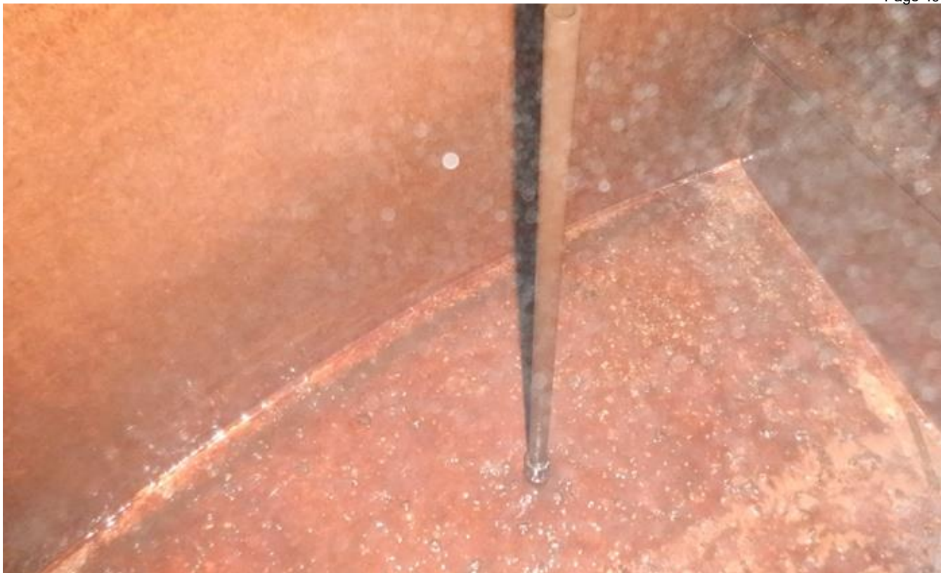
61. Pipe in bottom of middle tank section.
