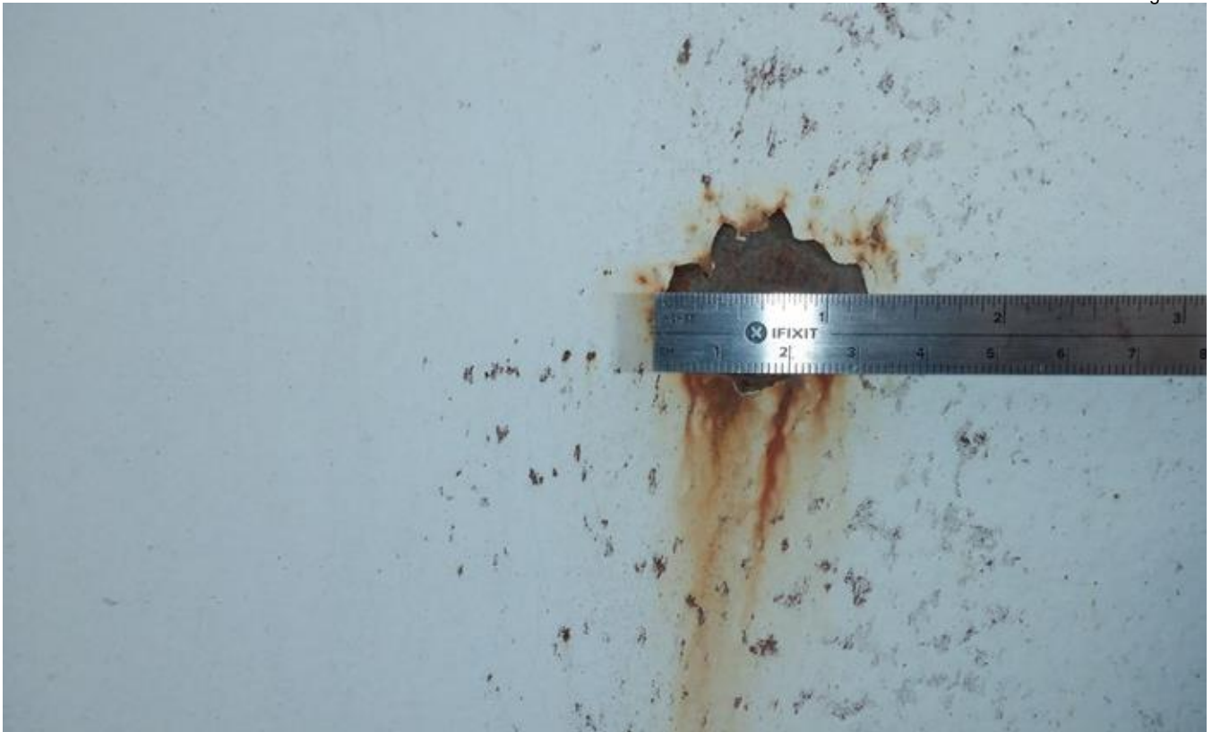
11. Coating failure and corrosion on shell coating.
