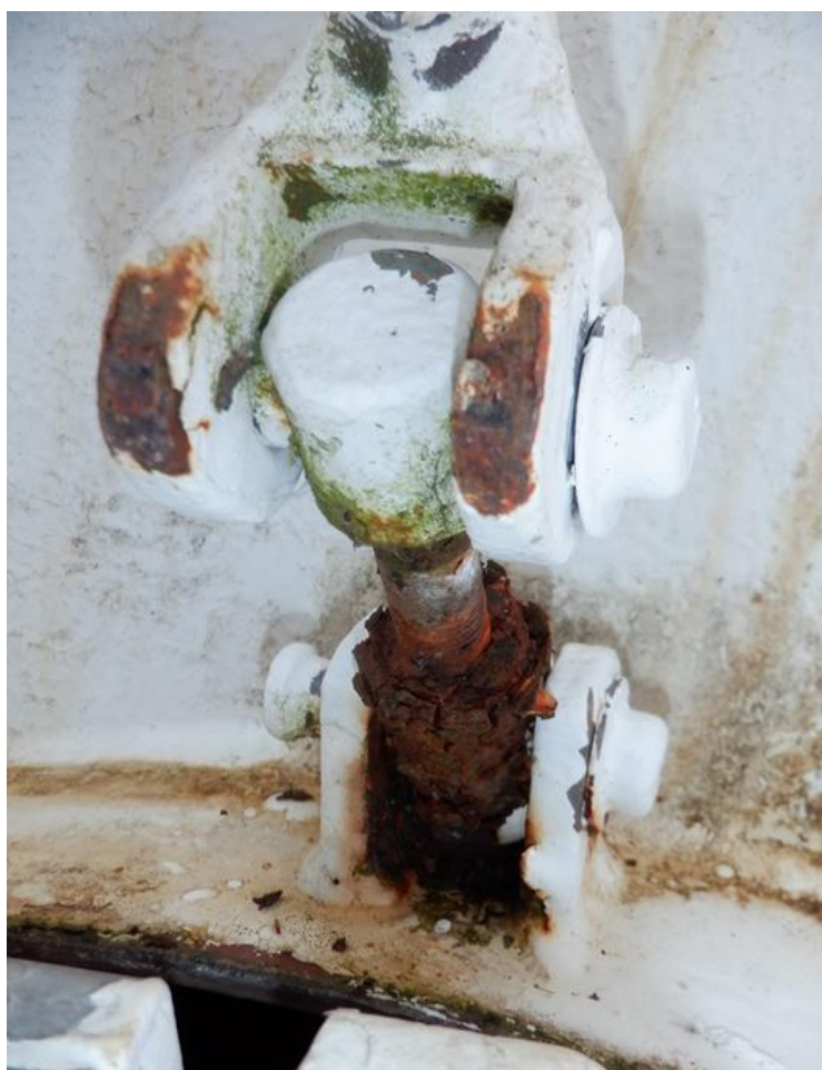
29. Corrosion on middle section roof manhole cover latch.
