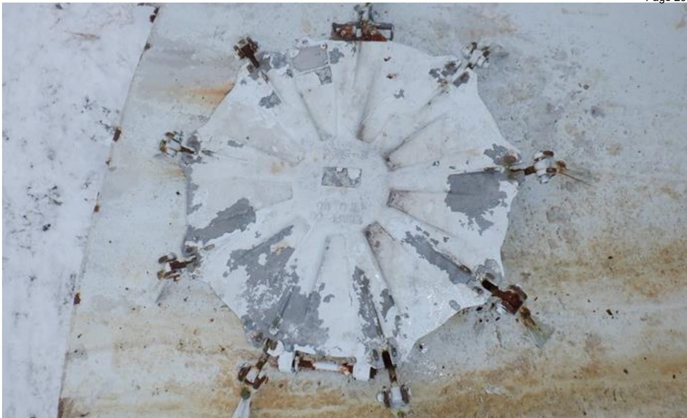
15. Roof manhole on bottom tank section roof.
