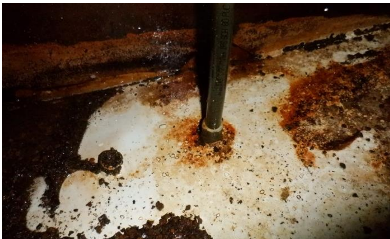
62. Pipe in bottom of middle tank section.
