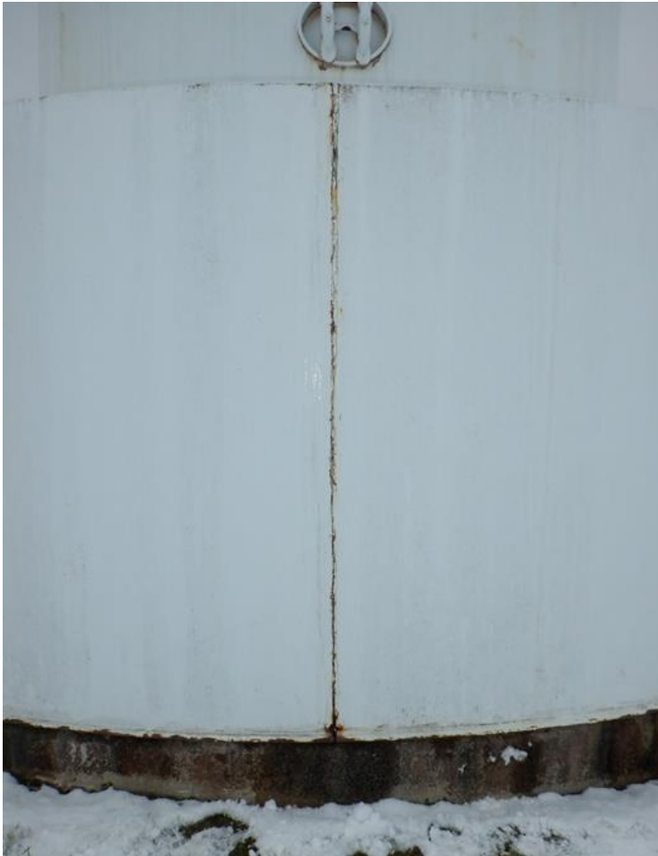
7. Vertical shell seam.
