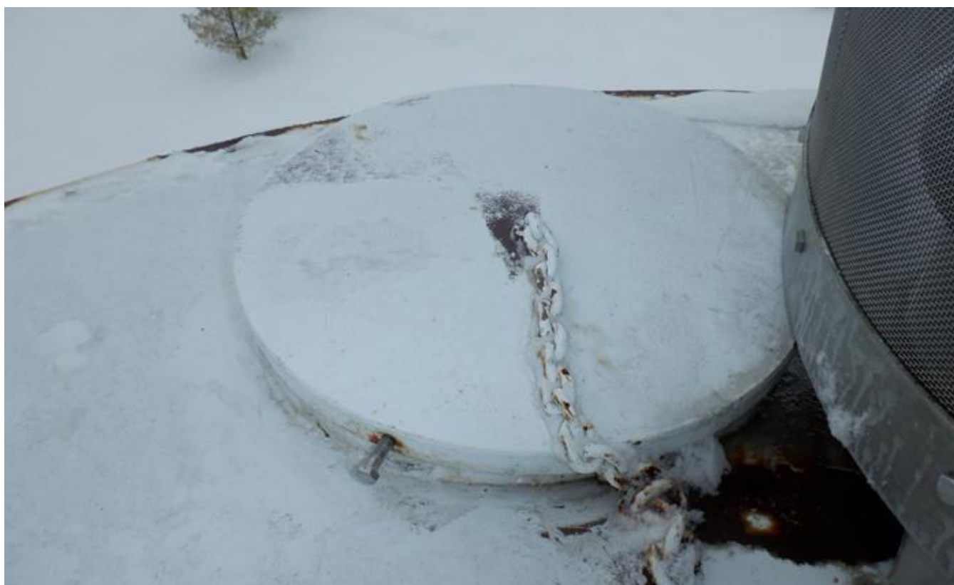
44. Top section roof manhole.
