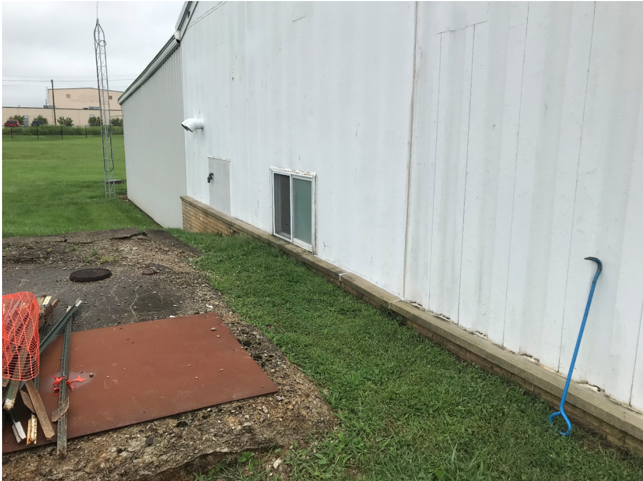
Exhibit 1-5: Photo from exterior of western wall
