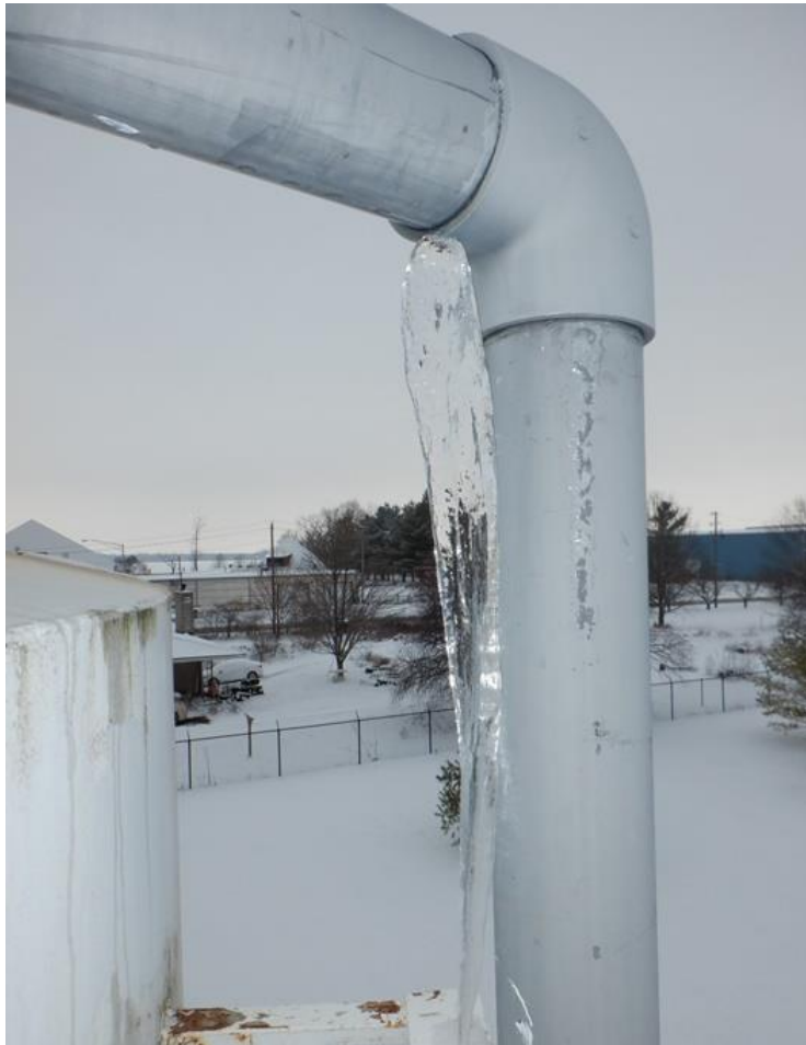
35. Overflow pipe projection and icicle.
