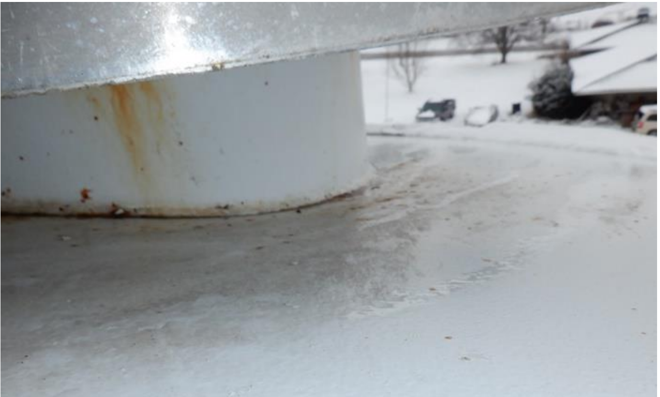
50. Blower-to-roof connection on top tank section roof.
