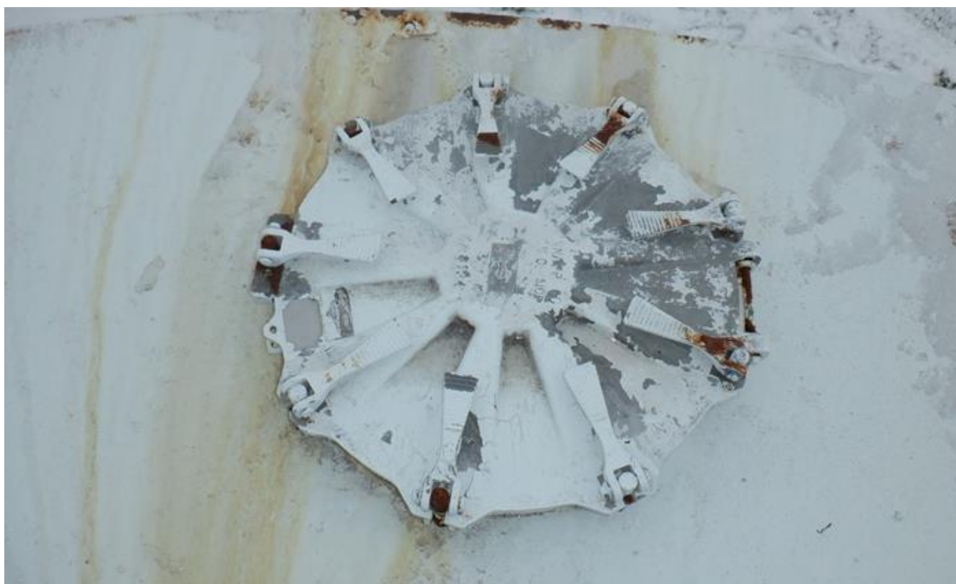
18. Roof manhole on bottom tank section roof.
