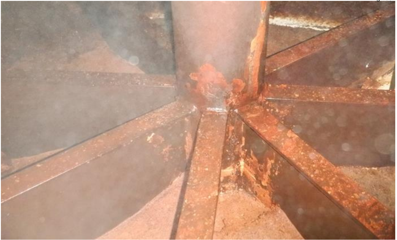
63. Inlet pipe and stiffeners at bottom of middle tank section.
