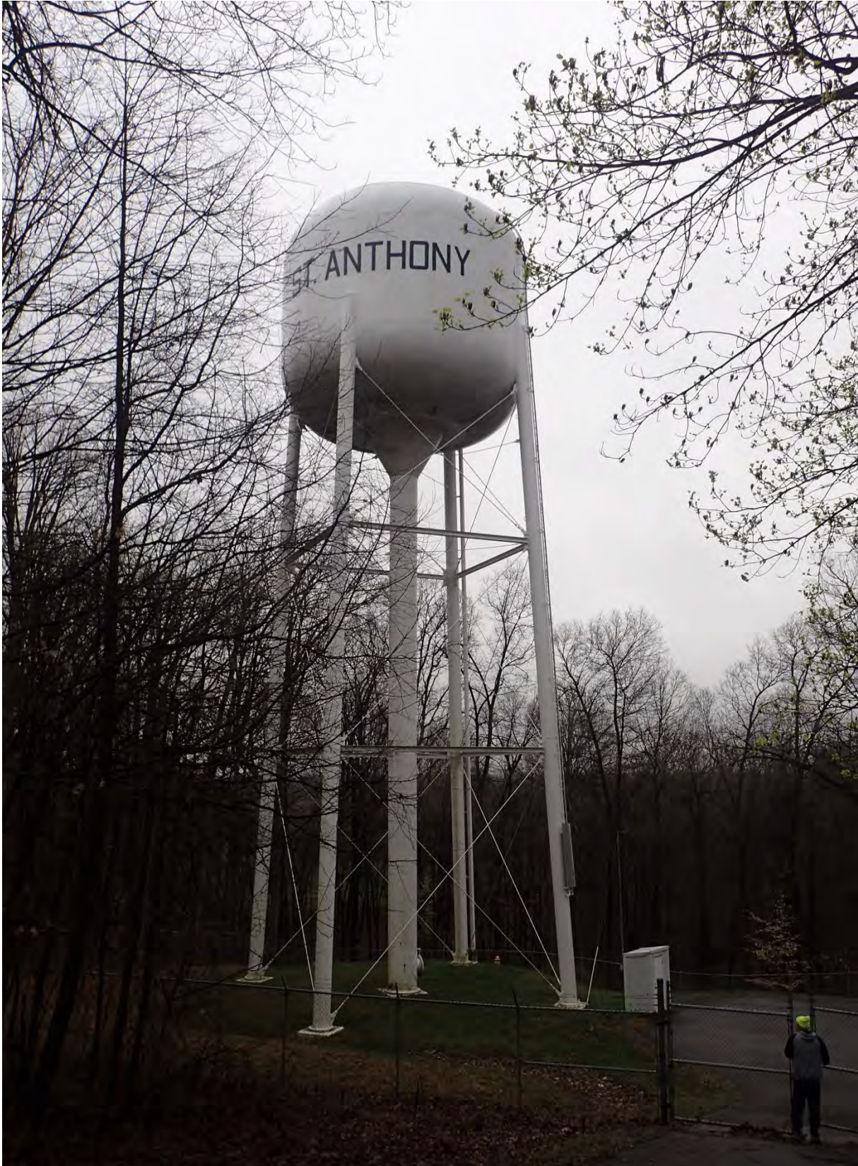
200,000 gallon elevated tank
