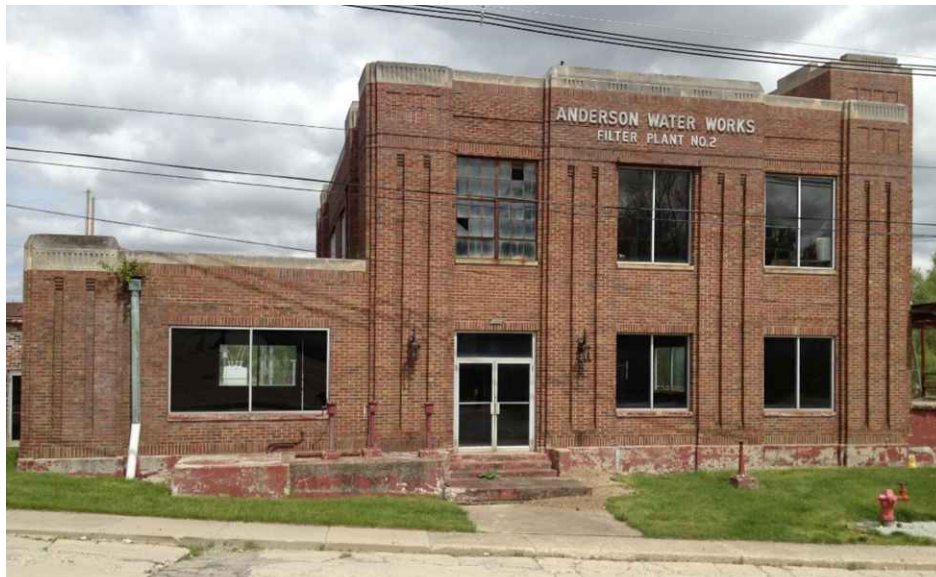
Figure 1.1.9 Abandoned Surface Water Treatment Plant Building
