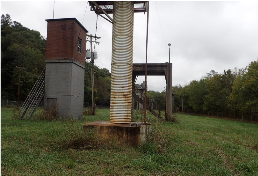
Figure 3 Elevated well platforms and Control Building
