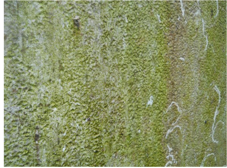
Figure 12 – Photo of corrosion pitting. Oct. 12, 2017
