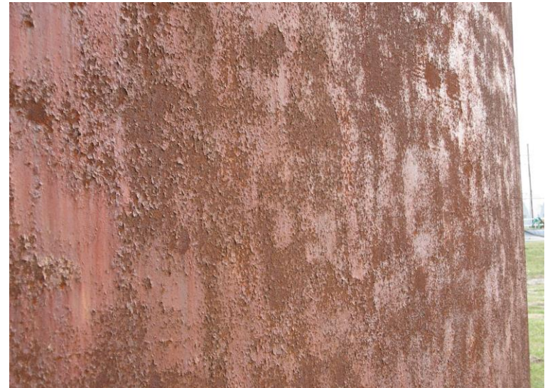
Figure 14 – 1.5 MG GST showing rust streaks. Photo taken in 2005.
