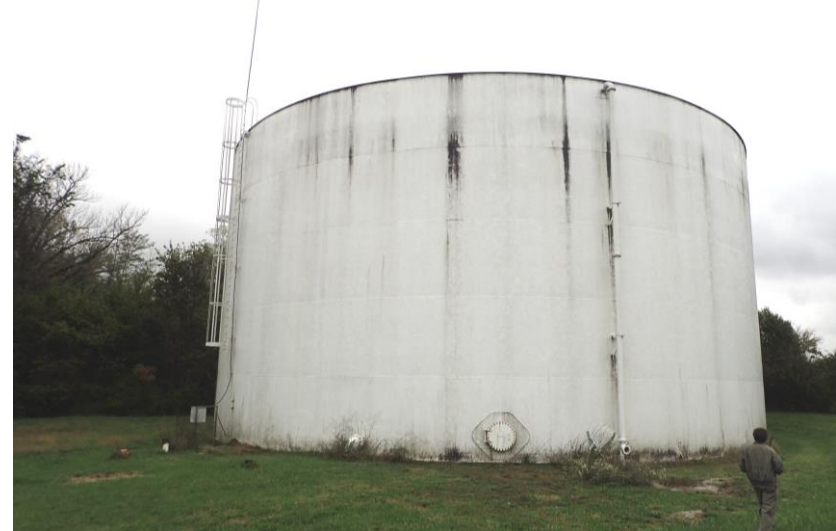
Figure 10 – 1.5 MG Ground Storage Tank showing manway and roof access ladder.
