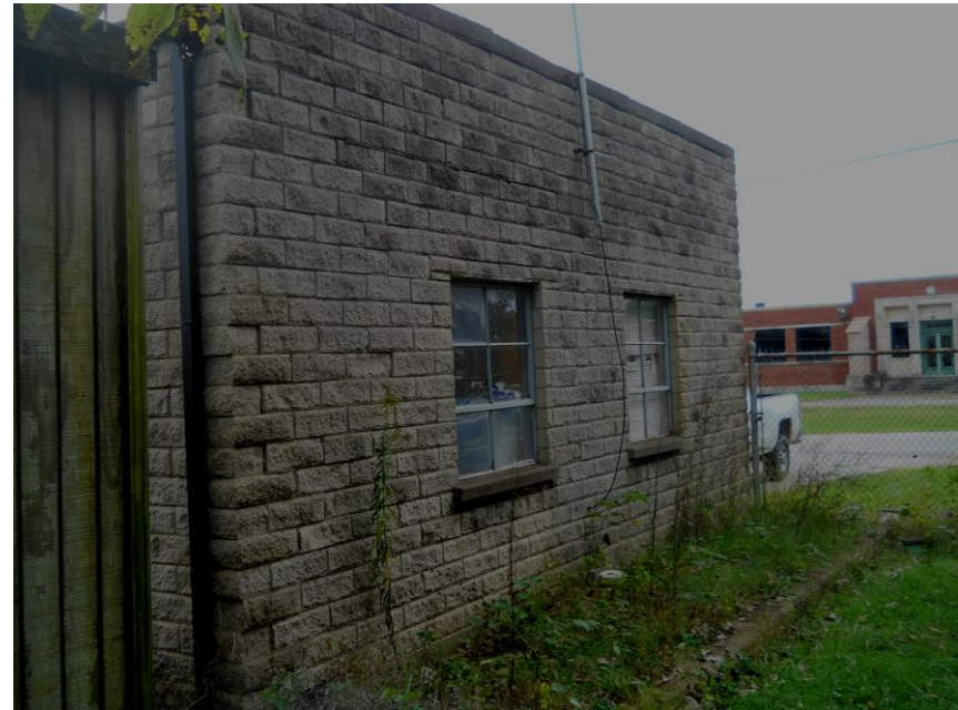
Figure 2 Pump Building – view of north side.
