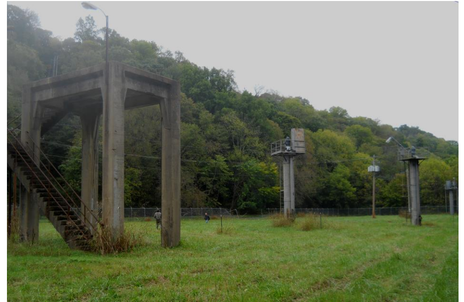
Figure 2 Elevated well platforms and concrete platform (abandoned)
