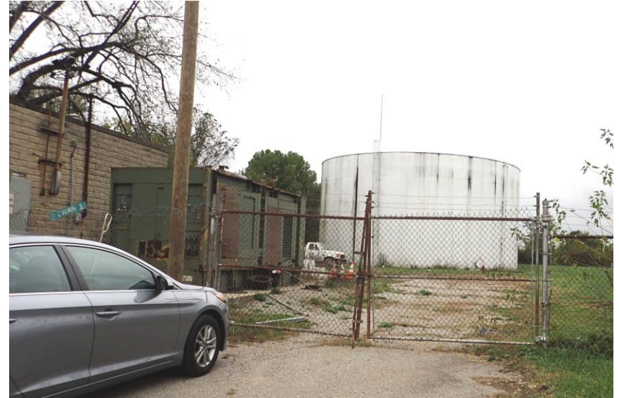
Figure 8 – 1.5 MG GST & Pump Bldg. Oct. 12, 2017 photo.
