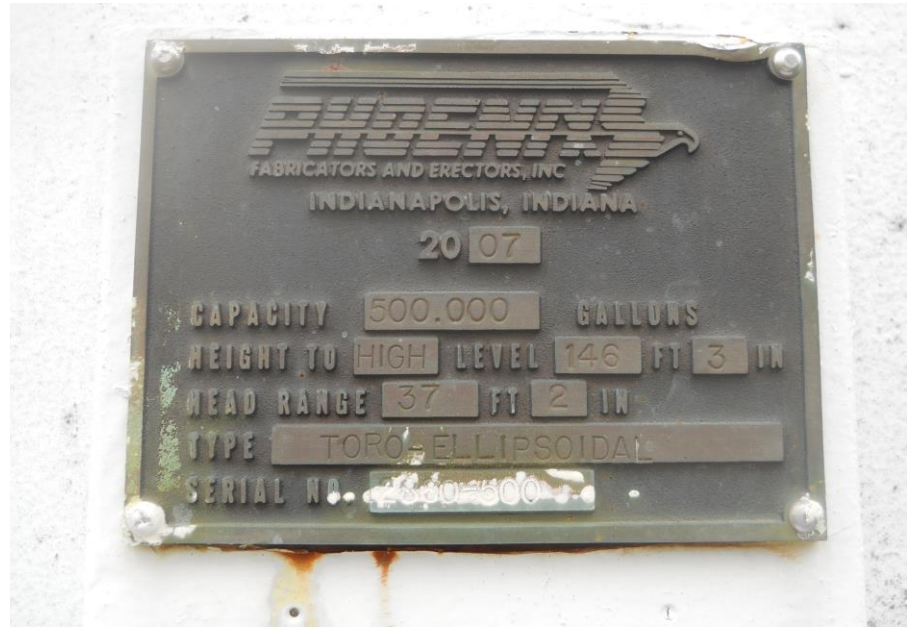
Figure 4 2007 Manufacturer plate – Phoenix Fabricators, Indpls., IN
