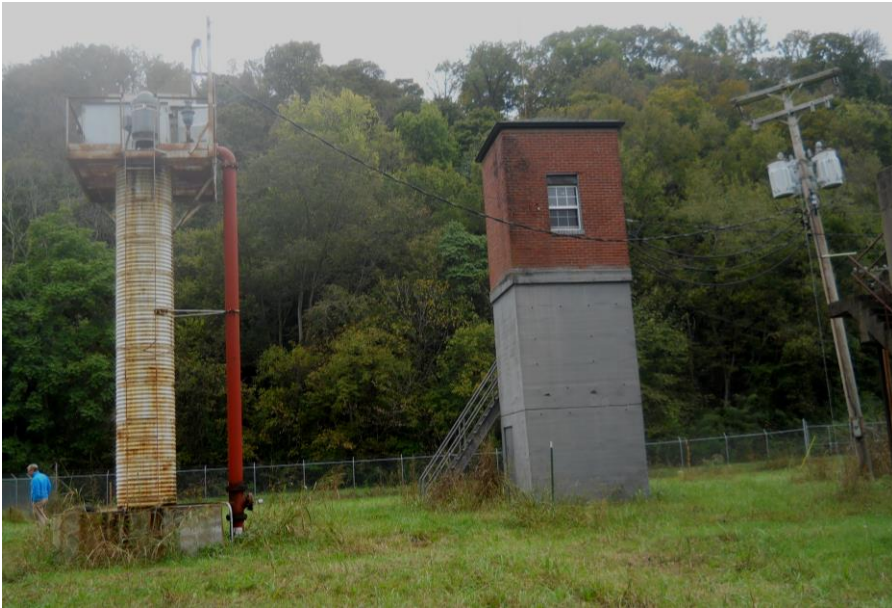
Figure 1 Wellfield – view of elevated well and Control Building
