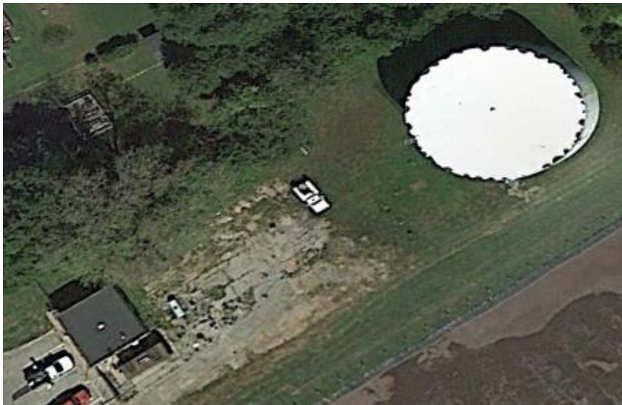
Figure 5 – September 2013 – Aerial of Charlestown’s Pump Building and 1.5 MG Ground Storage Tank showing the tank roof rust pockets at the roof-wall interface.
