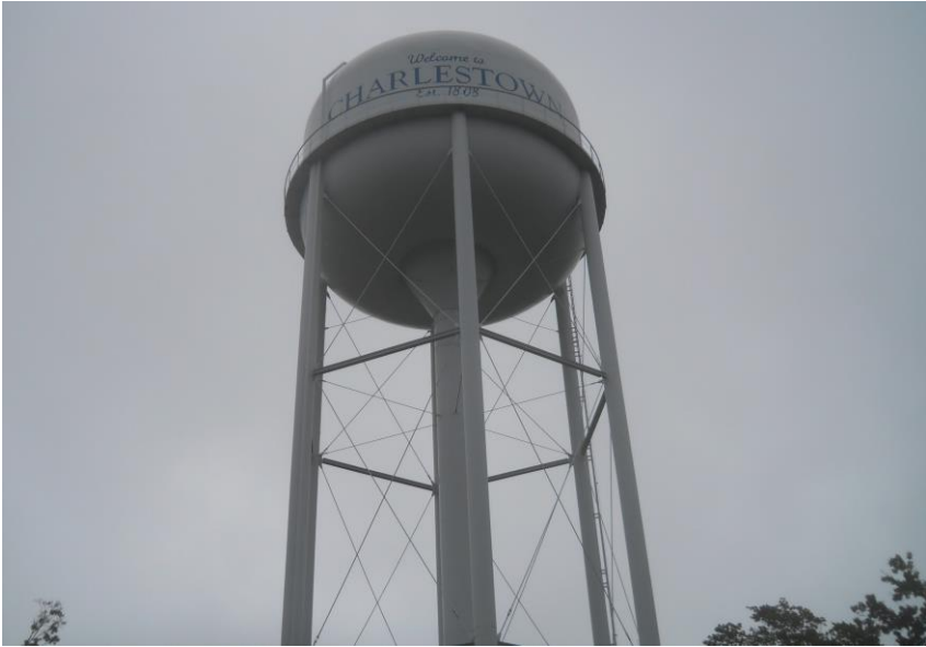
Figure 1 Elevated Water Tank (10/12/17 photos)
