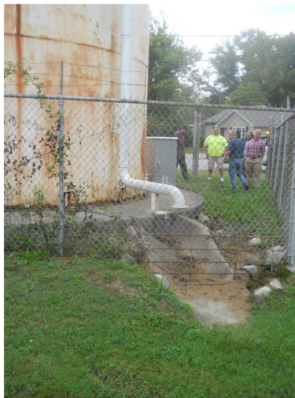
Figure 4 Standpipe overflow pipe.
