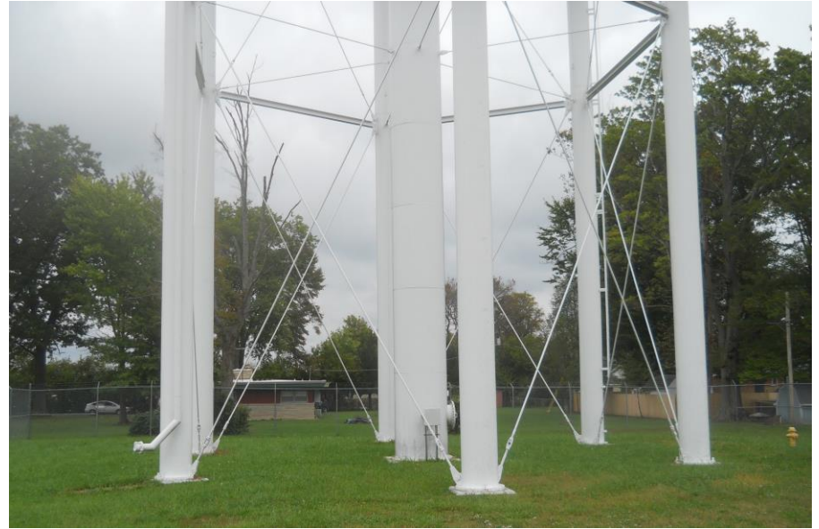
Figure 2 Elevated Water Tank – multi-column legs and fill pipe.
