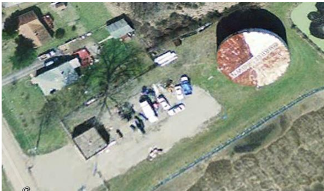
Figure 2 - March 2005 – Aerial of Charlestown’s 1.5 MG Ground Storage Tank showing extensive rusting of the roof steel.
