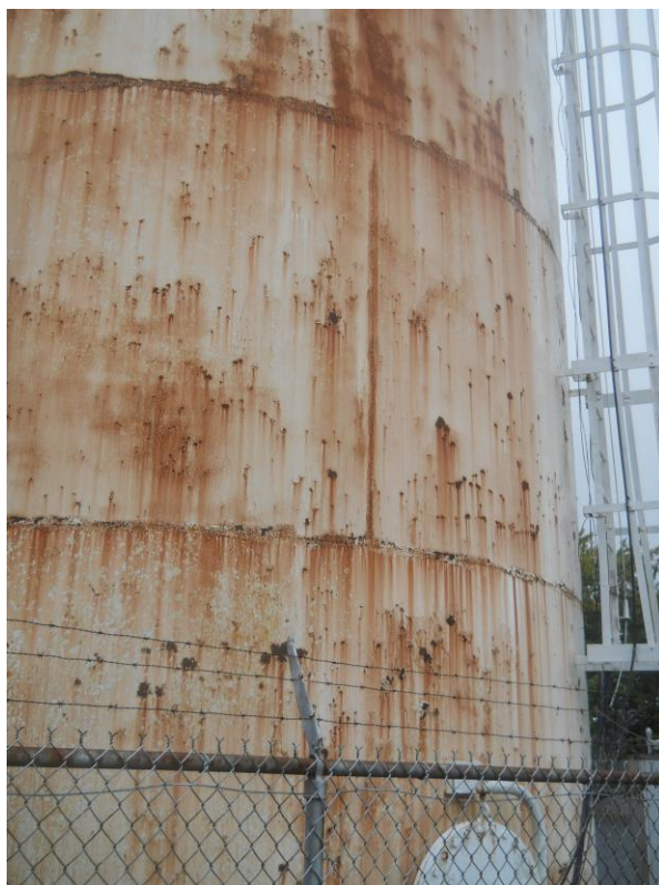
Figure 3 Standpipe rust.
