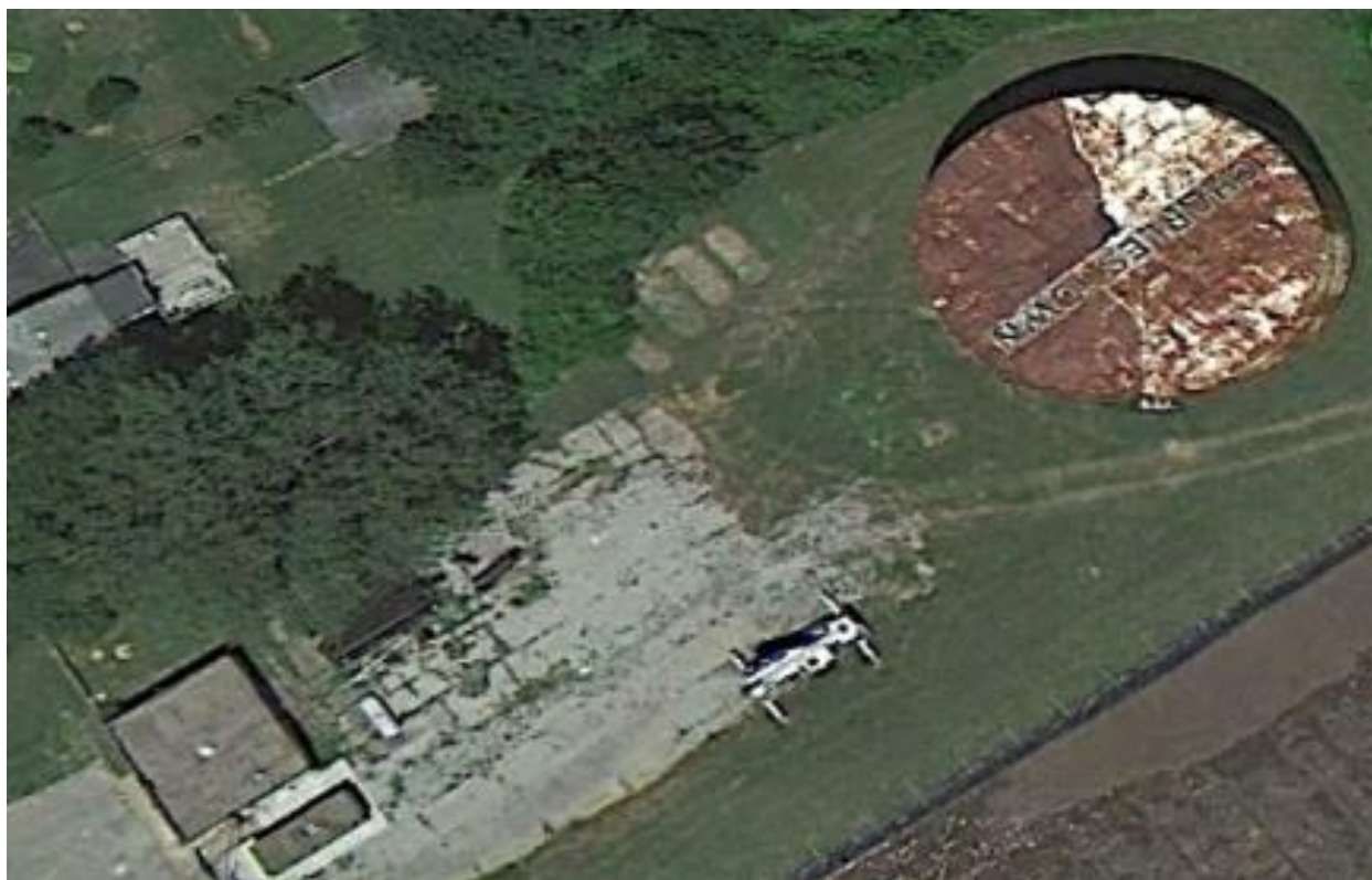
Figure 3 – June 2010 – Aerial of Charlestown’s 1.5 MG Ground Storage Tank showing the progression of roof rusting. Note the standby generator south of the Pump Building (lower left).
