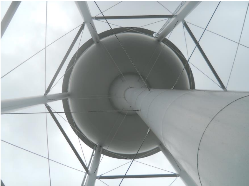
Figure 3 Elevated Water Tank – view from underneath
