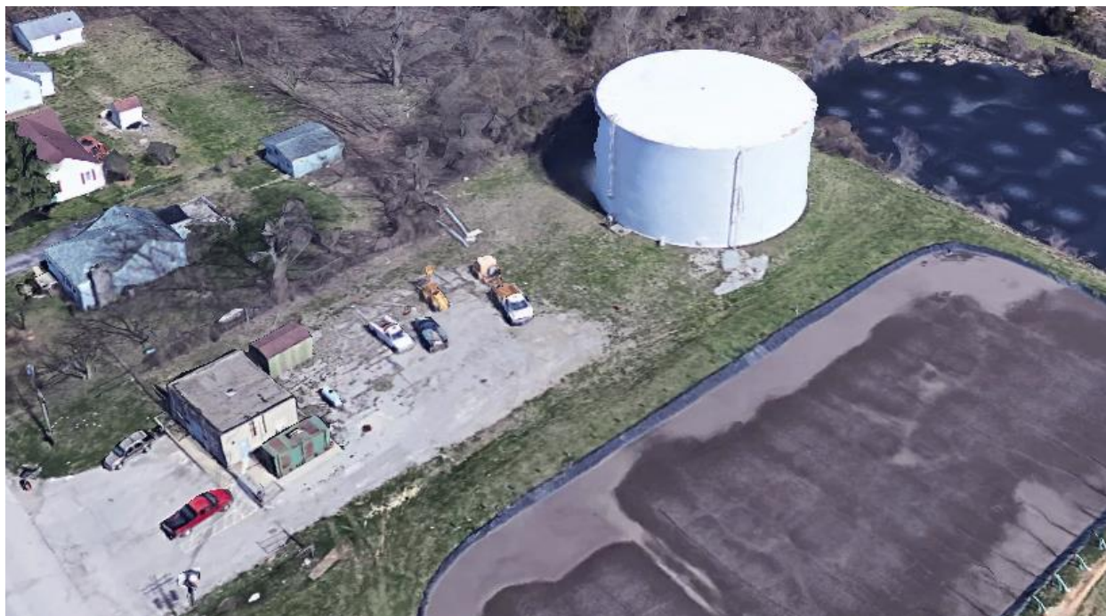
Figure 6 - September 2016 – Oblique view of Charlestown’s 1.5 MG Ground Storage Tank showing the repainted tank, Pump Building, and standby (nonfunctioning) generator (lower left).
