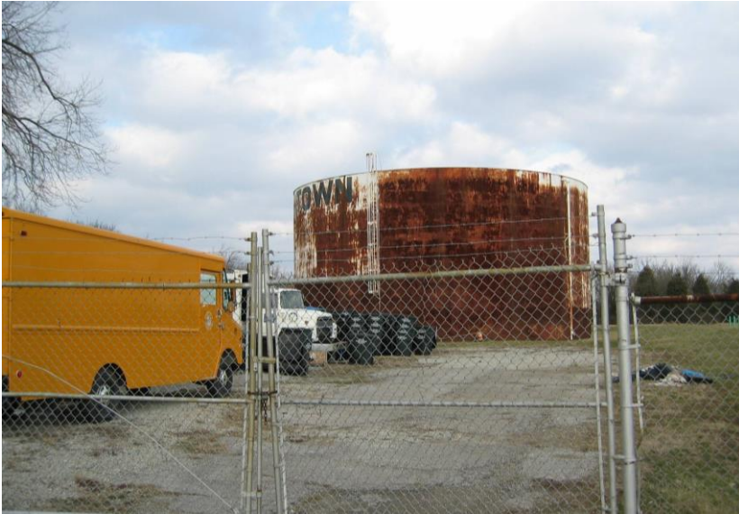
Figure 7 – 1.5 MG Ground Storage Tank. Photo taken in 2005.
