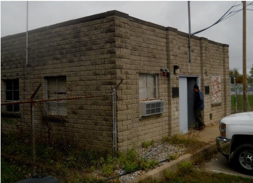
Figure 1 Pump Building entrance (10/12/17 photos)
