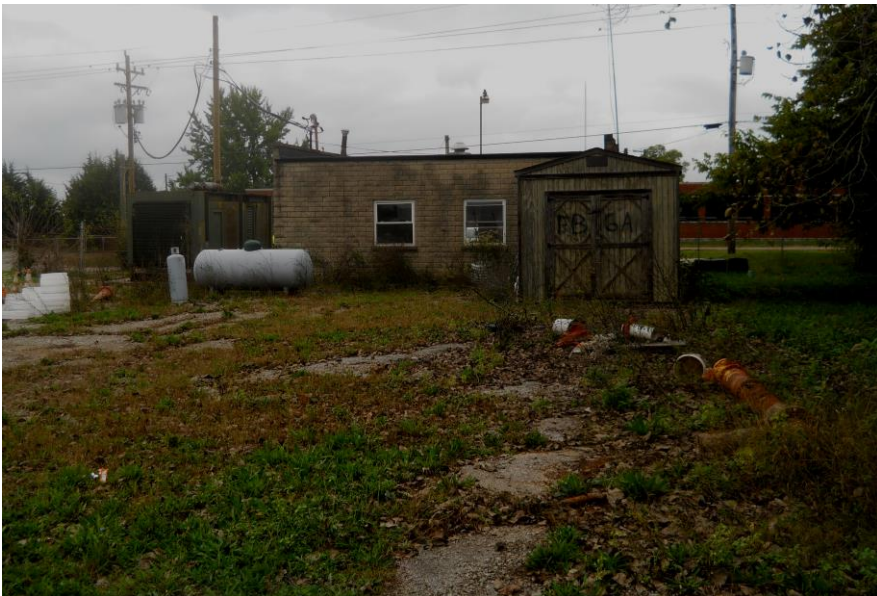
Figure 3 Pump Bldg – view from the east side. Generator is at left.
