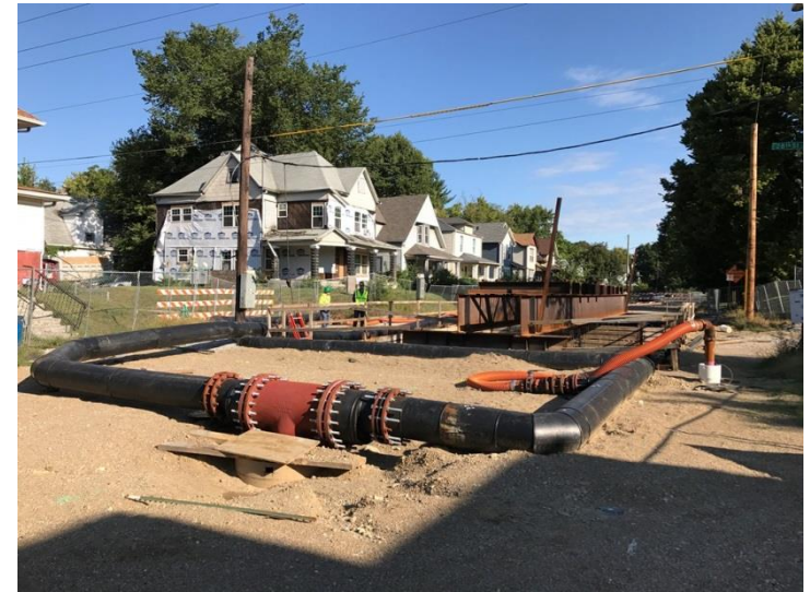
Capitol Ave. & 28 th St. Excavation Support and Sewer Bypass
