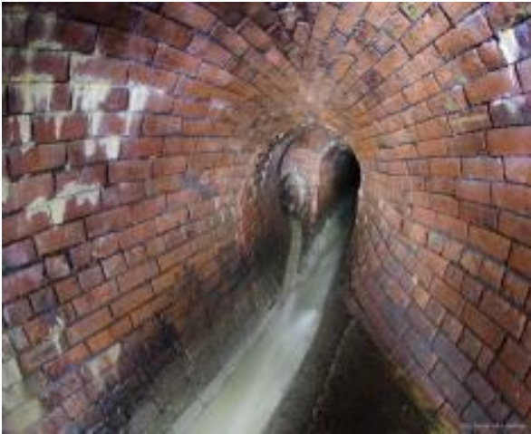
Brick Sewer Pipe, 1800's – 1950's
