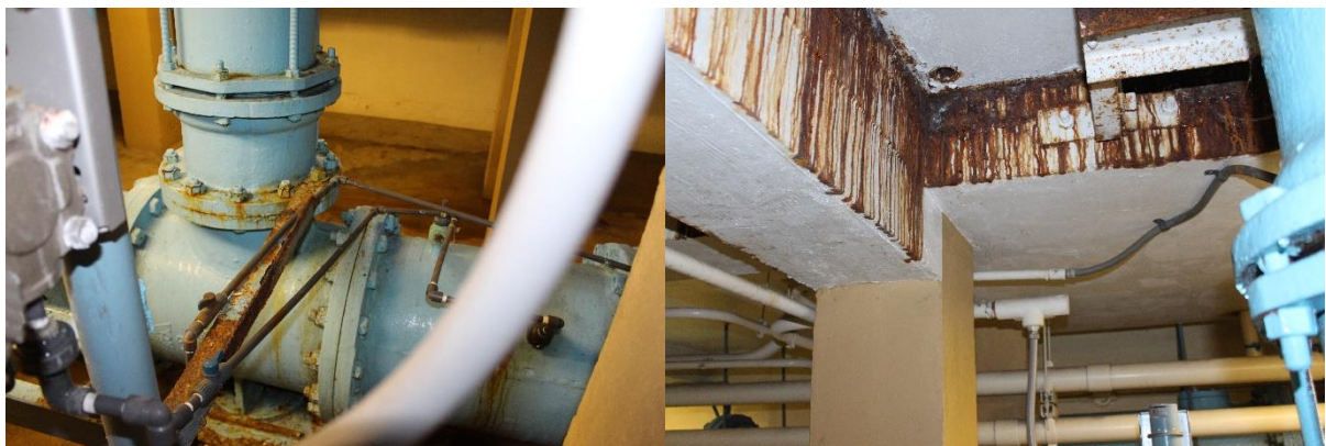
FIGURE 5. CLEANING AND COATING WORK NEEDS
