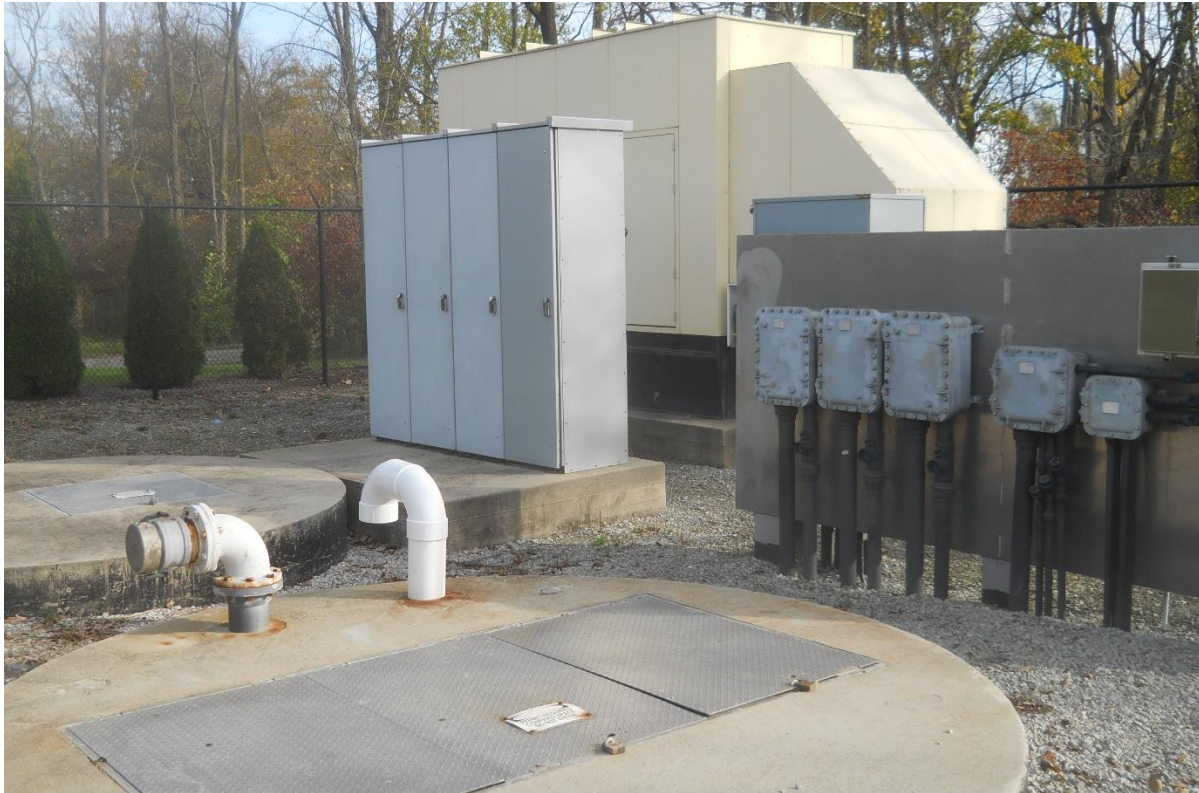
Photo 3 – View of the Washington Woods Lift Station constructed in 2007 and upgraded in 2016. The standby generator is in the background (tan structure).
