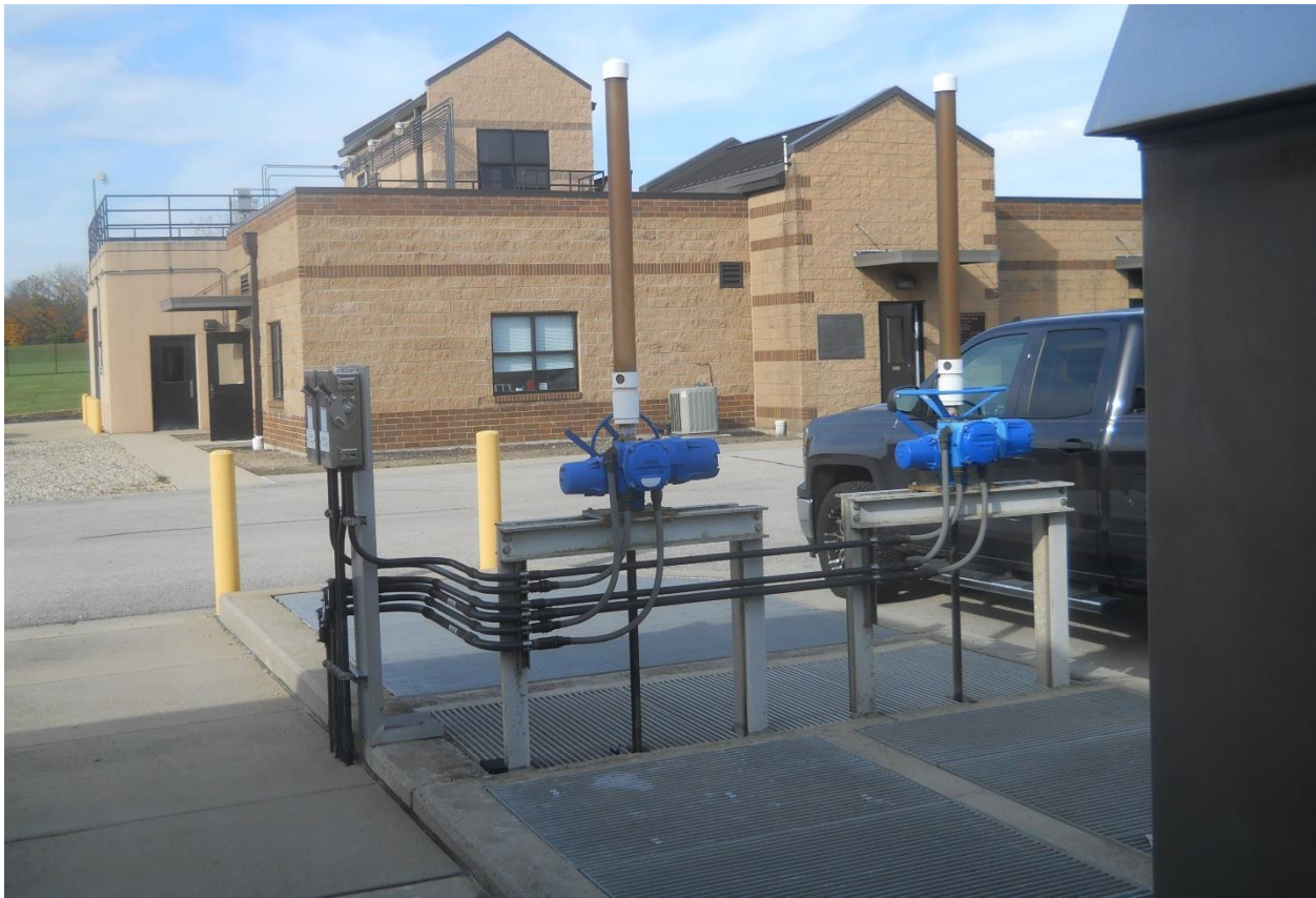
Photo 9 – View looking west of the Westside wastewater treatment plant showing the influent channels to the UV disinfection system.
