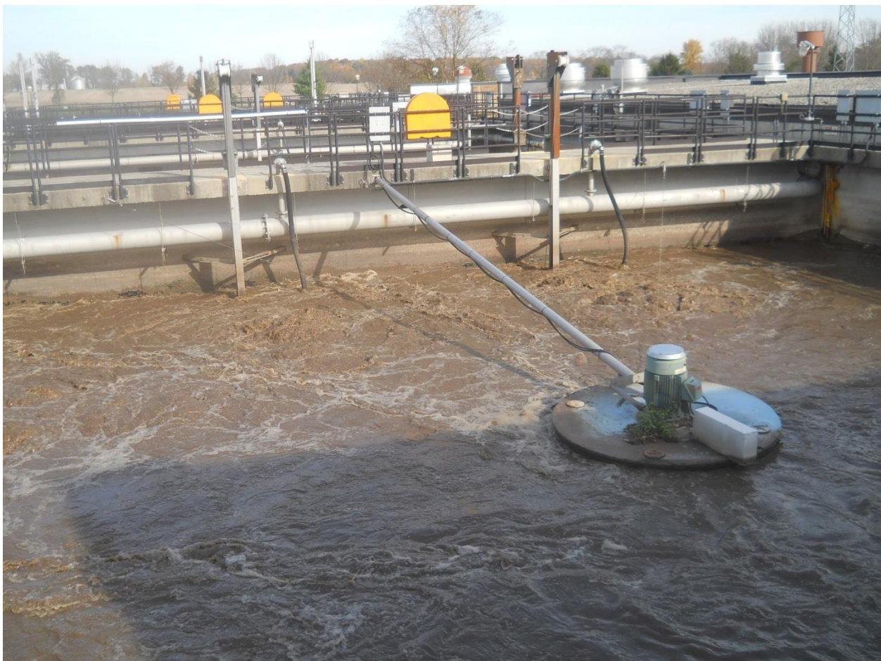
Photo 12 – Aeration and mixing sequence in the Sequencing Batch Reactors showing the floating mixer, aeration drop headers.
