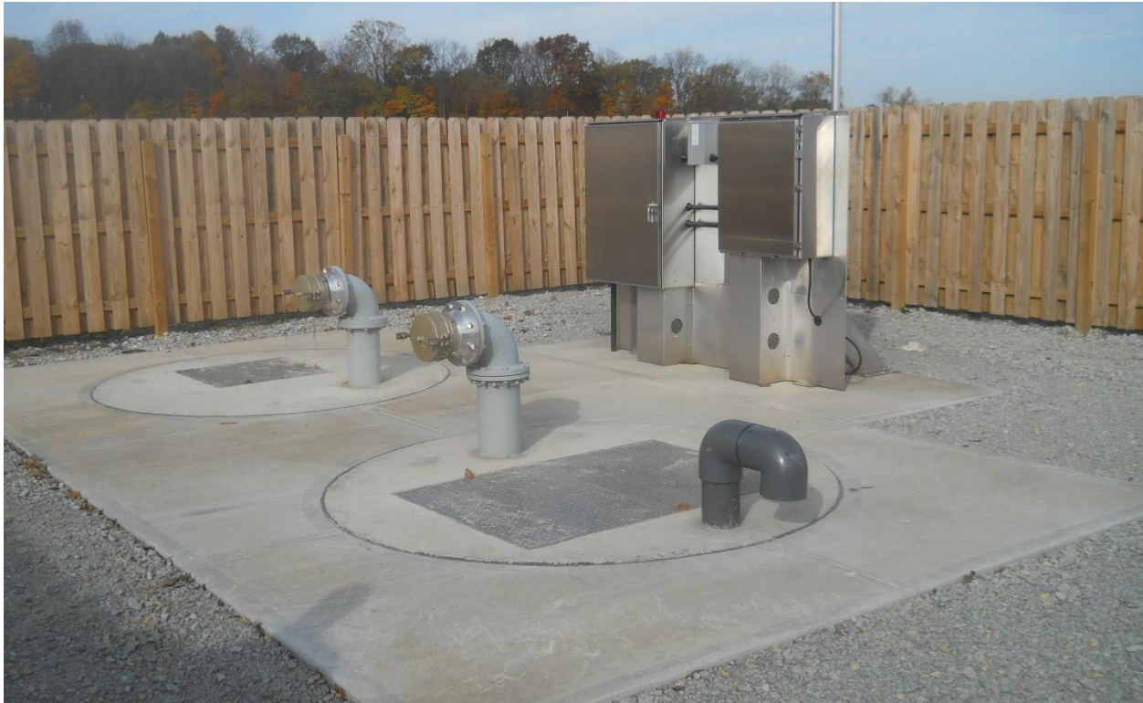
Photo 7 – View of the 156 th Street Interceptor temporary Lift Station installed in 2016.
