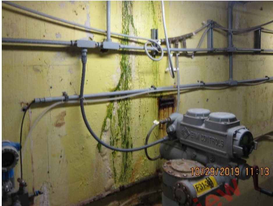
FIGURE 2-12 Flexible Cables
