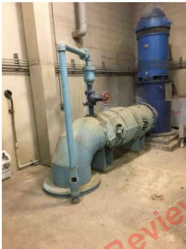
FIGURE 2-28 High Service Pump Station No. 3
