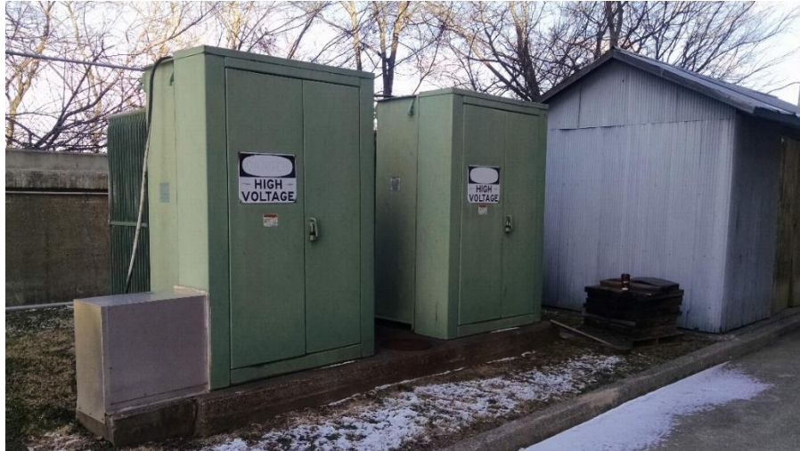
FIGURE 2-8 LSPS Transformer
