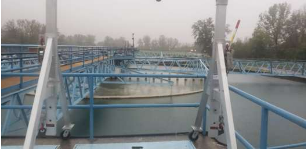
FIGURE 2-9 South Plant Primary Settling Basins
