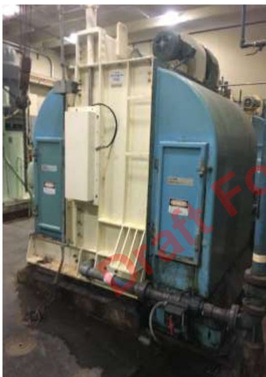
FIGURE 2-1 Traveling Screen
