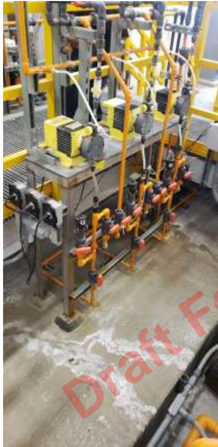
FIGURE 2-17 Coagulant Chemical Feed System
