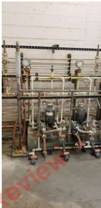
FIGURE 2-21 Fluoride Feed System
