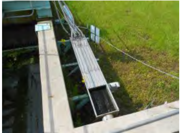
Ultraviolet Disinfection Unit
