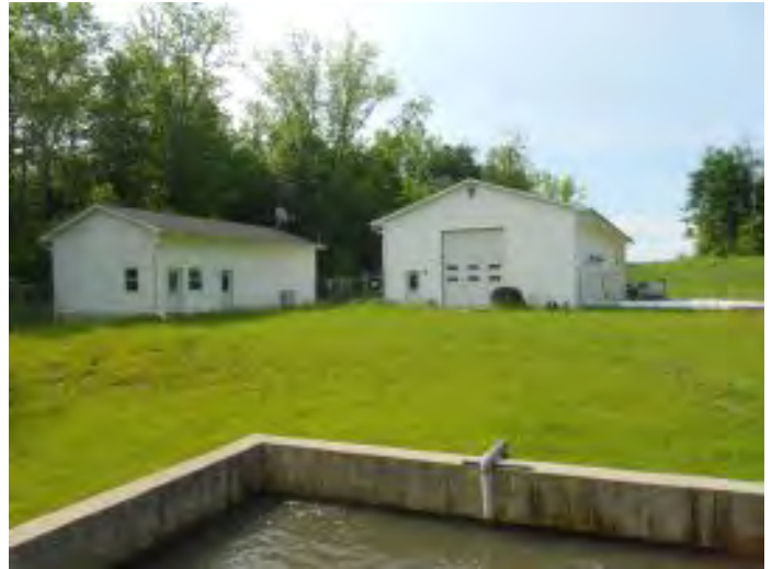
Looking southeast towards Control Building and Blower Building
