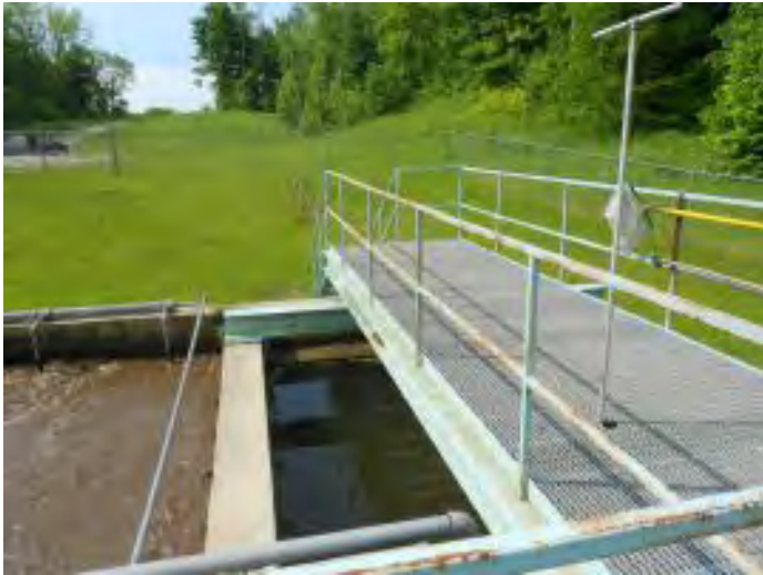
South Secondary Clarifier Under Walkway (One of Two)
