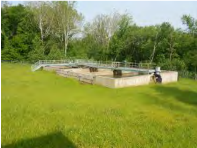
Looking northwest towards WWTP
