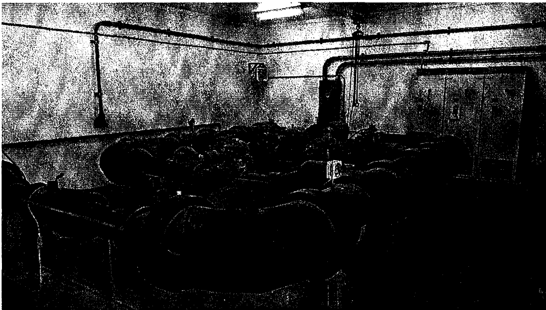
Photo 4 - Booster Pumping Station Interior, Showing High Service Pumps, Suction and Discharge Piping, Pump Control Valves, and Variable Frequency Drives
