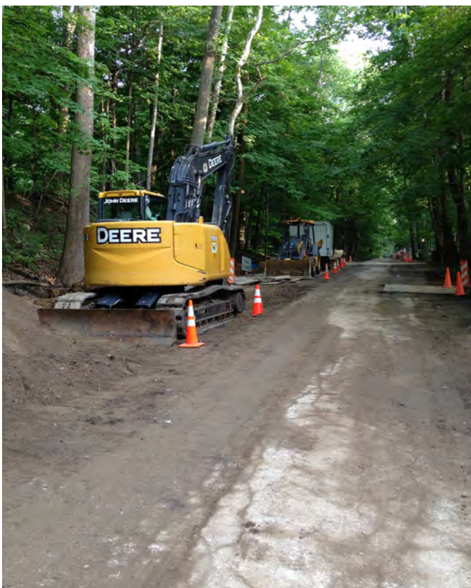
Above: Street view of a typical STEP construction site.
