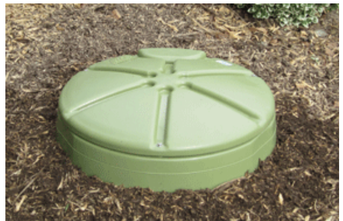
Surface View (post-installation)
