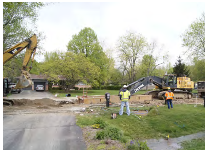
Typical Construction Area
