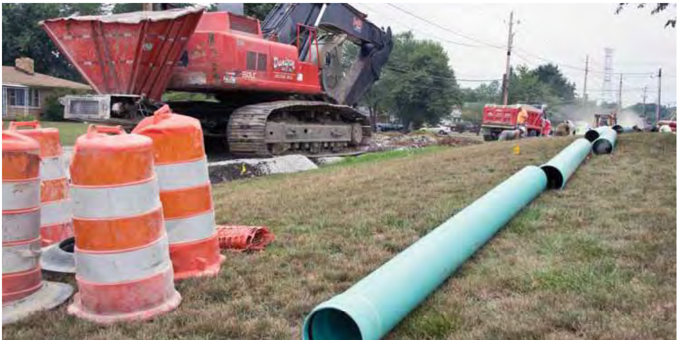
Construction continues on the Five Points and Southeastern STEP project.
