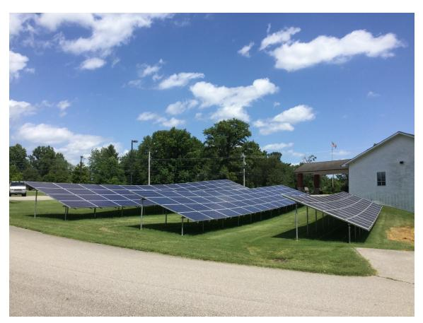
The specifications were for a system that would produce between 80-90% of the annual energy usage. The selected system was 54.4 kW. Electrical cost savings have dropped the previous electricity expenditure of about \$12,000/year to approximately \$4,000/year. The three (3) ground arrays have averaged 69,100 kWh/yr. I have personally monitored this solar system since its inception and prepared reports for our "Green Team" and members of the congregation.
