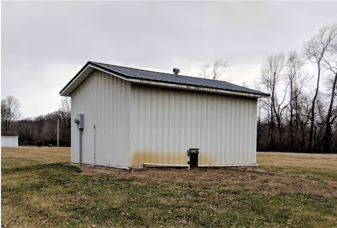
North well house exterior
