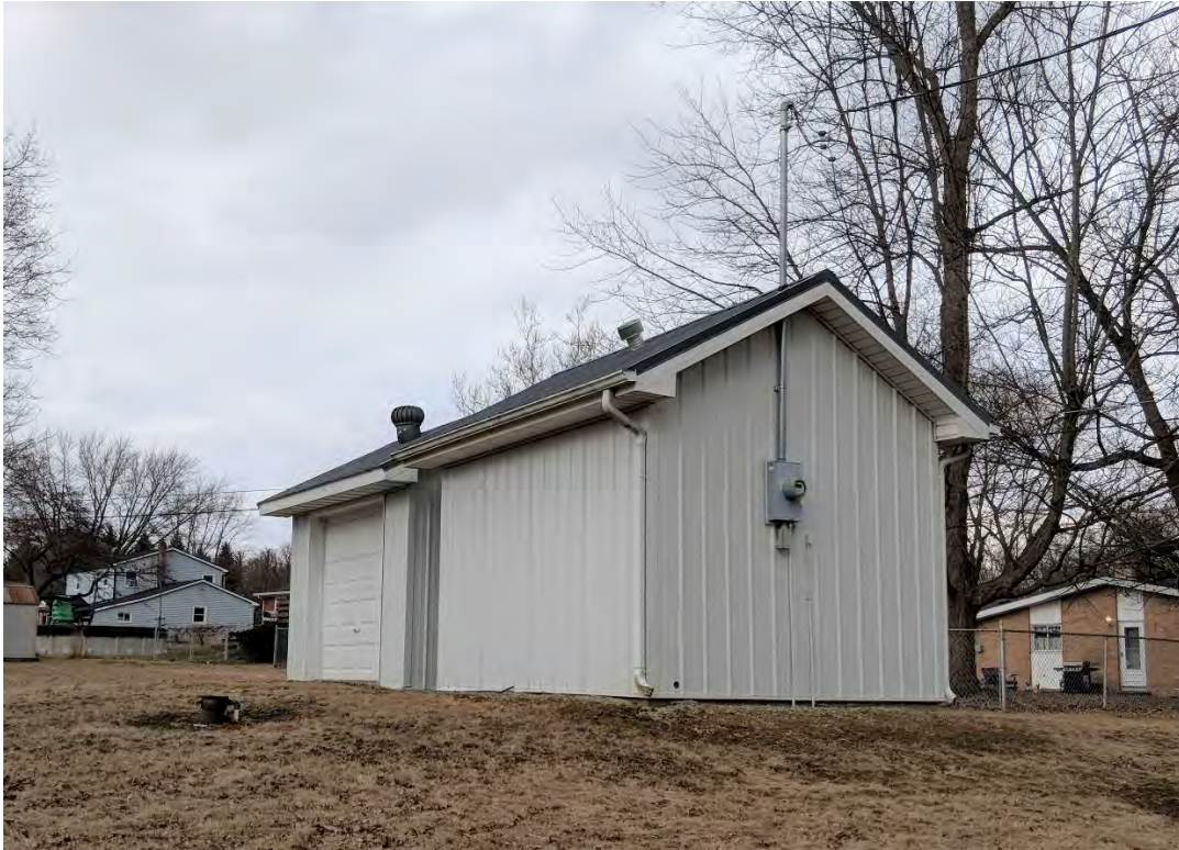
South well house exterior
