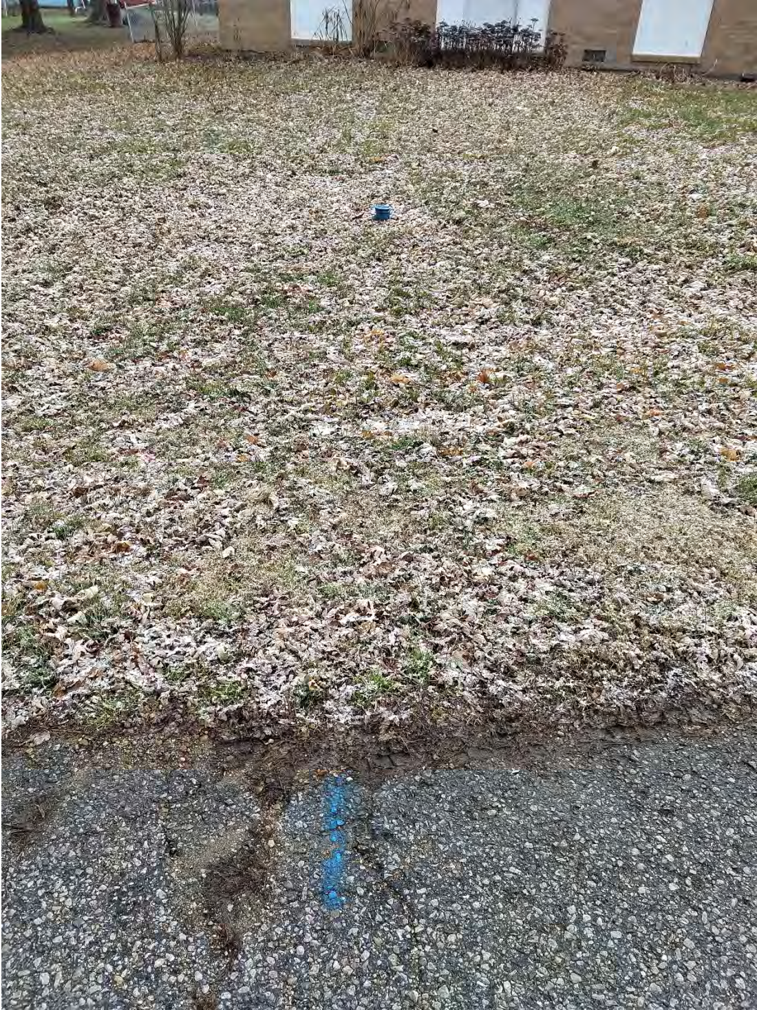
Example of service line, riser marking at residence. This is useful when trying to locate valves for emergency shut-offs.
