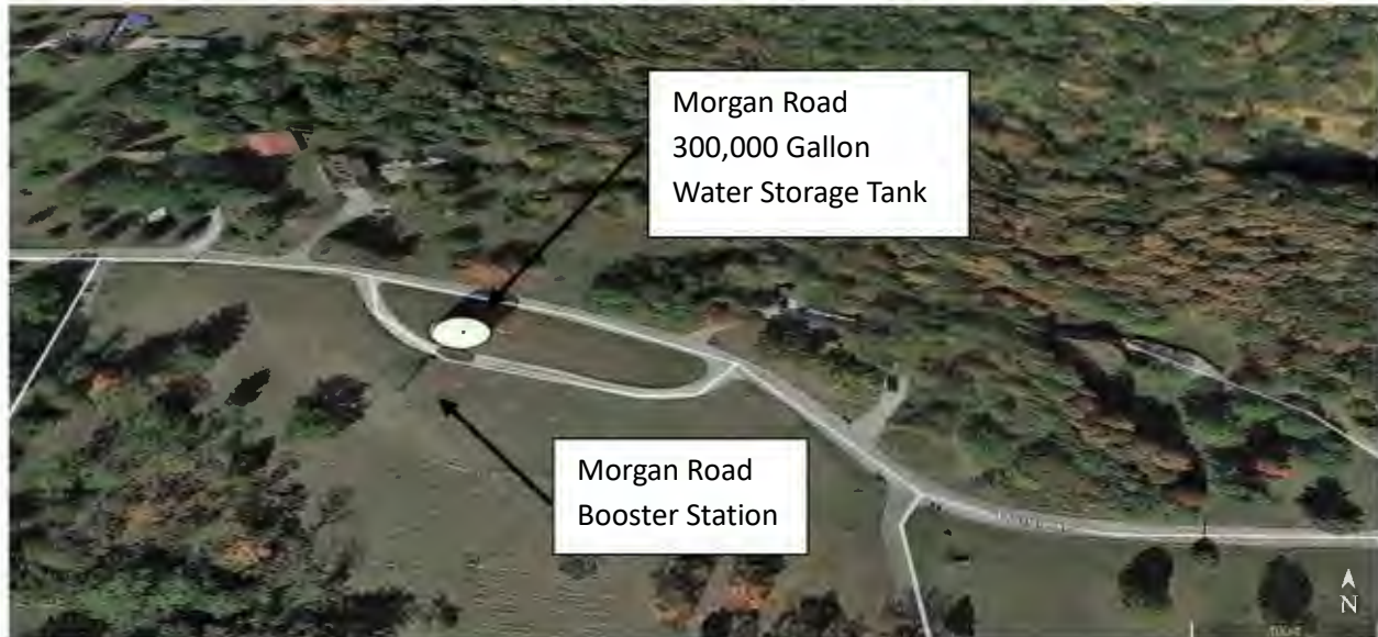
Figure 2.8.3 Existing Morgan Road Booster Station & 300,000 Gallon Water Tank
