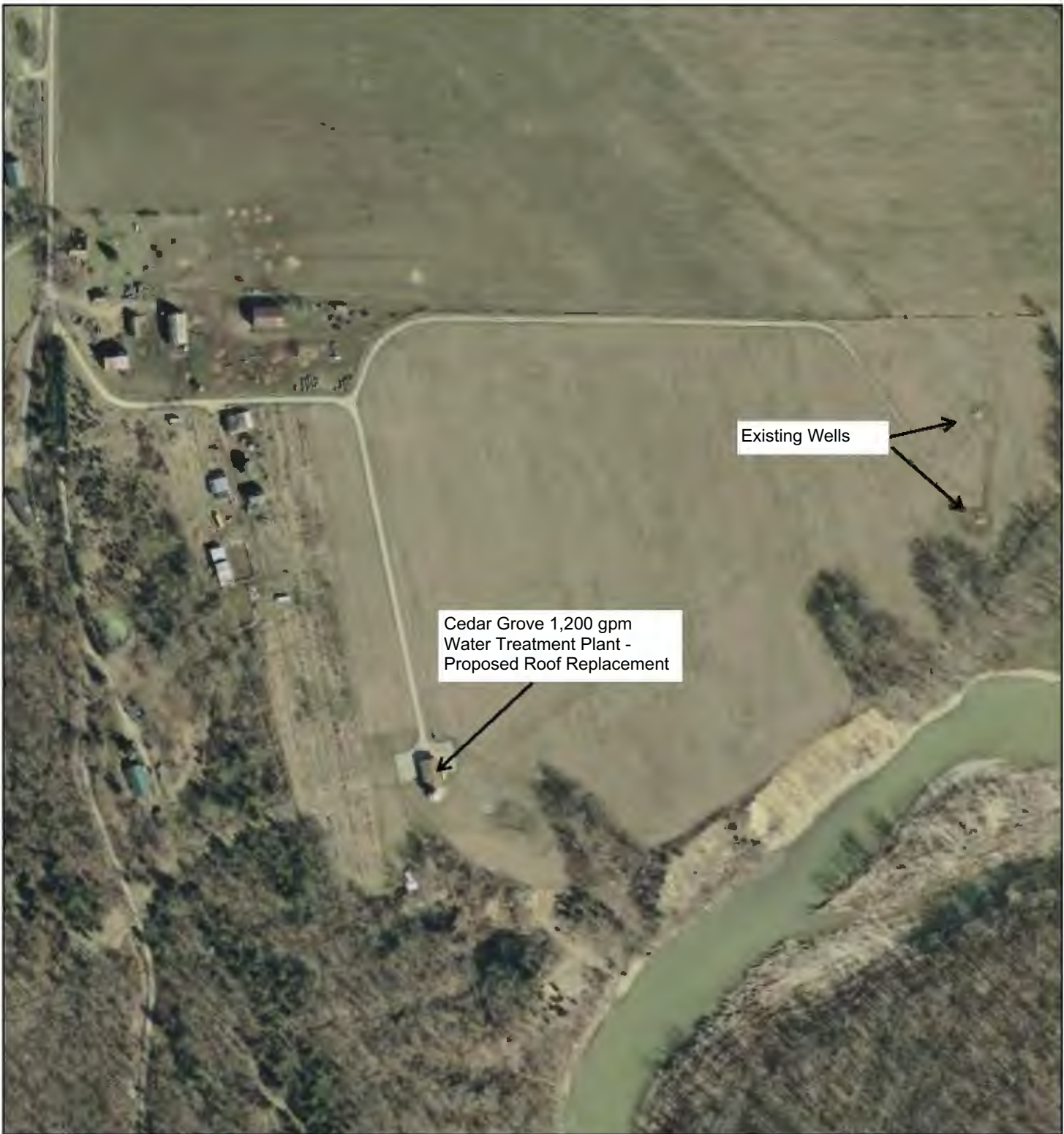
Figure 1.3.4 Tri-Township Water Corporation Proposed Cedar Grove Water Treatment Plant Roof Replacement Historic Sites Map
