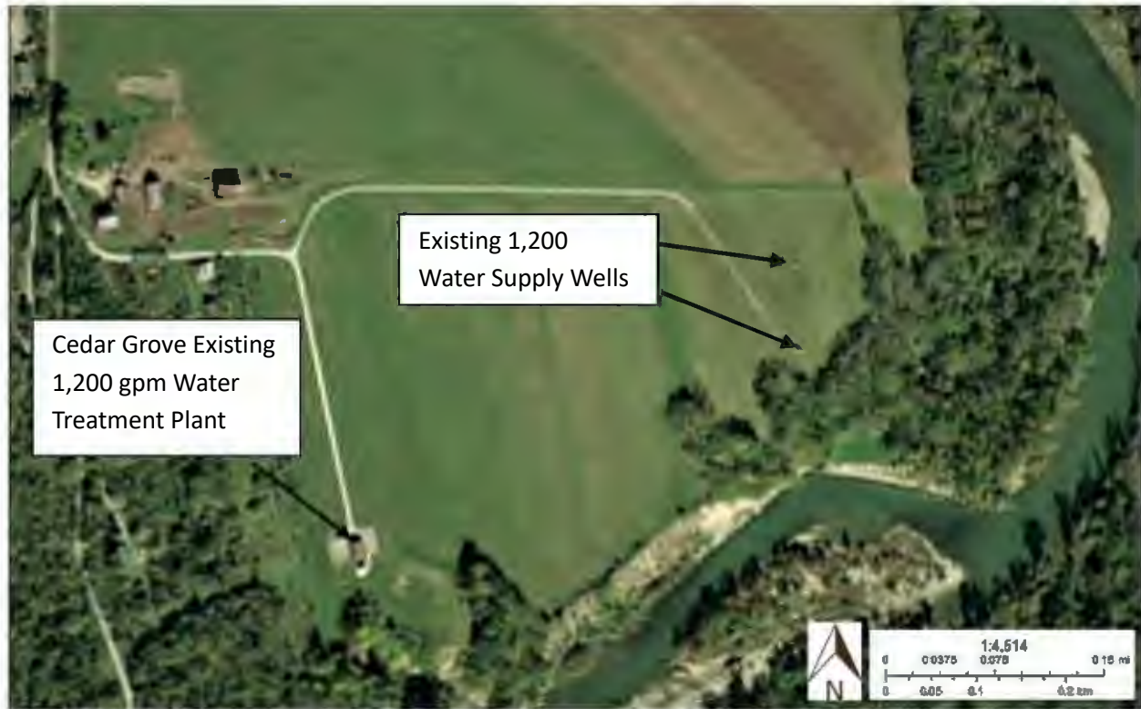
Figure 2.4.1 Existing Cedar Grove Well Field & Water Treatment Plant
