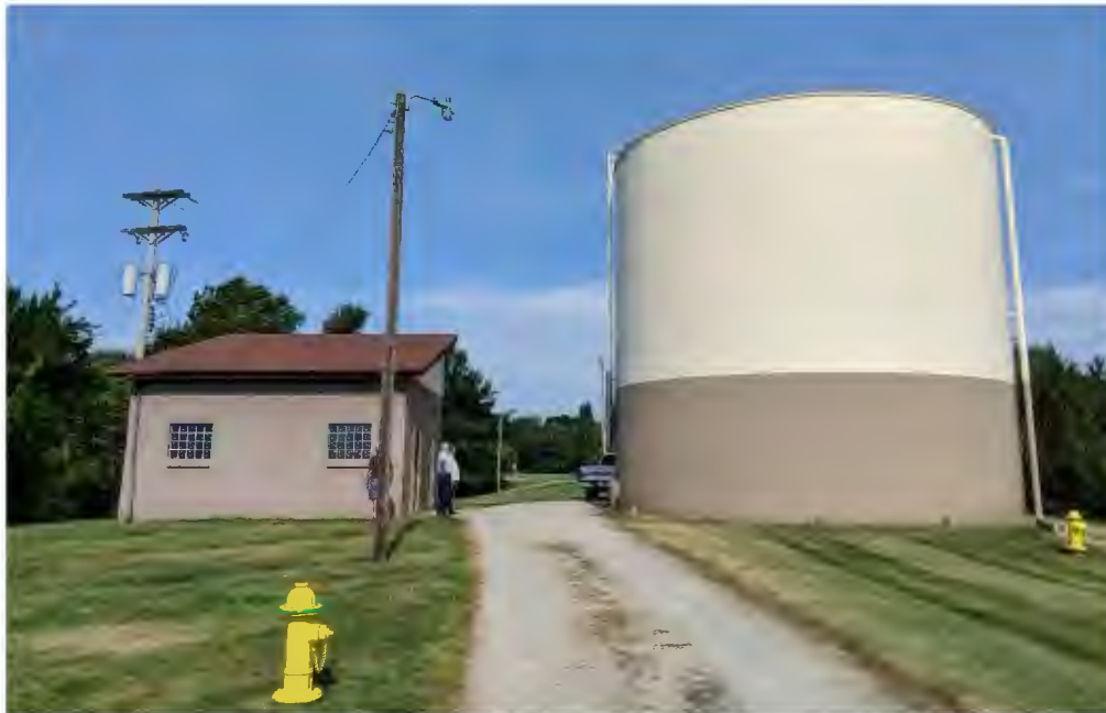
Morgan Road Booster Station, tank
