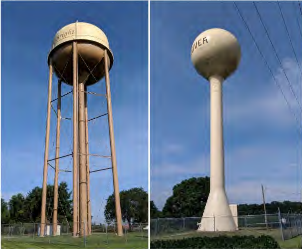
Justis Road (L) and Dover (R) tanks
