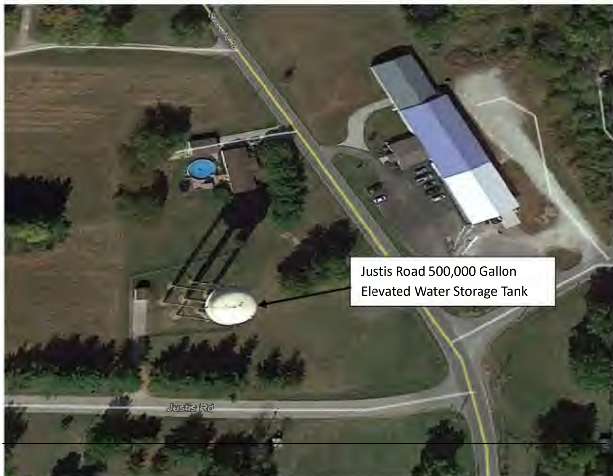
Figure 2.8.4 Existing Justis Road 500,000 Gallon Elevated Water Storage Tank
