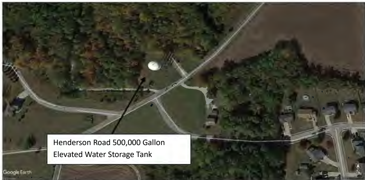
Figure 2.8.1 Existing Henderson Road 500,000 Gallon Elevated Water Tank
