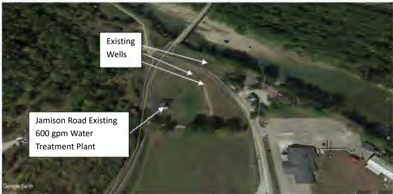
Figure 2.4.2 Jamison Road Well Field & Water Treatment Plant
