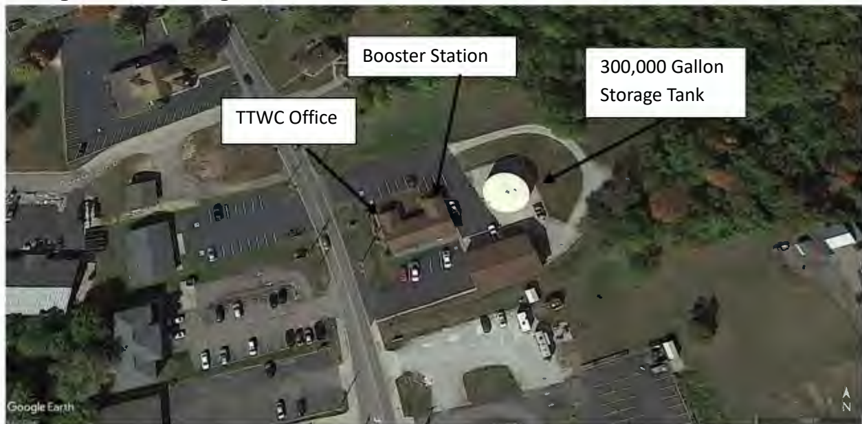
Figure 2.8.2 Existing TTWC Office, Booster Station, 300,000 Gallon Ground Level Tank
