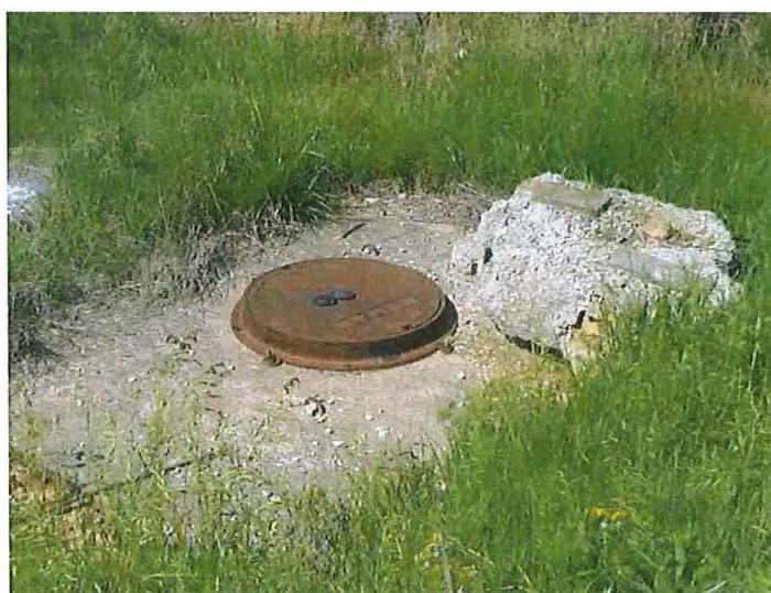
Point of connection (meter pit) with Evansville
