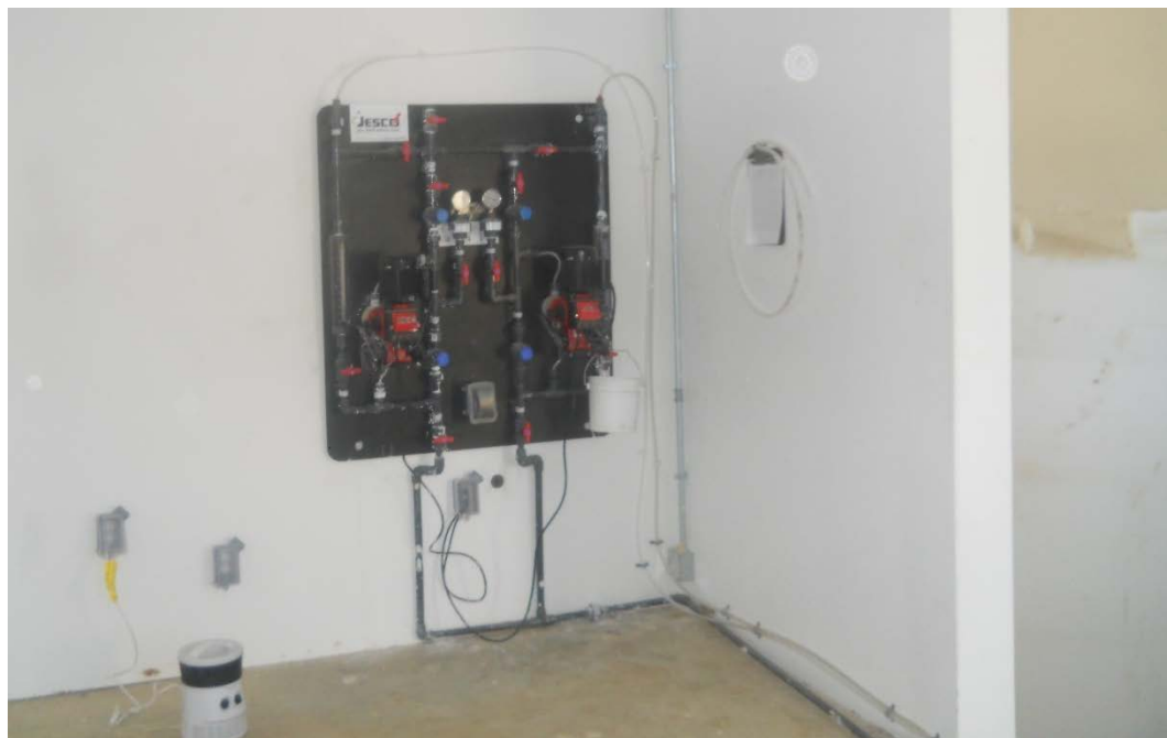
Figure 12 Phosphorus metering pump installation – December 4, 2019
