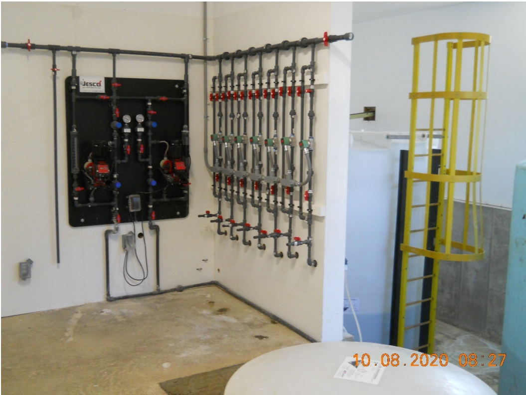
Figure 14 Phosphorus metering pump and piping installation – October 8, 2020
