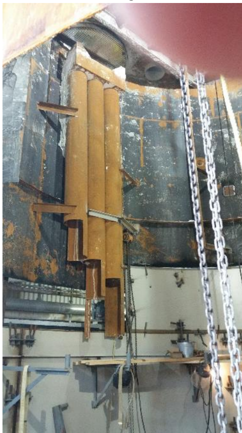
Photo 38 – Unit 2 Lime Mixing Tank - Foundation Rebuild
