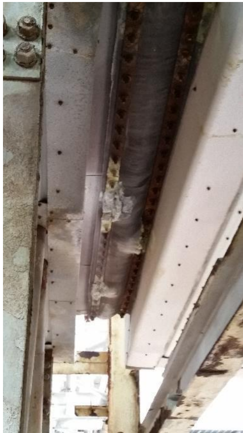
Photo 6 – Unit 1 North Absorber - Expansion Joint in Ductwork
