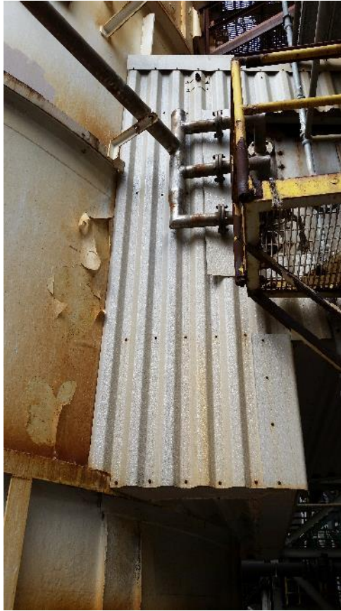
Photo 11 – Unit 1 South Absorber Tower Coating
