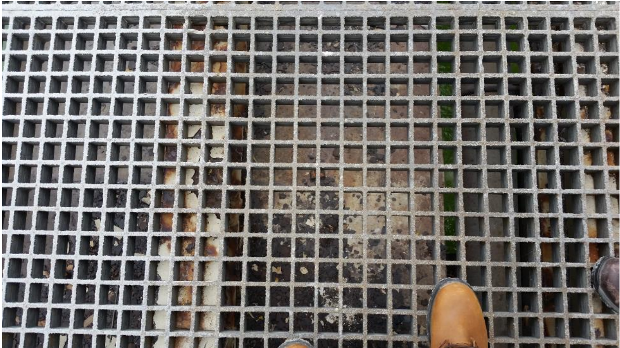
Photo 28 – Unit 1 Thickener - Grating Support Steel
