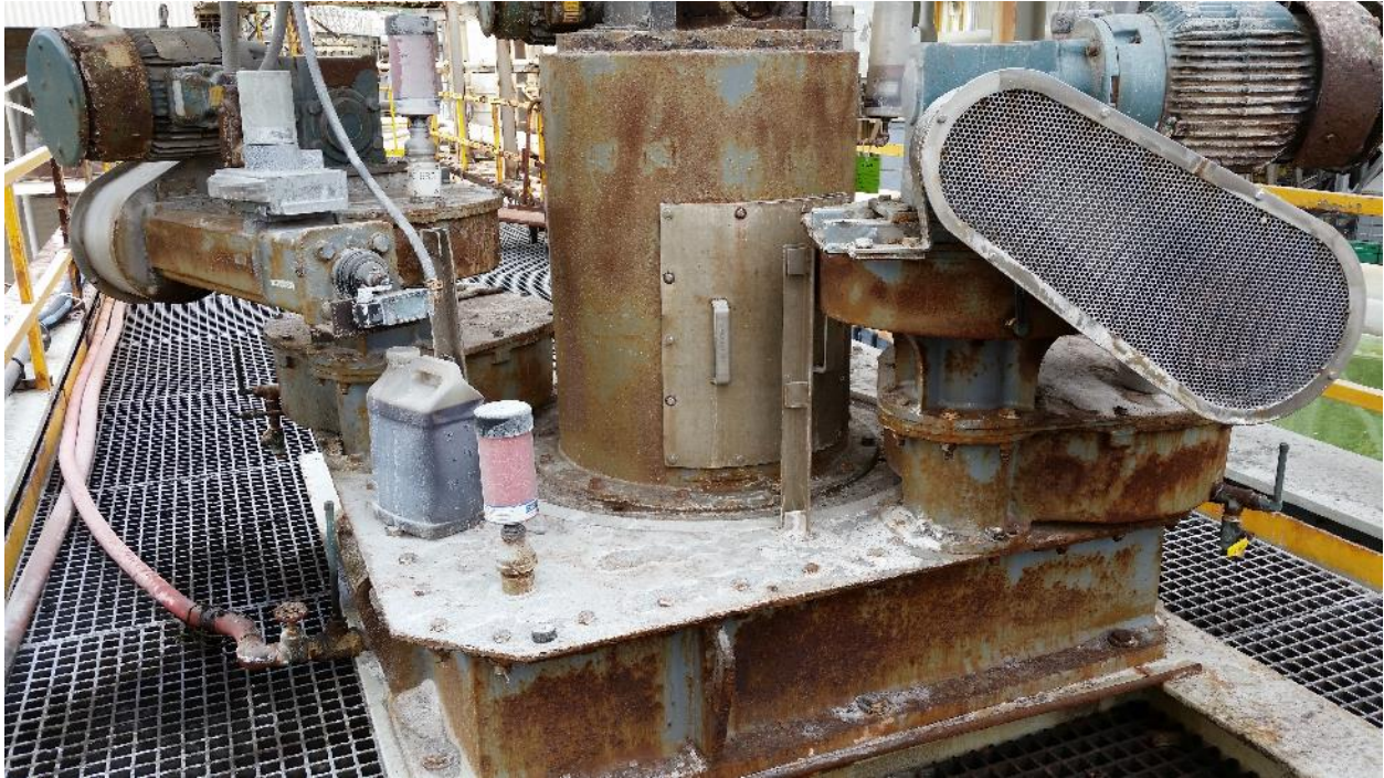
Photo 33 – Unit 1 Thickener - Drive
