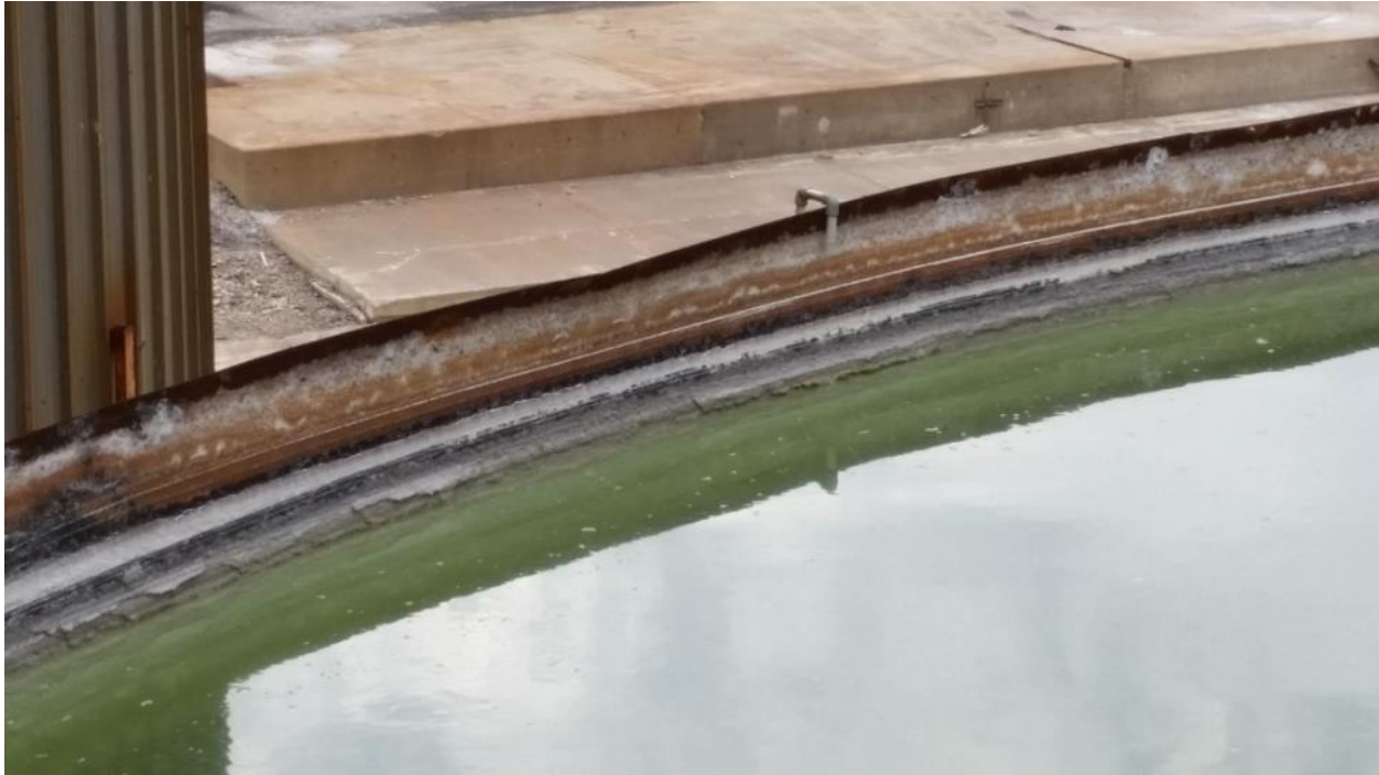
Photo 31 – Unit 1 Thickener - Launder Close-up
