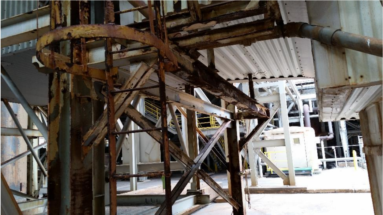
Photo 5 – Unit 1 North Absorber Outlet Duct Supports
