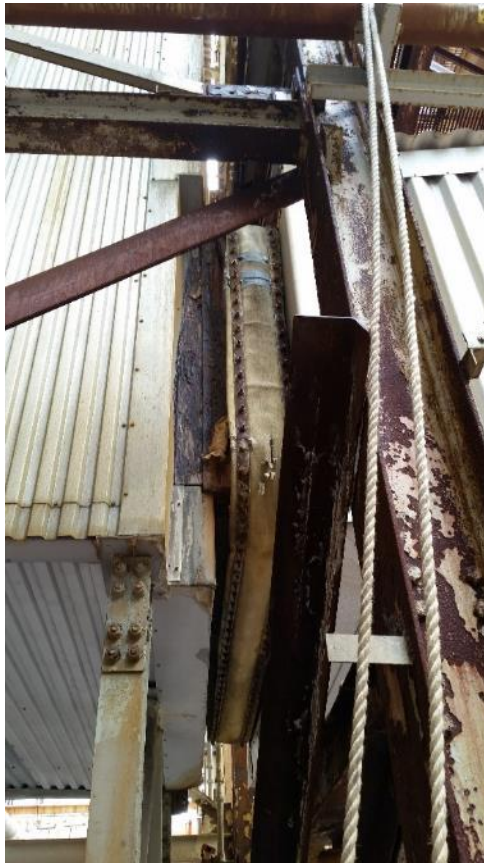
Photo 12 – Unit 1 South Absorber - Expansion Joint in Inlet Duct
