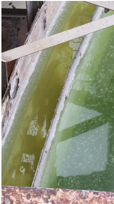
Photo 32 – Unit 1 Thickener - Launder Close-up Showing Color Difference
