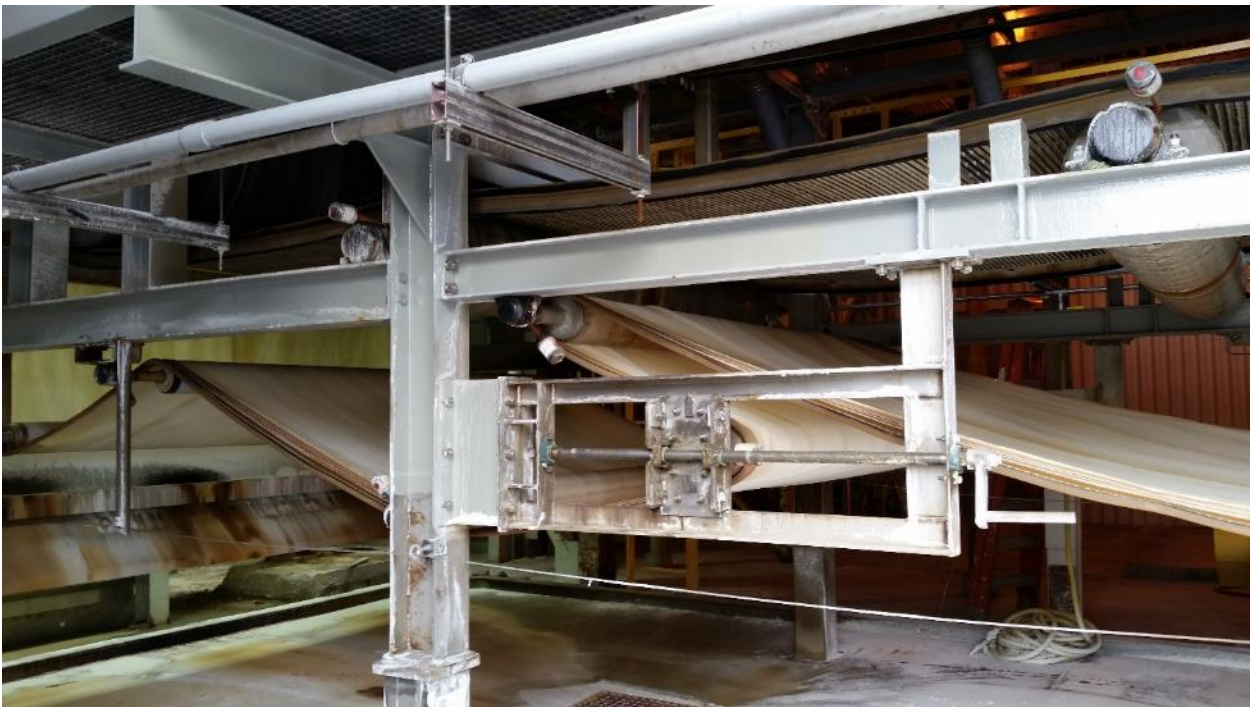
Photo 24 - Unit 1 Belt Filter Building - Belt Tightener
