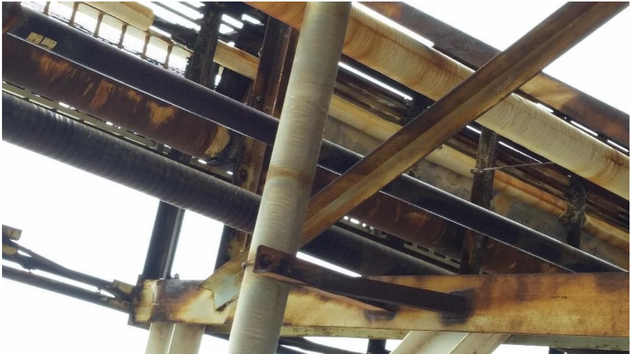
Photo 19 – Unit 1 South Absorber - Close-up of Pipe Supports
