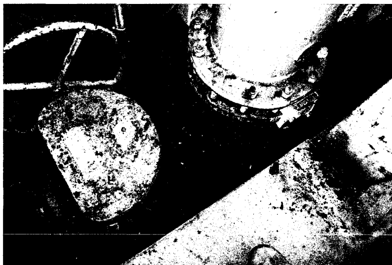
FIGURE 3-19 Corrosion in Pipe Gallery for North Filters 29-32
