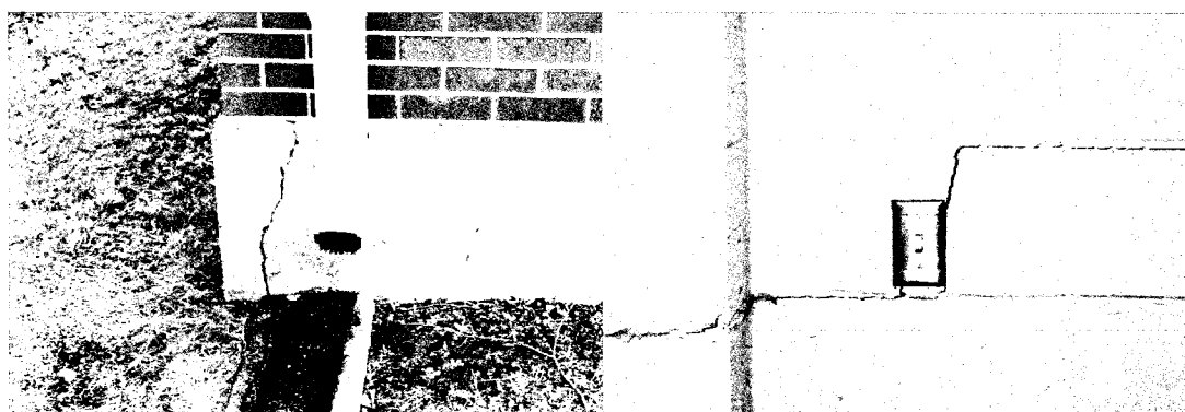
FIGURE 2-12 Killian Booster Station Structure Cracks
