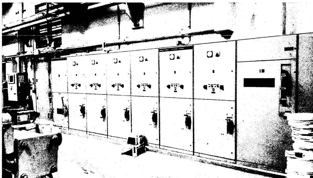
FIGURE 3-42 WTP Switchgear (MVC)
