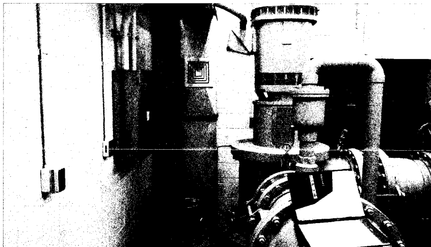
FIGURE 2-21 Weinbach Booster Station Code Violation
