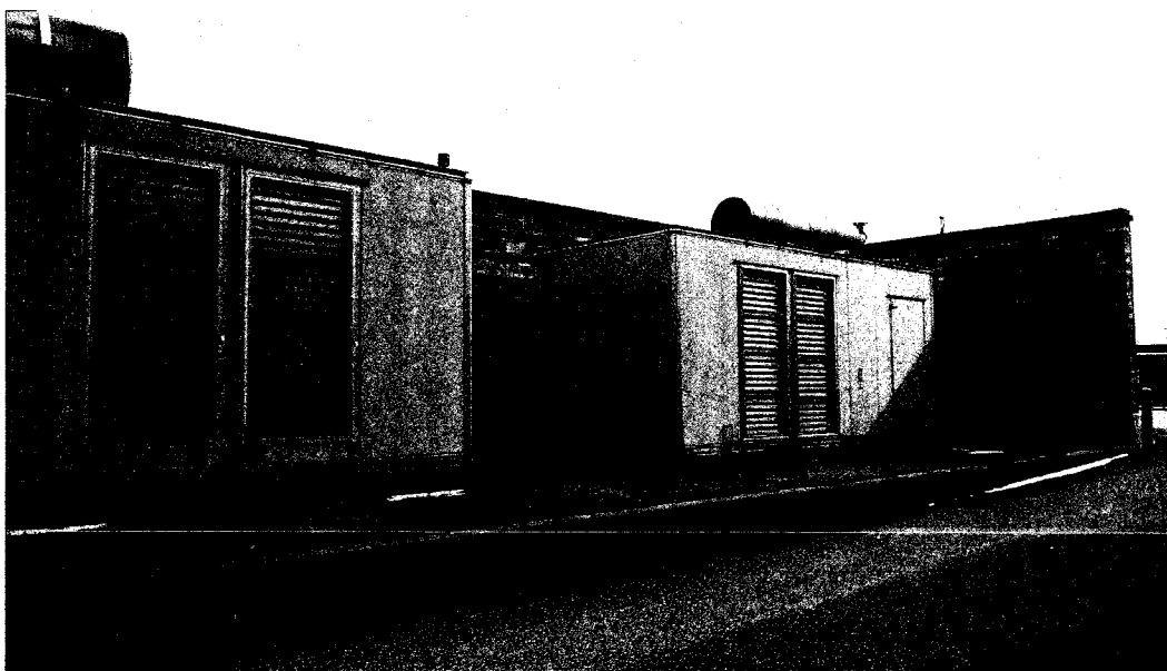
FIGURE 3-39 Back-Up Diesel Generators
