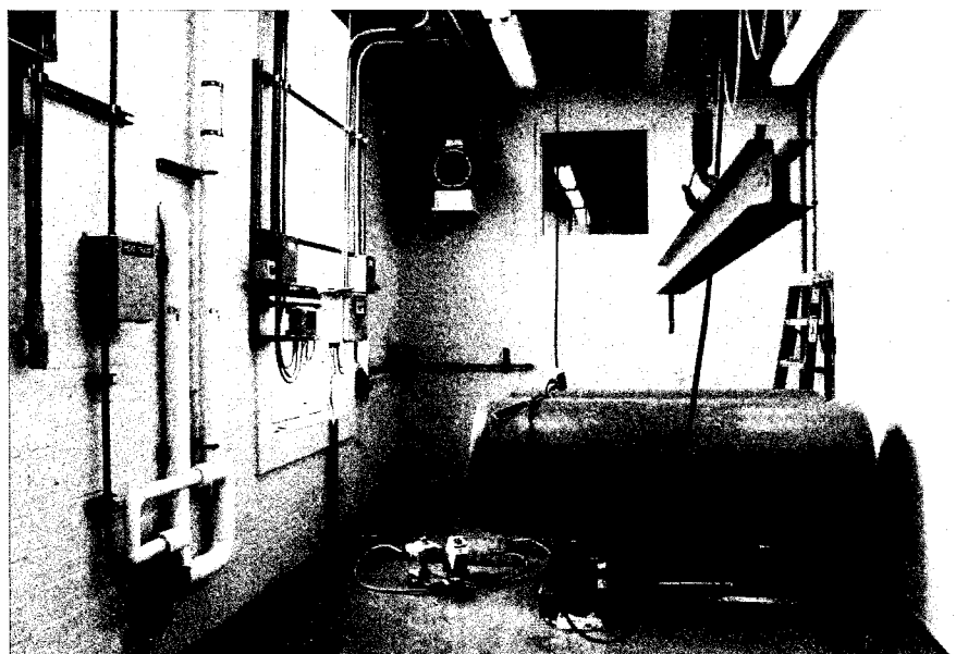
FIGURE 3-25 Sulfur Dioxide Chemical Feed System for Backwash Disinfection
