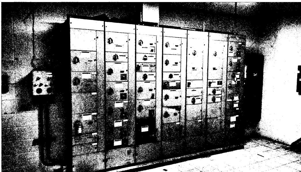
FIGURE 3-45 South Filter Building Electrical Room MCC
