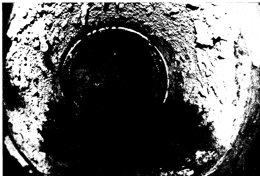
FIGURE 3-32 Interior of Effluent Piping from High Service Pump Station No. 2
