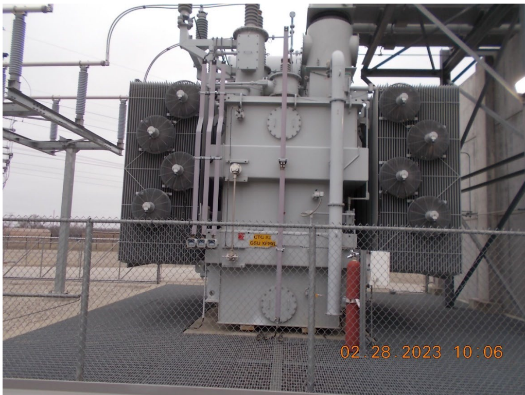
ACCOUNT 345, ACCESSORY ELECTRIC EQUIPMENT GT UNIT 2 GSU TRANSFORMER
