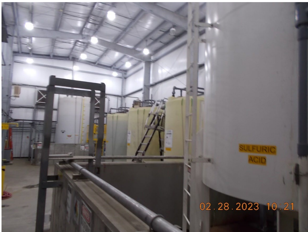
ACCOUNT 343, PRIME MOVERS CHEMICAL STORAGE FOR WATER TREATMENT
