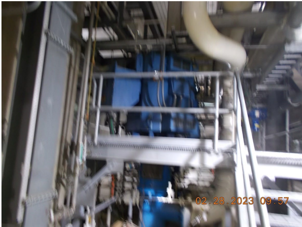
ACCOUNT 312, BOILER PLANT EQUIPMENT CONDENSATE PUMP
