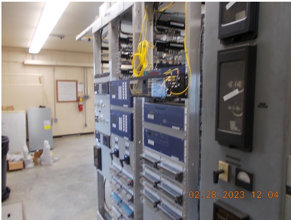
ACCOUNT 362, STATION EQUIPMENT MICROPROCESSOR CONTROLS
