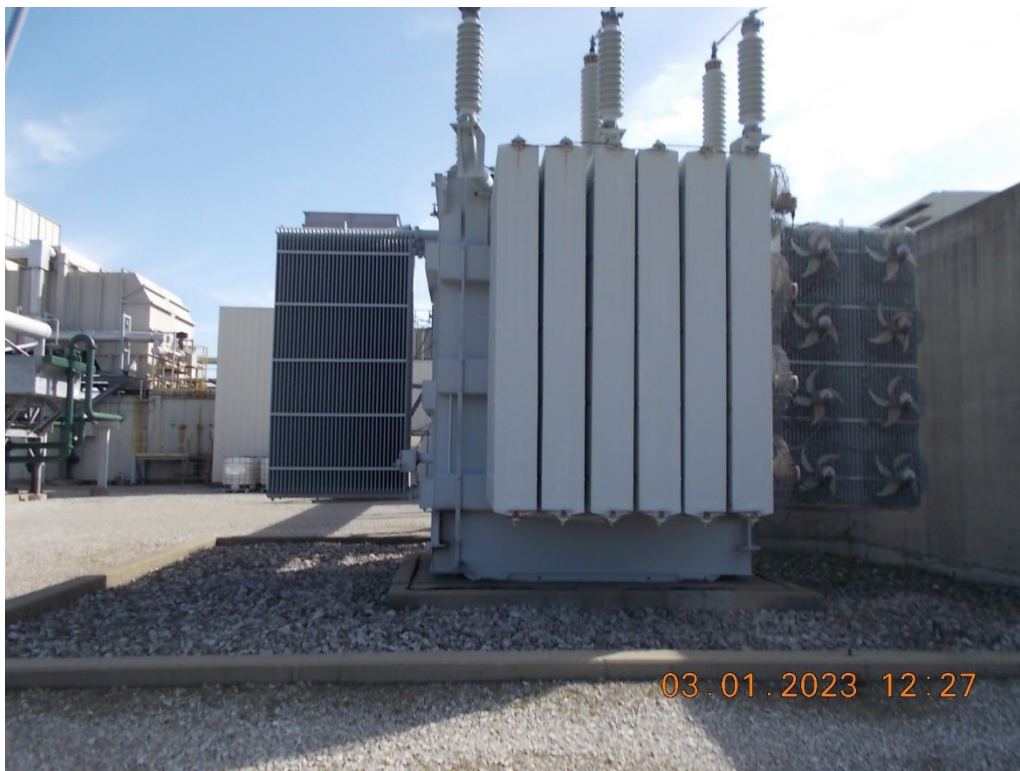
ACCOUNT 345, ACCESSORY ELECTRIC EQUIPMENT GT UNIT 1 GSU
