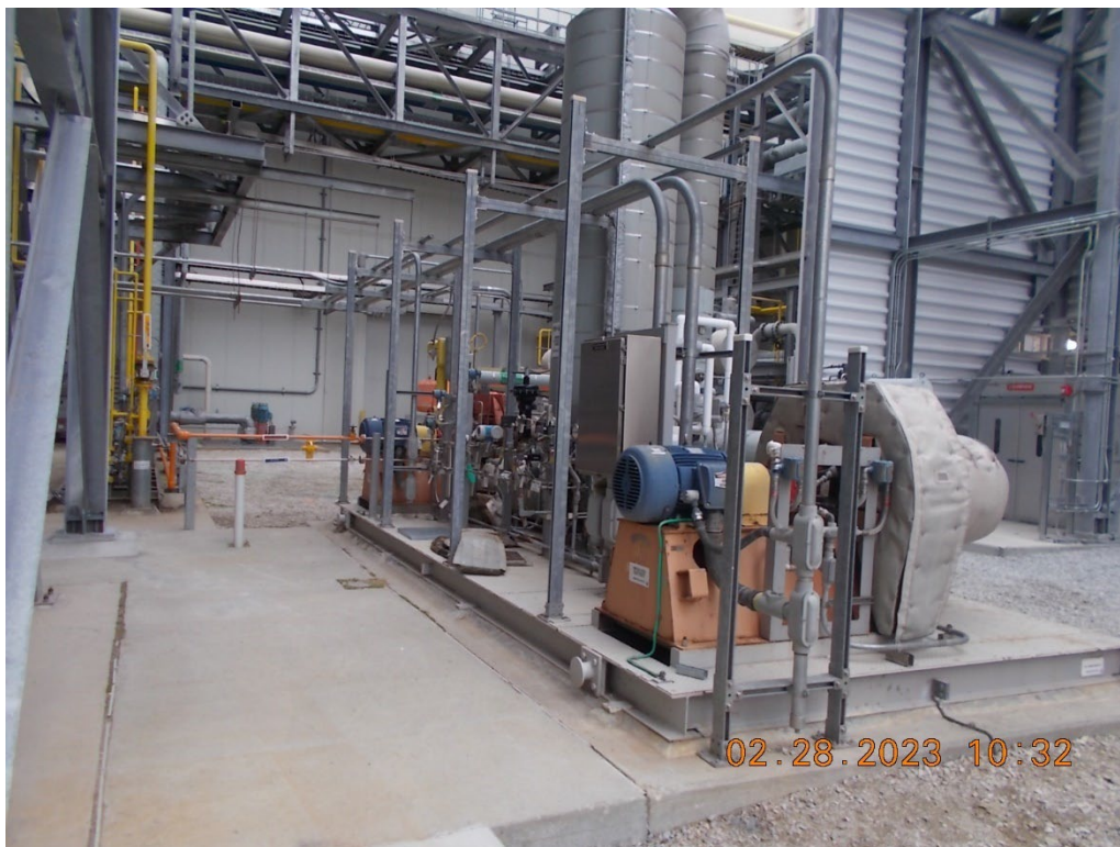
ACCOUNT 344, GENERATORS AMMONIA VAPORIZOR SKID
