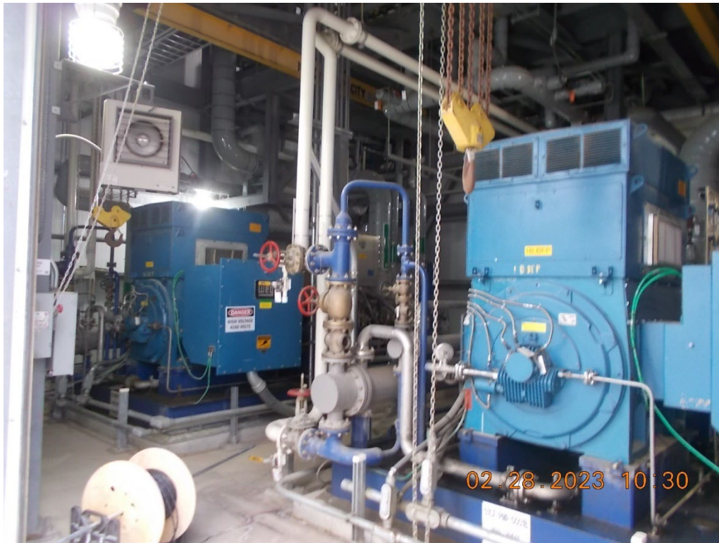
ACCOUNT 312, BOILER PLANT EQUIPMENT BOILER FEED PUMPS
