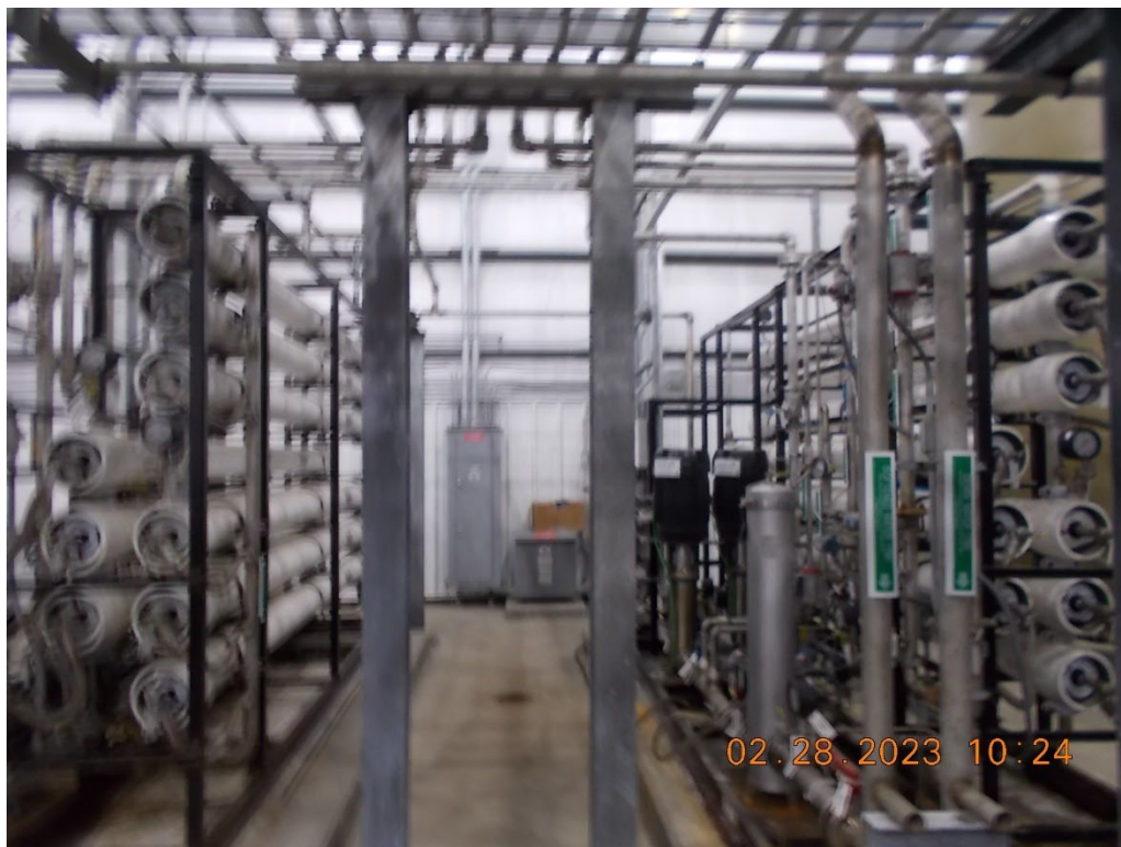
ACCOUNT 343, PRIME MOVERS RO WATER TREATMENT SYSTEM
