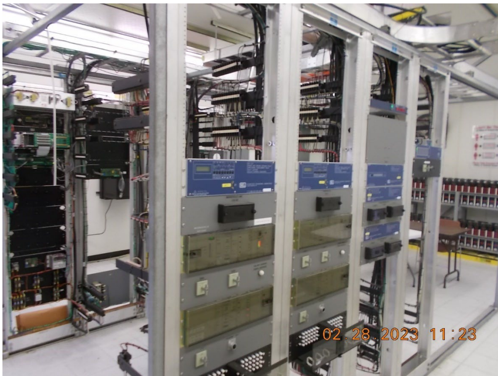
ACCOUNT 362, STATION EQUIPMENT MICROPROCESSOR CONTROLS
