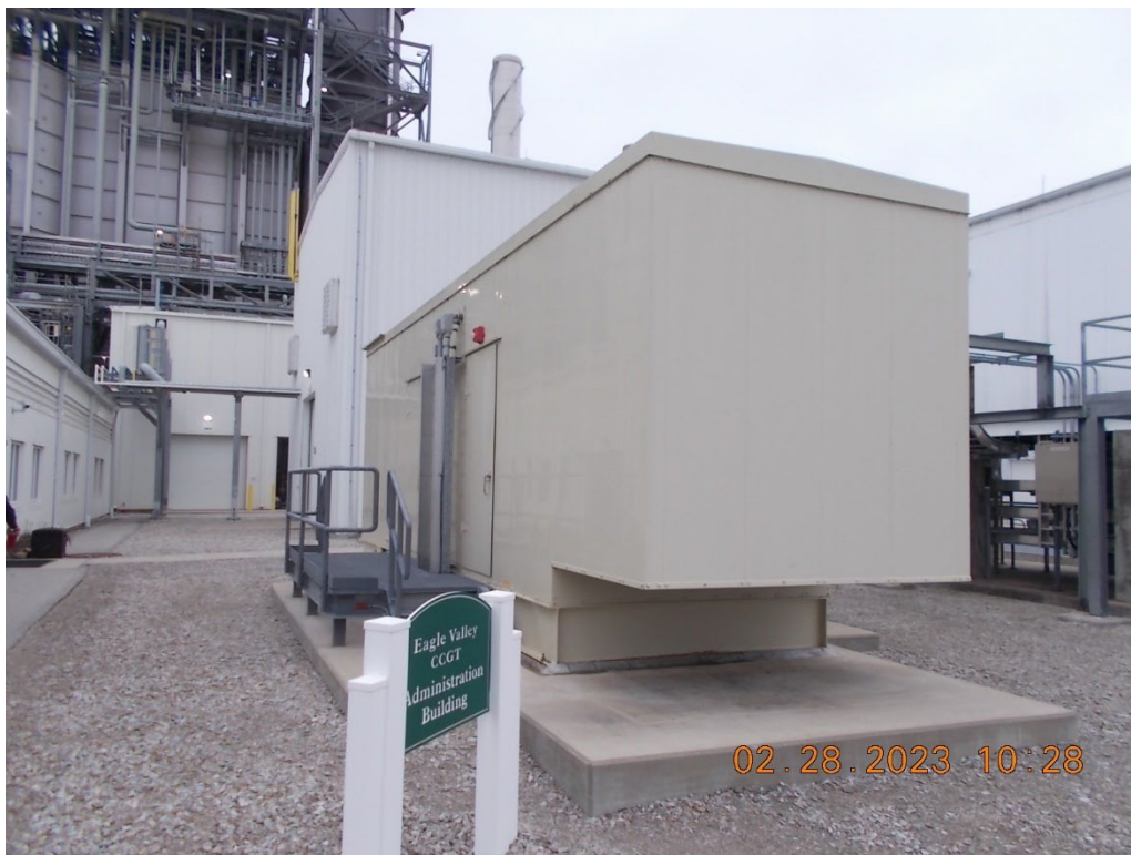
ACCOUNT 344, GENERATORS BACKUP DIESEL GENERATOR
