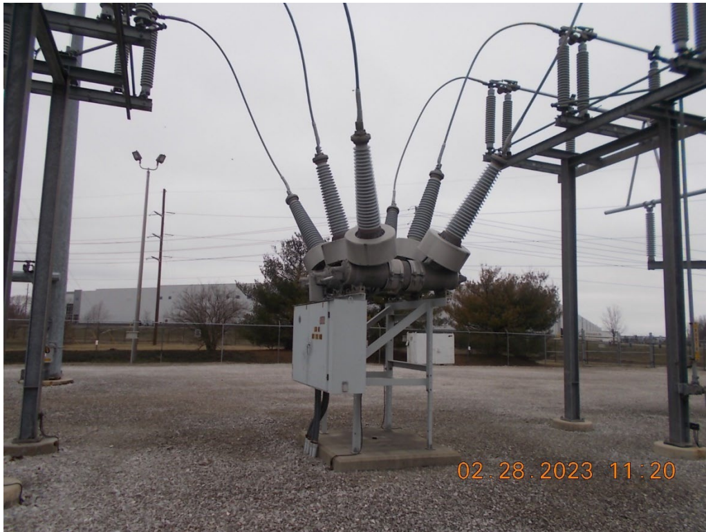
ACCOUNT 362, STATION EQUIPMENT SF6 GAS BREAKER
