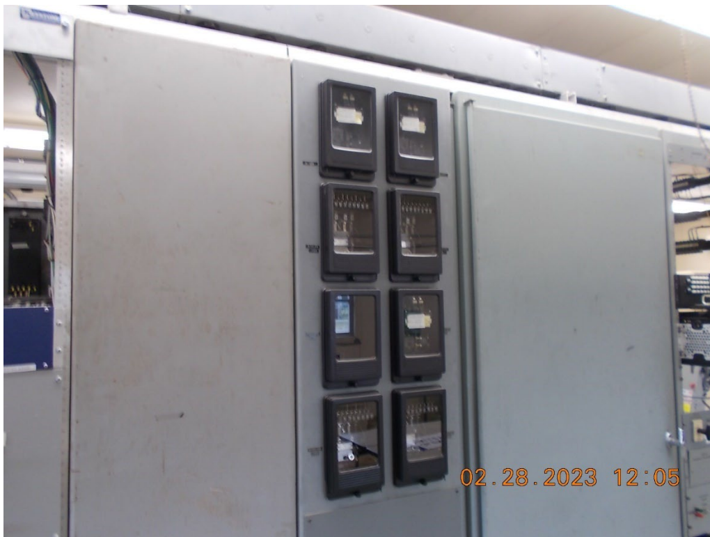
ACCOUNT 362, STATION EQUIPMENT ELECTROMECHANICAL RELAYS
