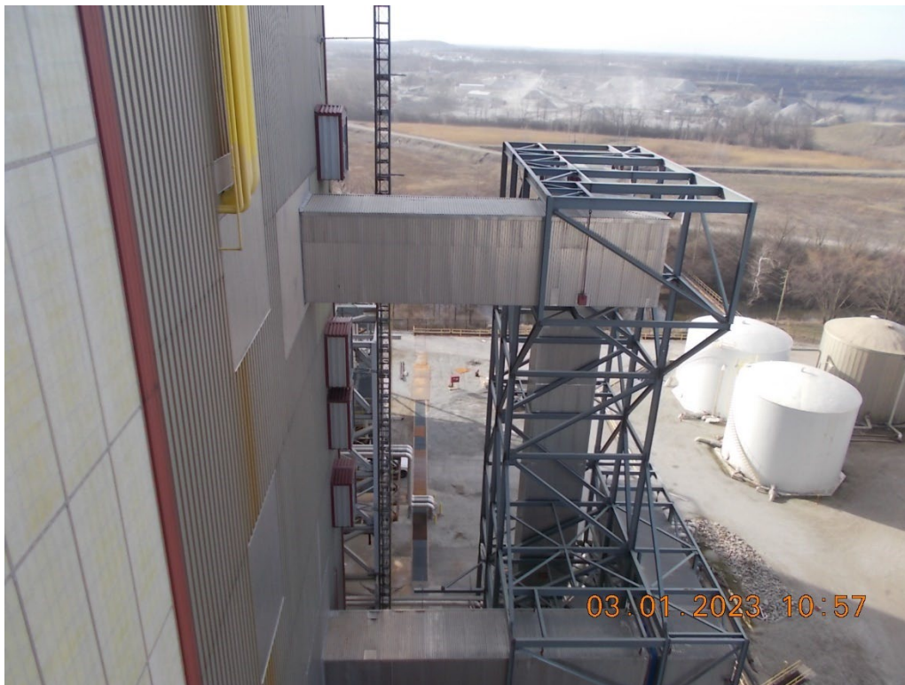
ACCOUNT 312, BOILER PLANT EQUIPMENT STEAM UNIT 7 FDR DUCTWORK FOR COOLING FANS
