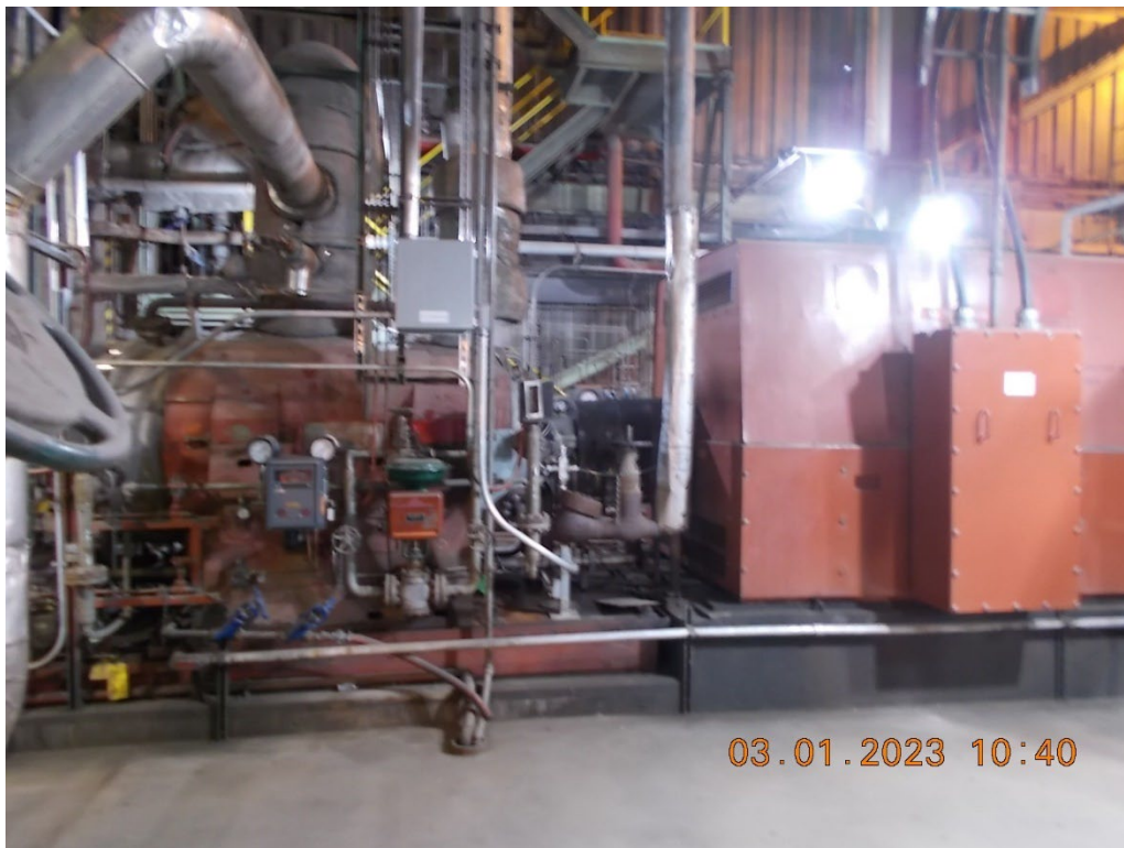
ACCOUNT 312, BOILER PLANT EQUIPMENT BOILER FEED PUMP
