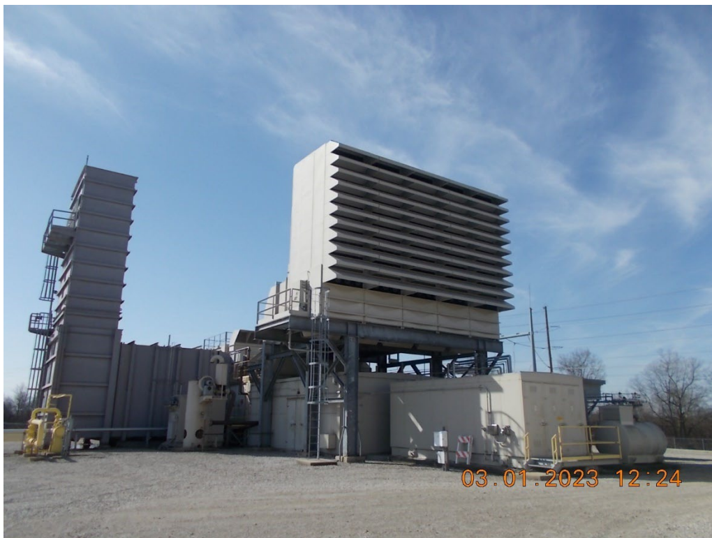
ACCOUNT 344, GENERATORS GT UNIT 4 AIR INTAKE
