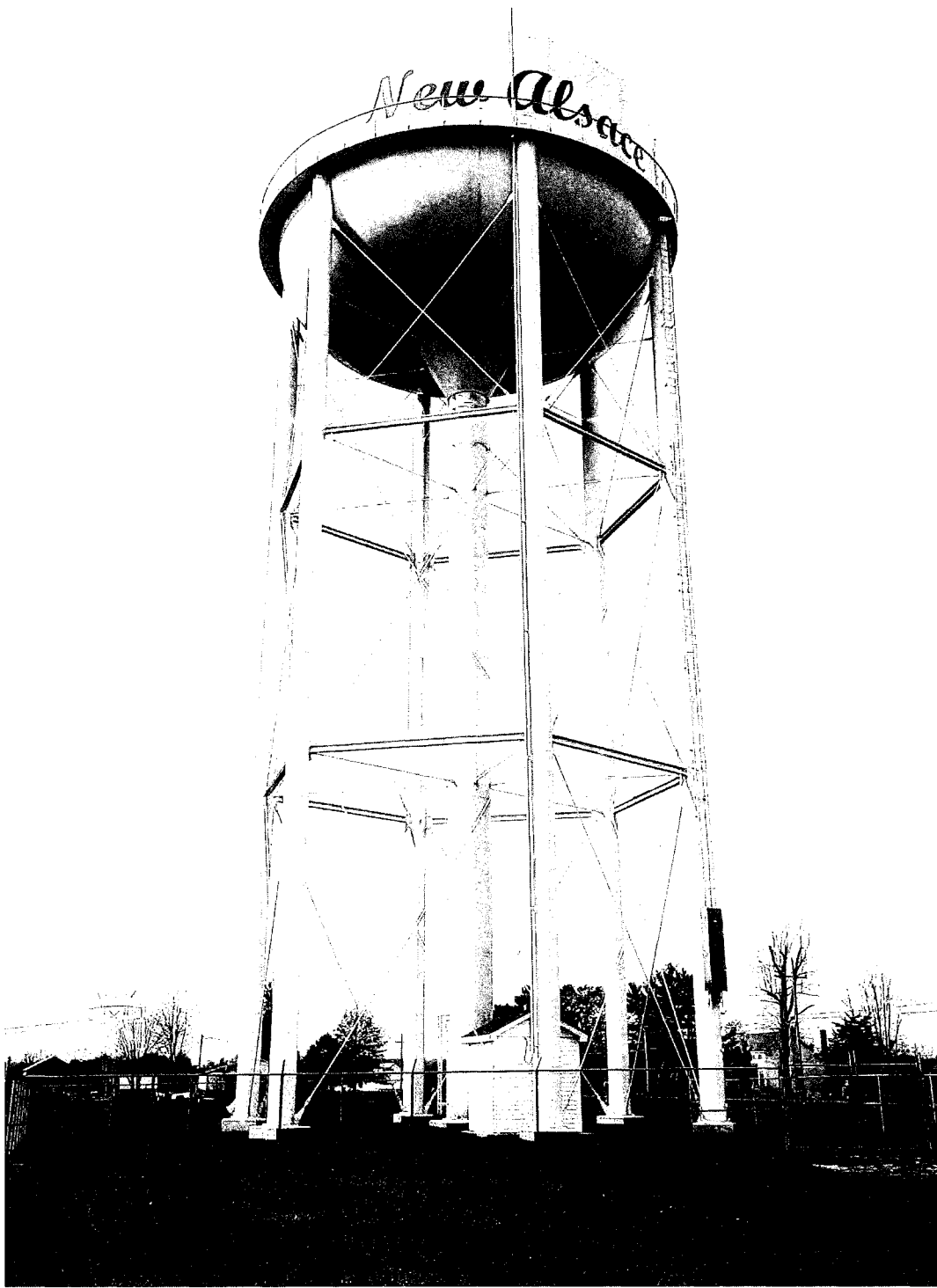
New New Alsace 500,000-gallon Tank
