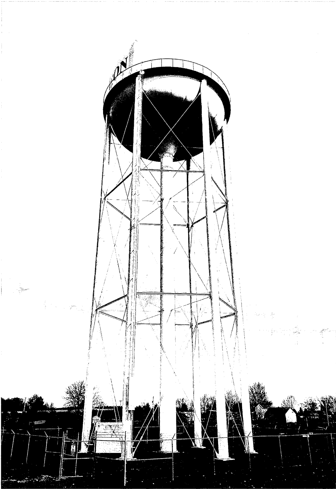
St. Leon 500,000-gallon tank
