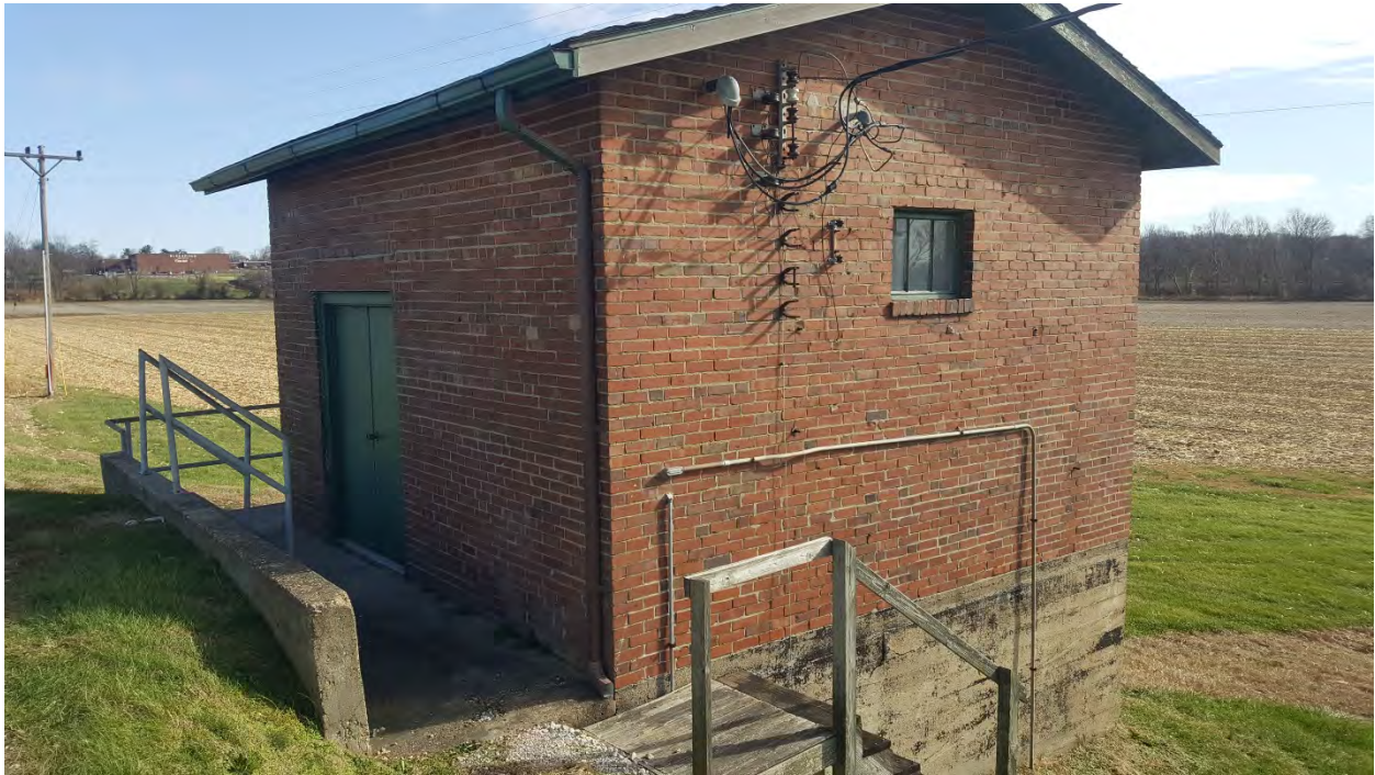
Bloomfield Wellfield Treatment Plant Exterior
