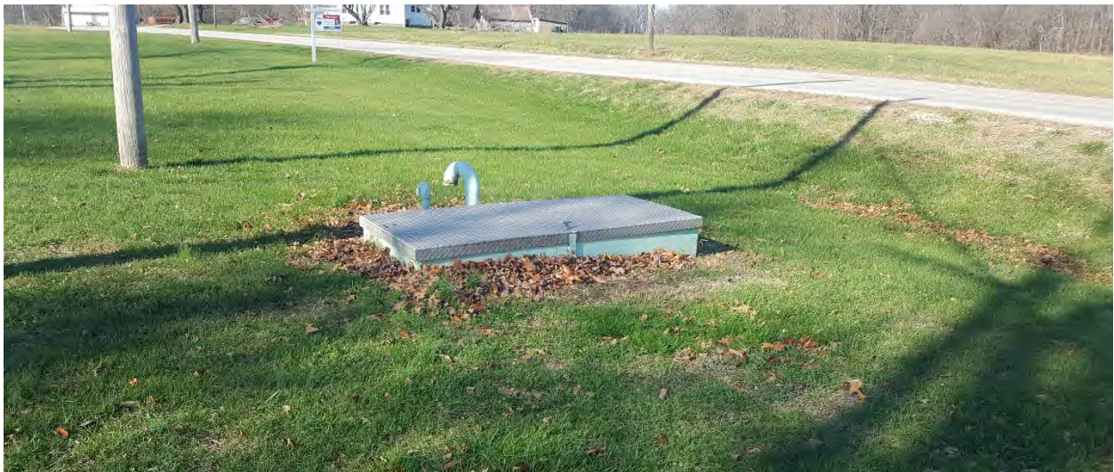
Booster Station #2 Exterior
