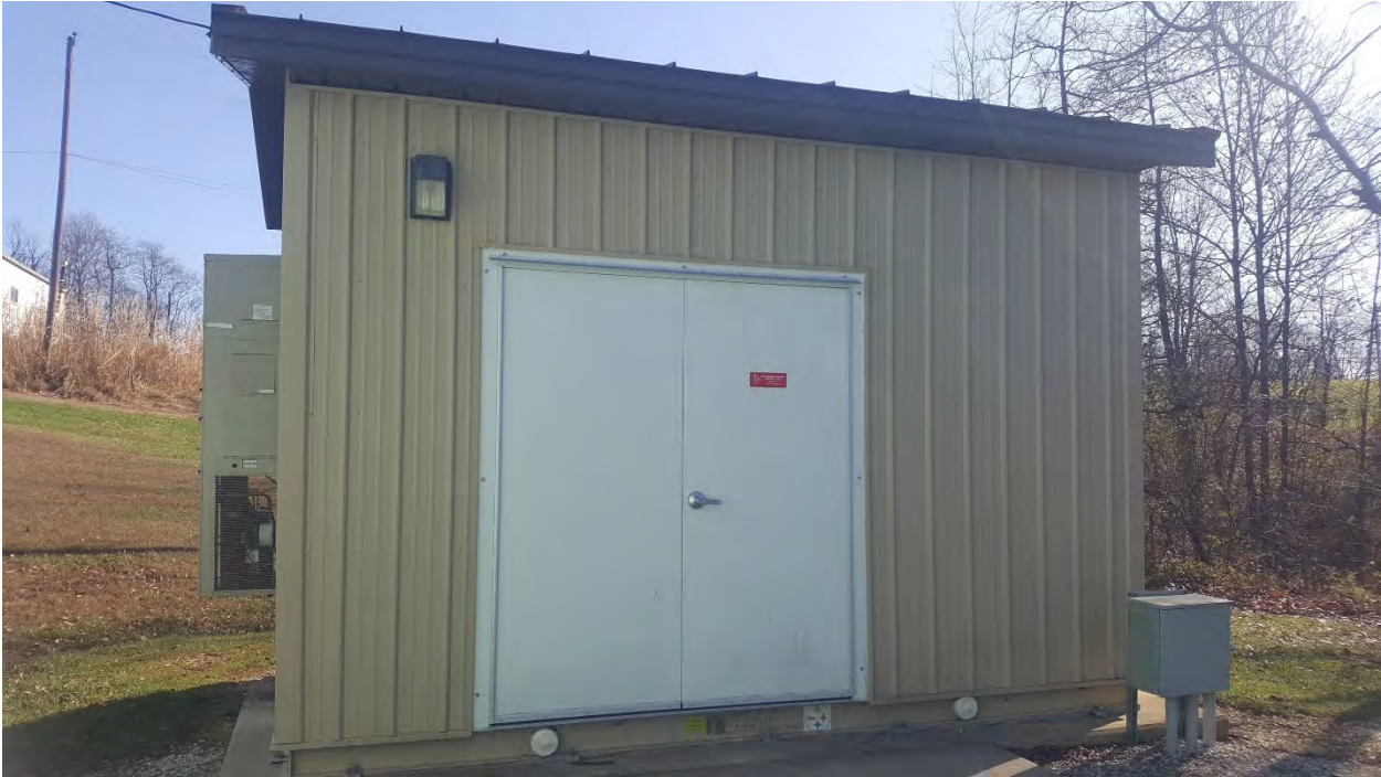
Booster Station #1 Exterior
