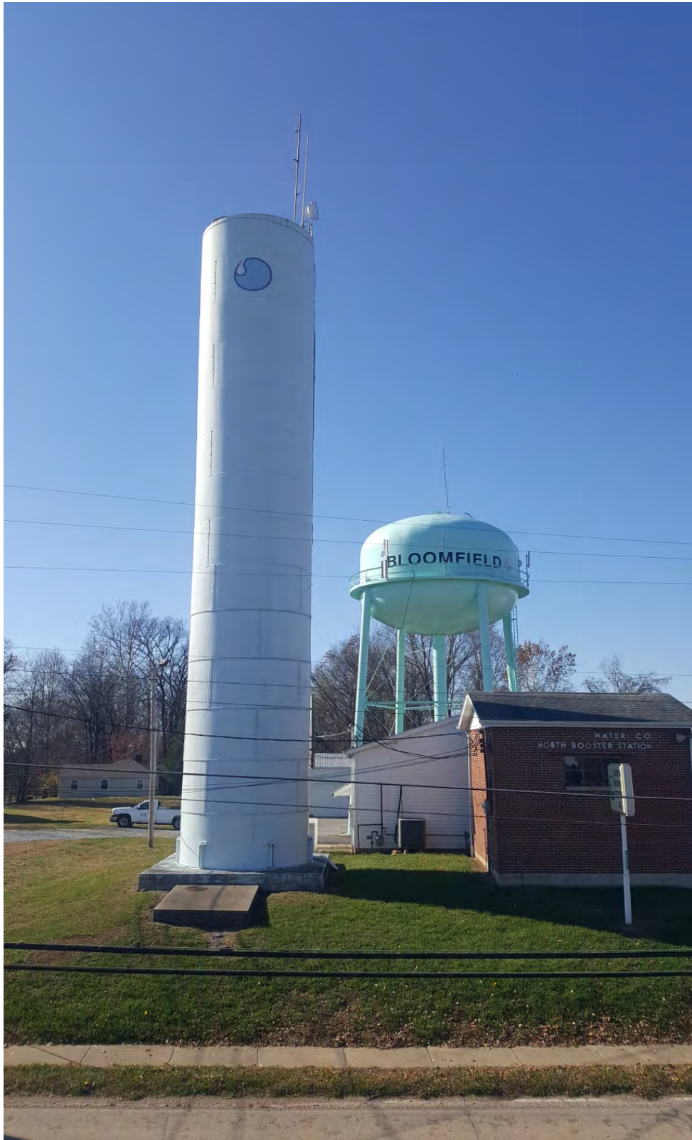
Bloomfield Standpipe – 60,000 gal. & Bloomfield Storage Tank – 200,000 gal.
