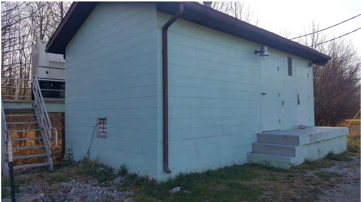
Worthington Wellfield Treatment Plant Exterior
