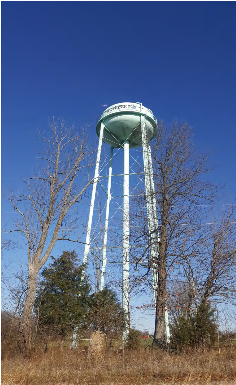
Sosberry Storage Tank – 100,000 gal.
