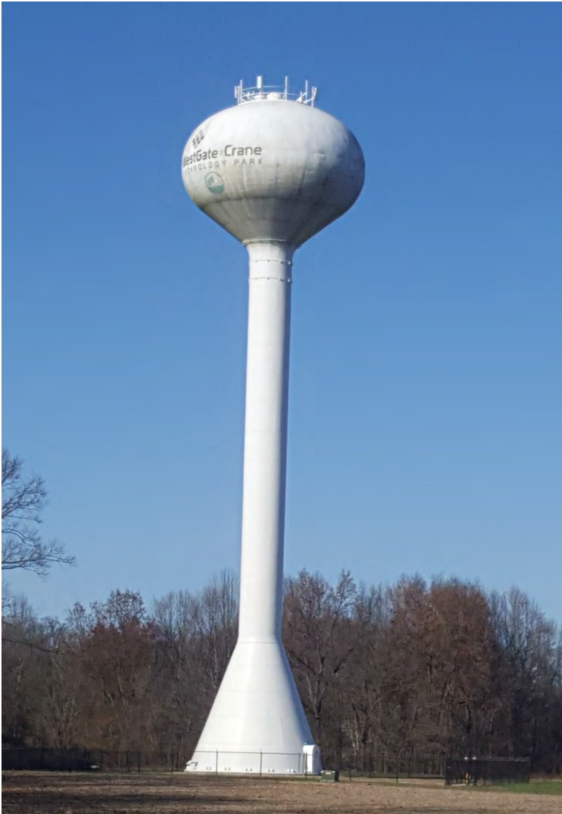
Westgate Storage Tank – 250,000 gal.
