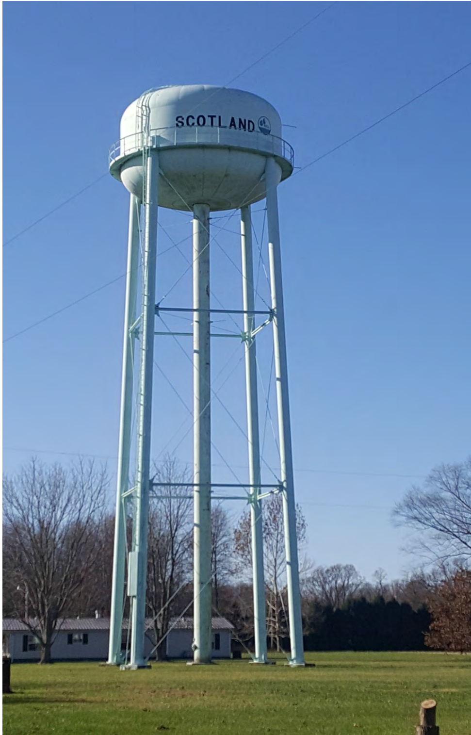
Scotland Storage Tank – 100,000 gal.
