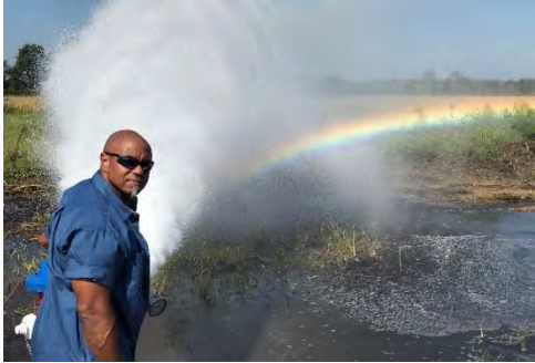
Dell Allen flushing new distribution line
