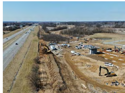
Water Main Installation – Beacon Pkwy
