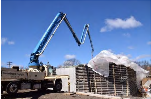
Pumping concrete to the top of the tank
