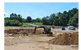
Live Webcam Gumwood Well Field 1.5 Million Gallon Water Storage Tank Build
