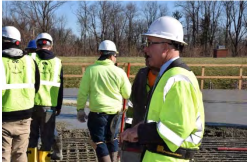
Mayor Dave helping out at the new tank
