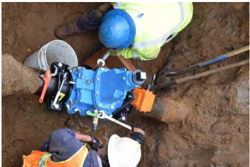
Valve insertion equipment installation
