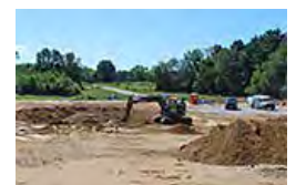
Live Webcam Gumwood Well Field 1.5 Million Gallon Water Storage Tank Build
