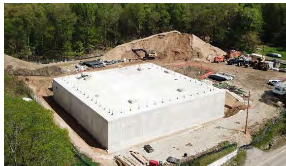
New 2-million-gallon water tank under construction
