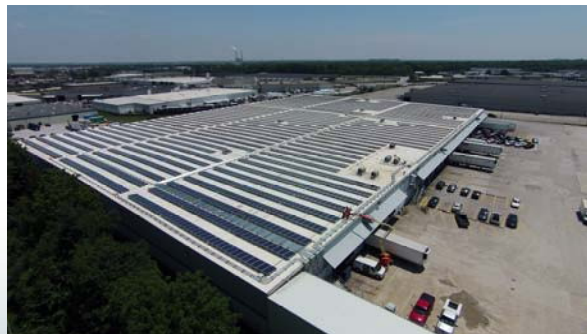
Grocers Supply Roof, 1MW rooftop system.
