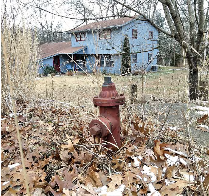
Typical flush hydrant (fire hydrants not provided)
