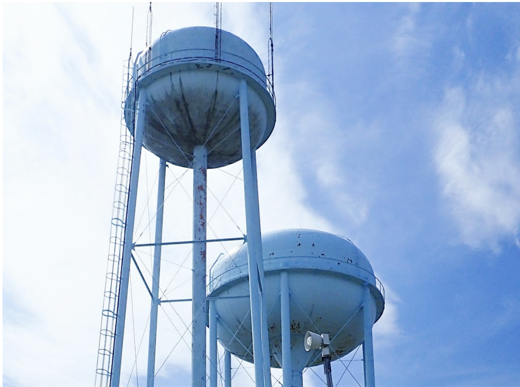
Wye Tanks in 2017 before coating
