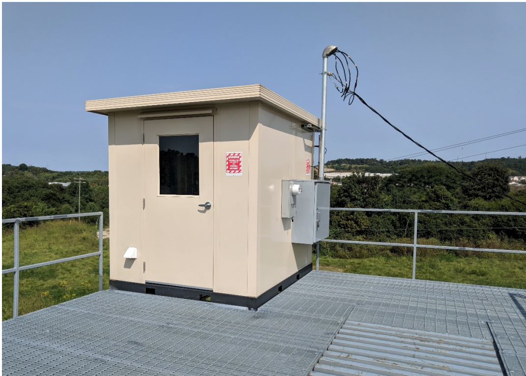
New well control building exterior
