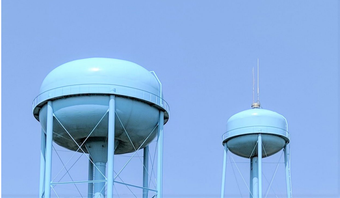
Wye Tanks close-up in September 2020 showing new coating
