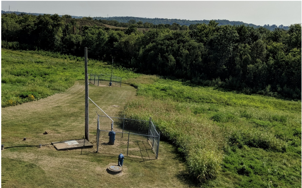
View of wellfield from new well control structure
