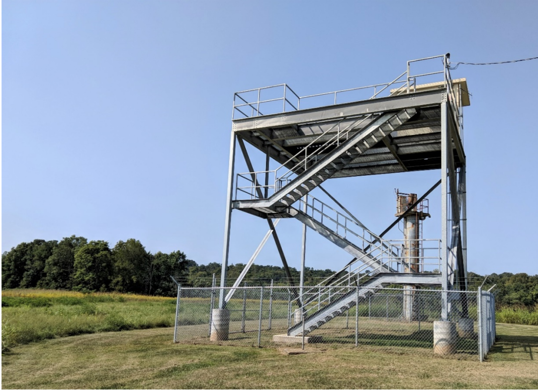
New well control platform, building in foreground, old platform in background
