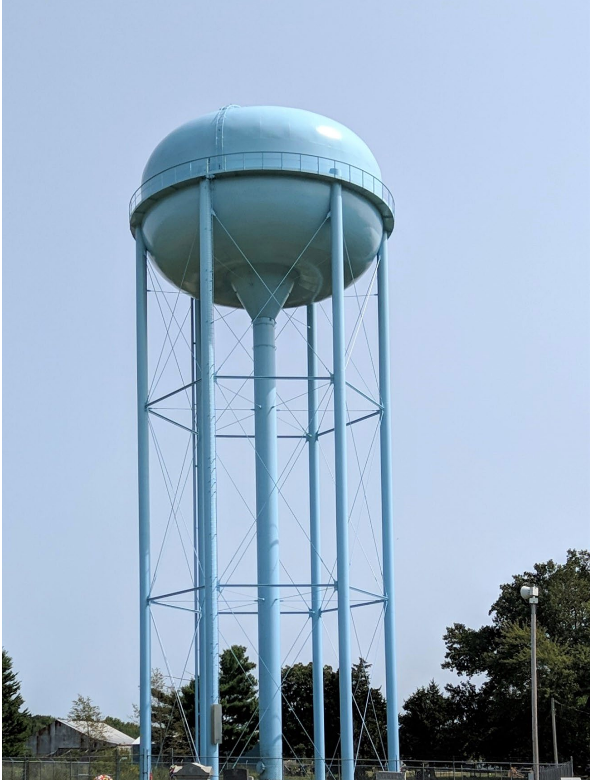
Hogan Hill tank September 2020 after coating
